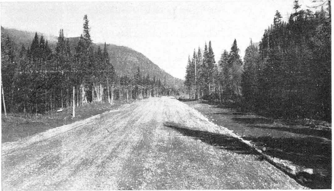
Gravel coating laid on the new St. Anne des Monts—New Richmond road.
