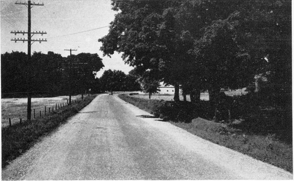
Surface treatment laid at Roxton Pond on Highway No. 13. This type of work was carried out, in 1950, over a length of 593 miles in various regions of the Province.
