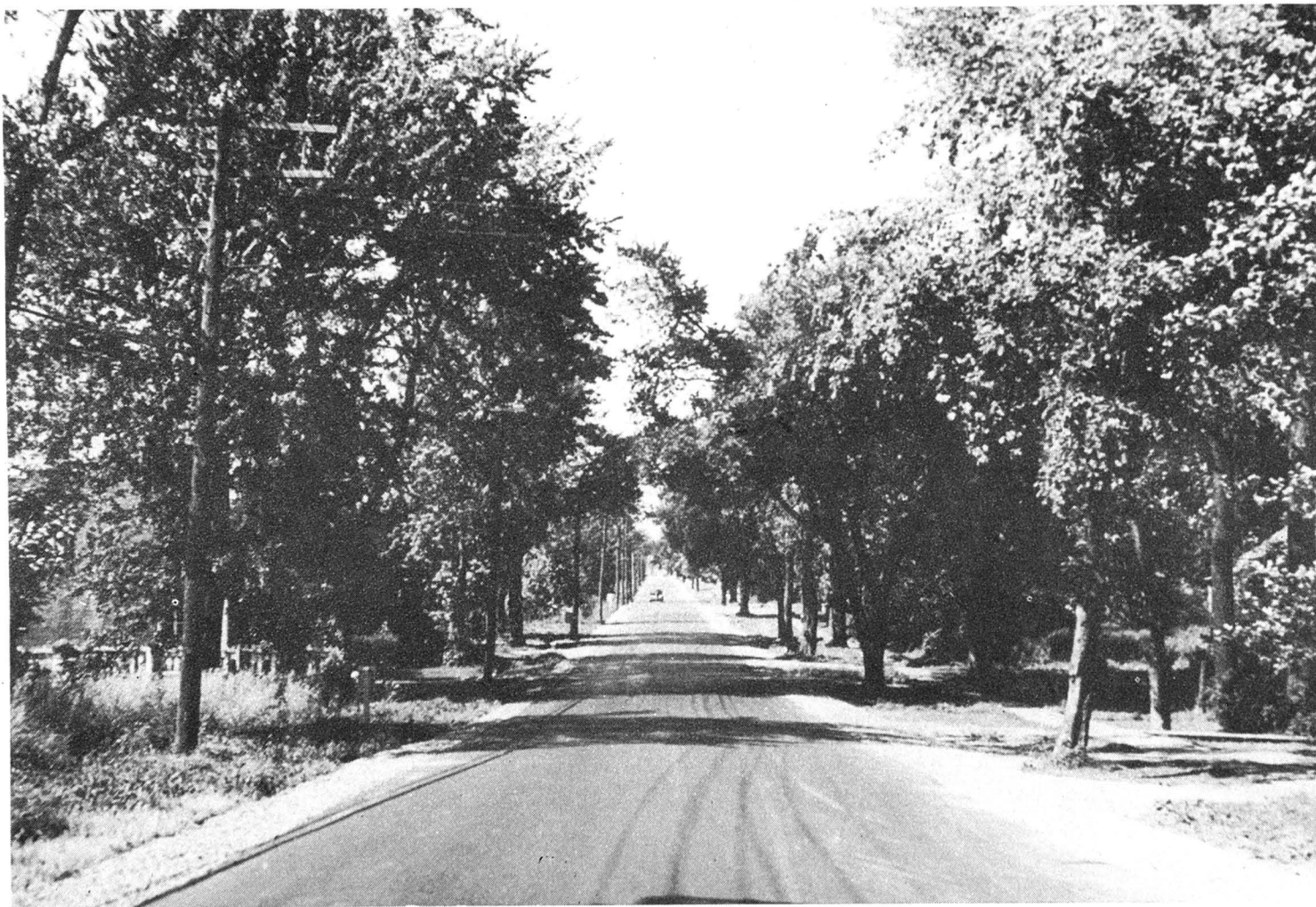
Asphalt carpet coat laid in 1945, on the connecting road of Highways 2 and 37, at Dorval.
