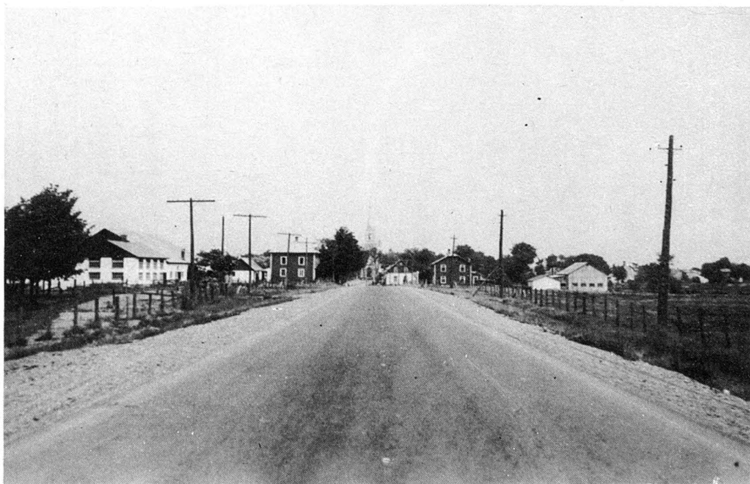
Same section of Highway No.23, near Saint-Henri, after the laying of the bituminous concreté pavement.
