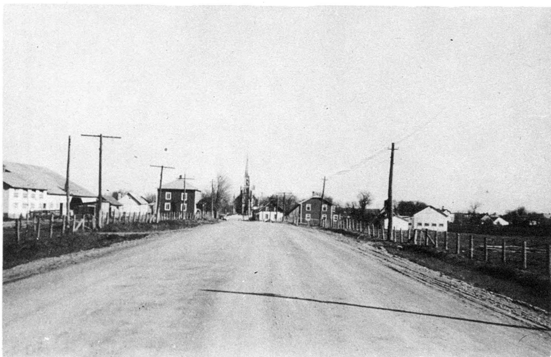
Highway No. 23, near Saint-Henri. Stabilisation before the laying of the bituminous pavement.
