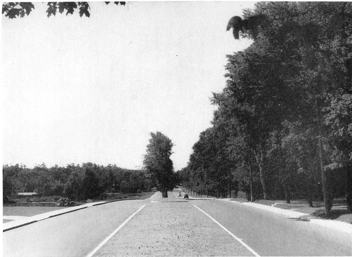
Bituminous concrete pavement laid last summer, on the Sir Wilfrid Laurier Way, at Sillery.
