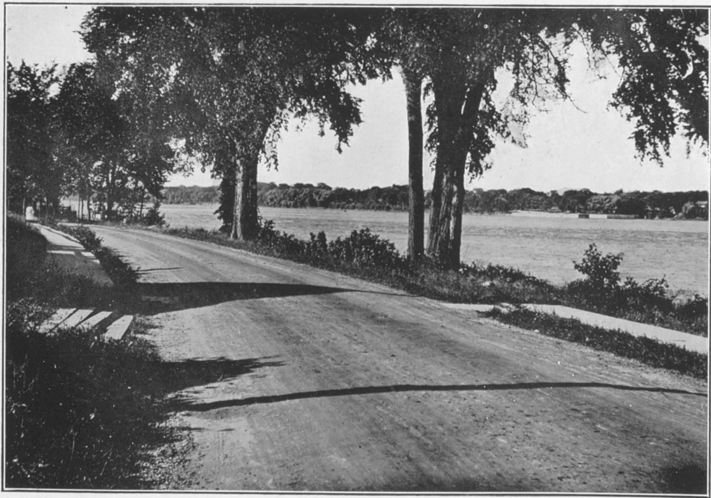
Route VAUDREUIL-POINTE-FORTUNE Highway—Pointe-Fortune Macadam huilé entretenu en régie. Oiled macadam maintained by the Department.
