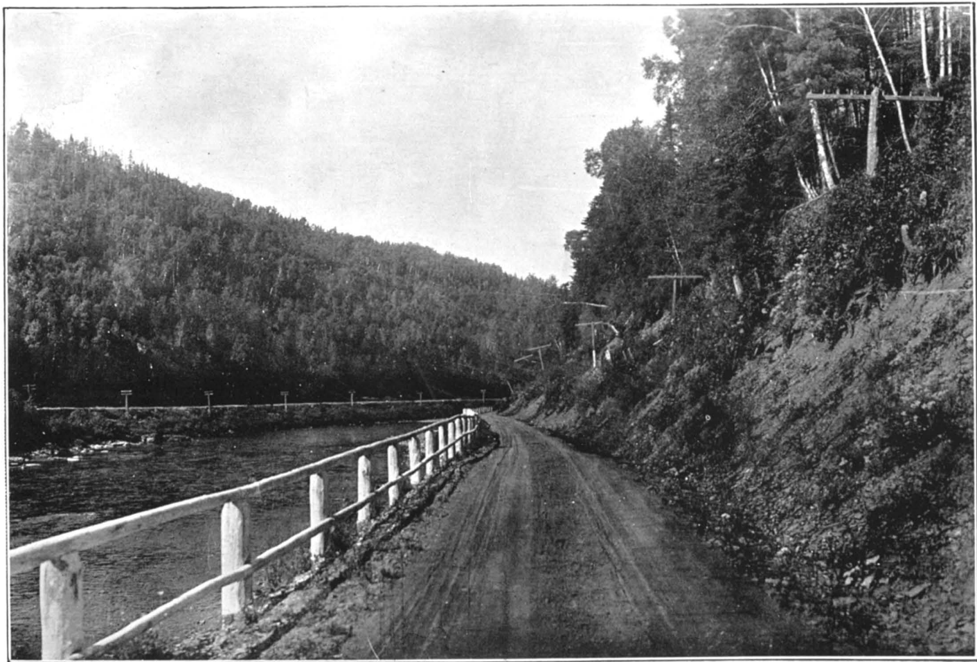
Route RIMOUSKI-MATAPEDIA Highway—Canton Asemetquagan, (township)—Bonaventure Gravelage entretenu par le département. Gravel maintained by the Department.
