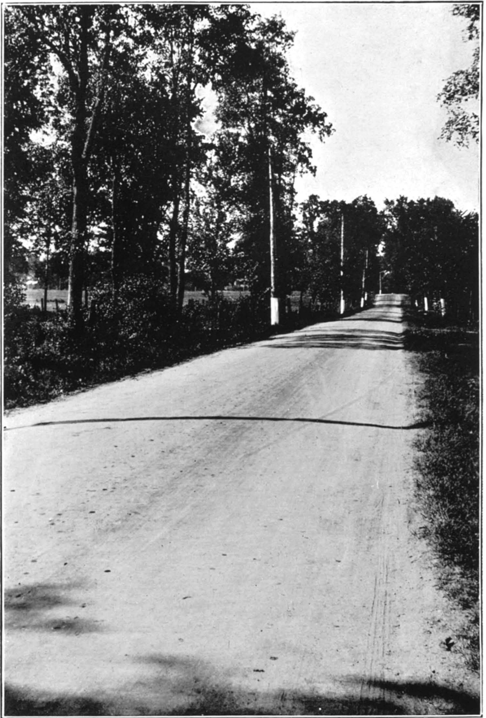
Route VAUDREUIL-POINTE-FORTUNE Highway Como-Est
