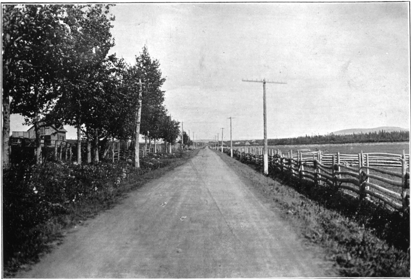
Route RIMOUSKI-MATAPEDIA Highway—Ste-Marie de-Sayabec, Matapédia. Macadam rechargé de gravier. Macadam resurfaced with gravel.
