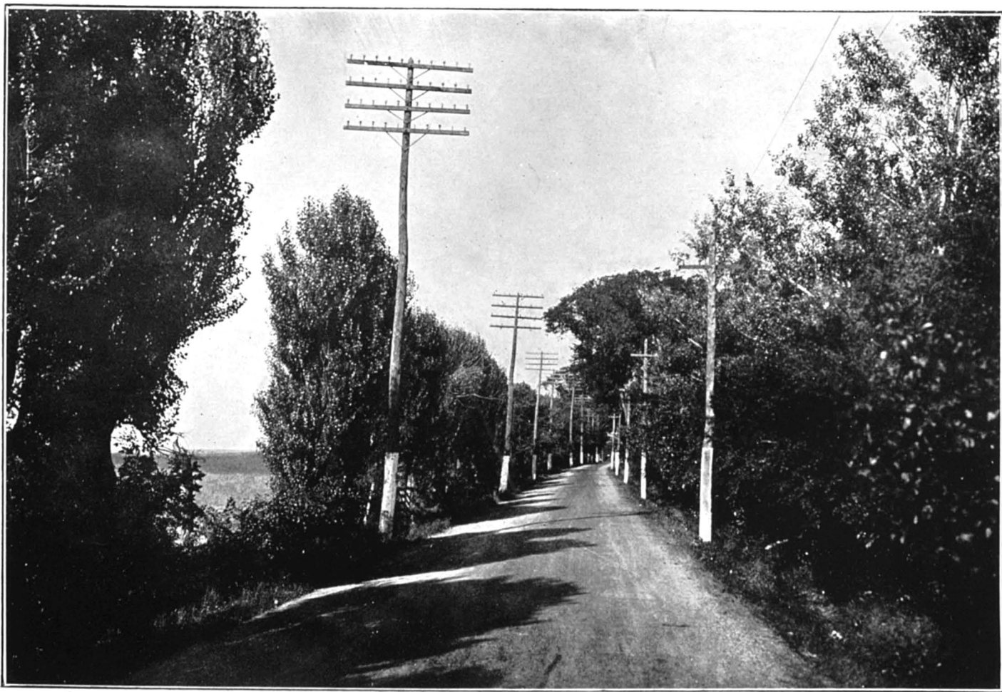
St-Vincent-de-Paul, Laval—Chemin MASSON Road. Macadam entretenu en régie. Macadam maintained by the Department.
