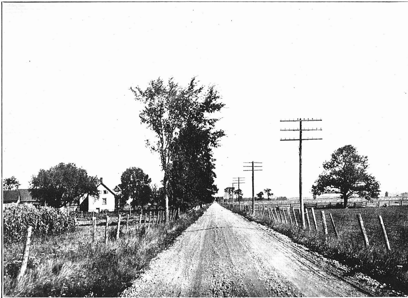
Route MONTREAL ROUSE'S POINT (via St-Jean) Highway—St-Blaise, p. Gravier. Construction de 1924 Gravel. Construction of 1924.
