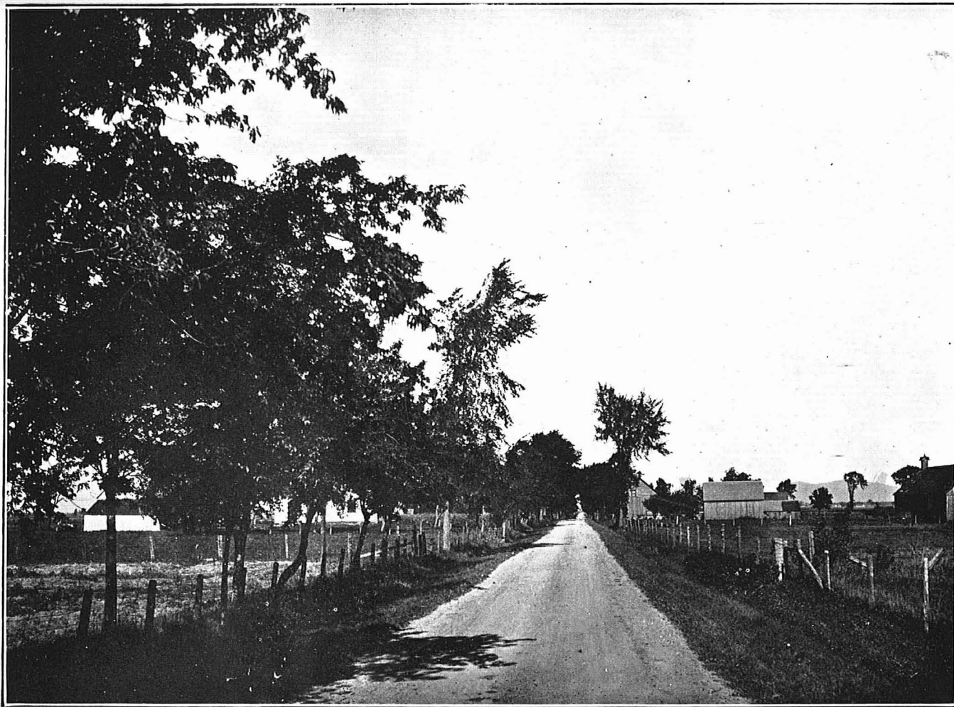
Route MARIEVILLE-COWANSVILLE Highway.—Ste-Marie-de-Monnoir Macadam rechargé de gravier Macadam resurfaced with gravel
