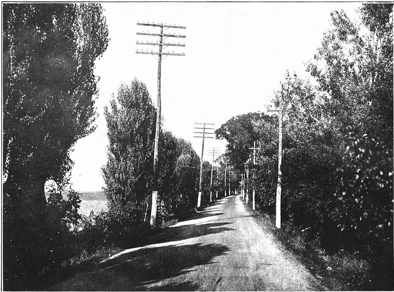
St-Vincent-de-Paul, Laval—Chemin MASSON Road. Macadam entretenu en régie. Macadam maintained by the Department.
