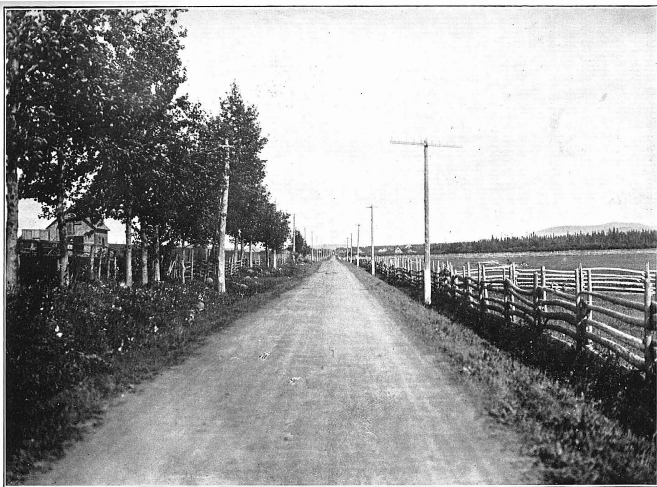
Route RIMOUSKI-MATAPEDIA Highway—Ste-Marie de-Sayabec, Matapédia. Macadam rechargé de gravier. Macadam resurfaced with gravel.
