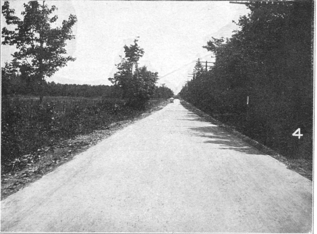
3. Application of coating of asphaltic concrete.—4. The road as finished
