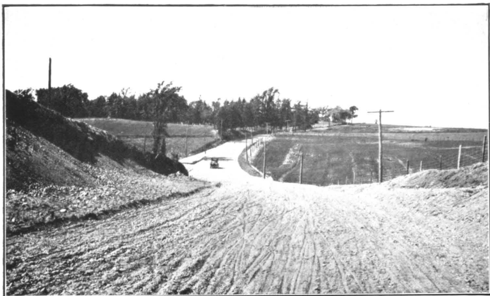
No. 12.—Levis-Jackman road. Sainte Marie (Beauce). On the left is the excavation of the gravel-pit. In the background is the fill (1914) Bedard's hill.
