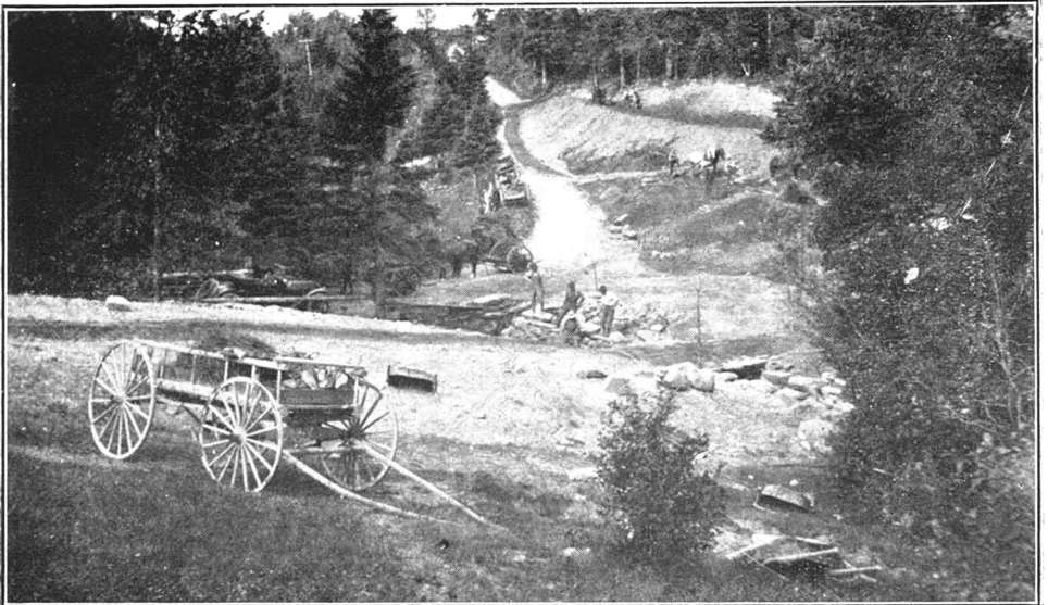
No. 15.—Levis-Jackman road. Saint Georges (Beauce). Donovan hill. On the left is the old hill; on the right are the fill being made and the turn to reduce the slope (1914).
