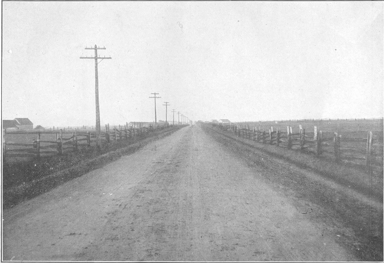
No. 49.—Saint Charles (Bellechasse). North Road. Macadam made in 1914.
