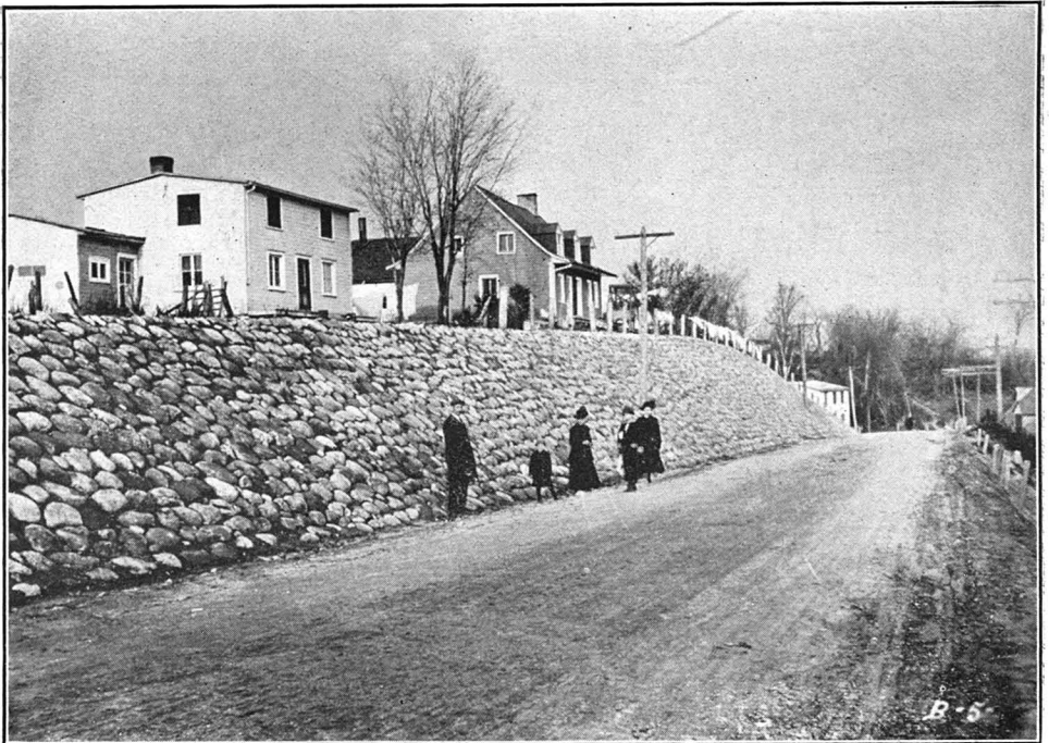
No. 21.—Montreal-Quebec road. Same as in the engraving above which shows especially the wall in dry-stones protecting the slope' Work done in 1914.
