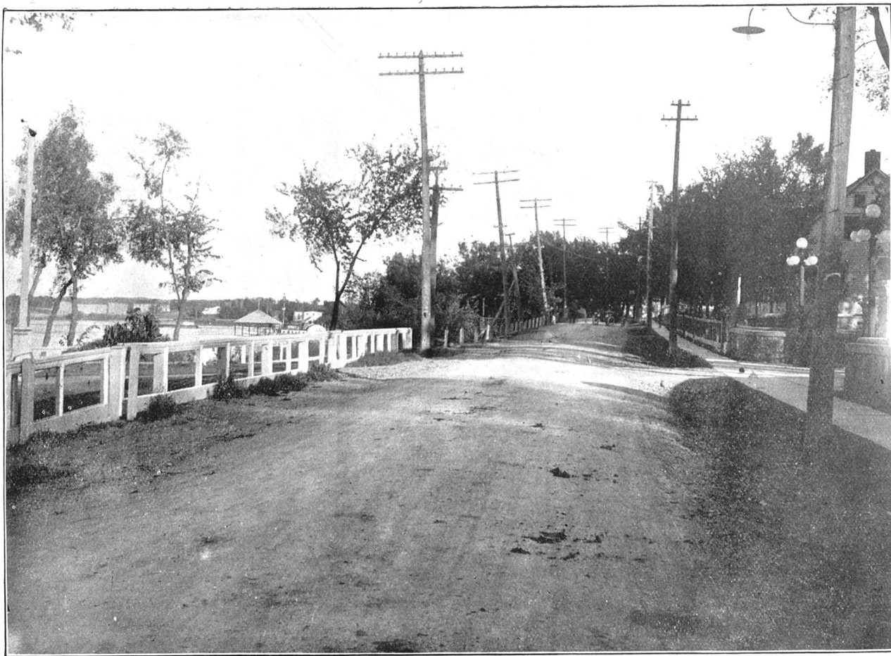
N° 16—Chambly-Basin, county of Chambly. Macadamized in 1913
