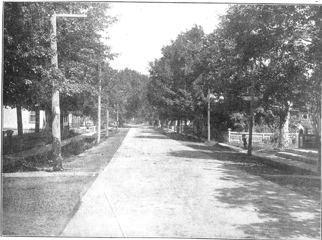
N° 3—Edward VII Road—Village of Napierville. The same road after laying of concrete paving
