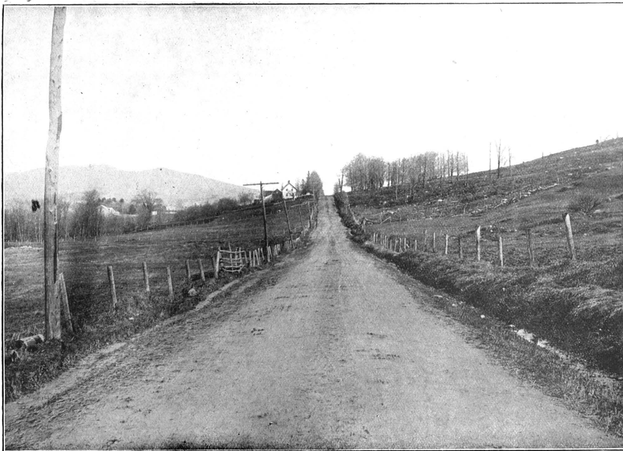
N° 6—Knowlton, county of Brome. Hill macadamized in 1912. This work presented difficulties owing to the presence of springs which necessitated special drainage. Photographed in 1913
