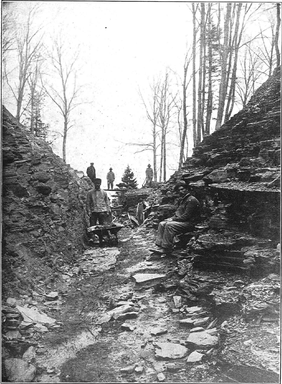
N° 34—Montreal-Quebec road. Cutting for straightening road at Martel's mill, St. Augustin, county of Portneuf
