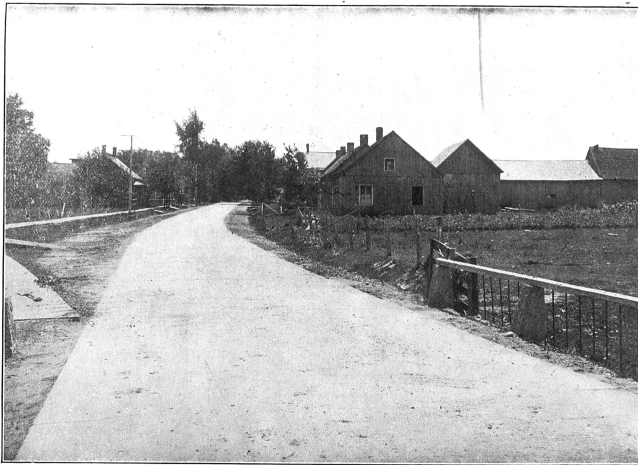
N° 4—Edward VII Road—Village of Napierville. Concrete paving
