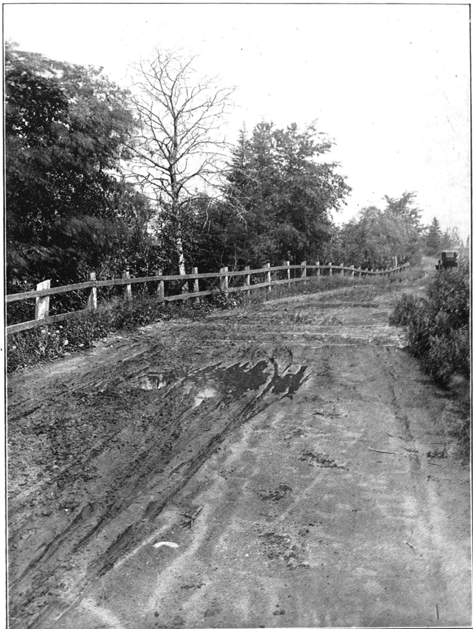
N° 32—Notre-Dame-des-Laurentides, county of Quebec. Lake Beauport road before macadamizing
