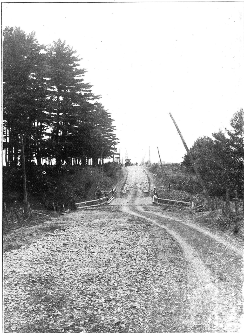
N° 29—La-Baie, county of Yamaska. Preliminary work before macadamizing (1913)
