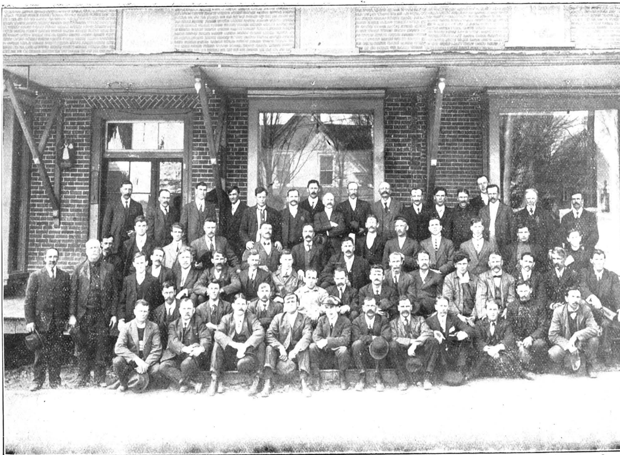
N° 5—Instructors of the Government on the municipalities, who, in the spring of 1913, followed at Knowlton, a course of macadamizing given by the Engineers and inspectors of the Roads Department
