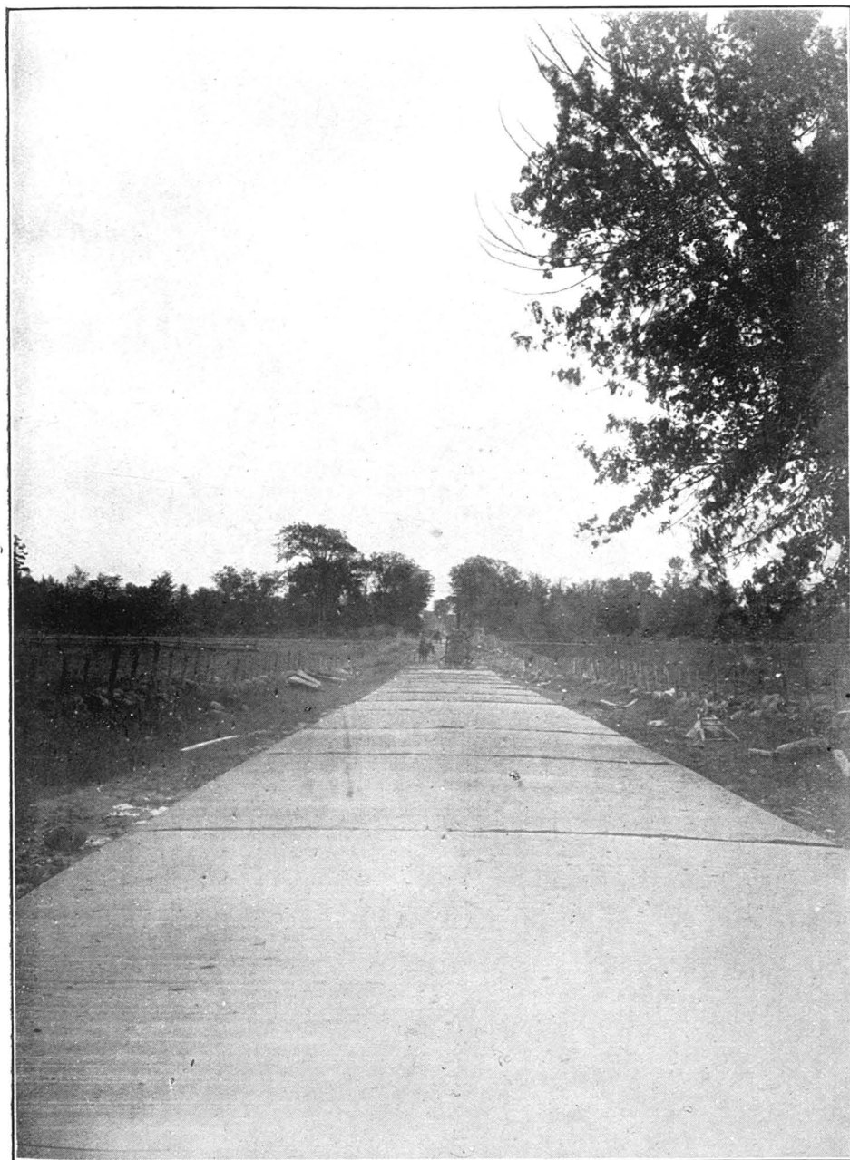
N° 11—Ste. Rose grade, county of Laval. Concrete road made in 1913. (This grade ] will have a total length of 6\frac{1}{2} miles)
