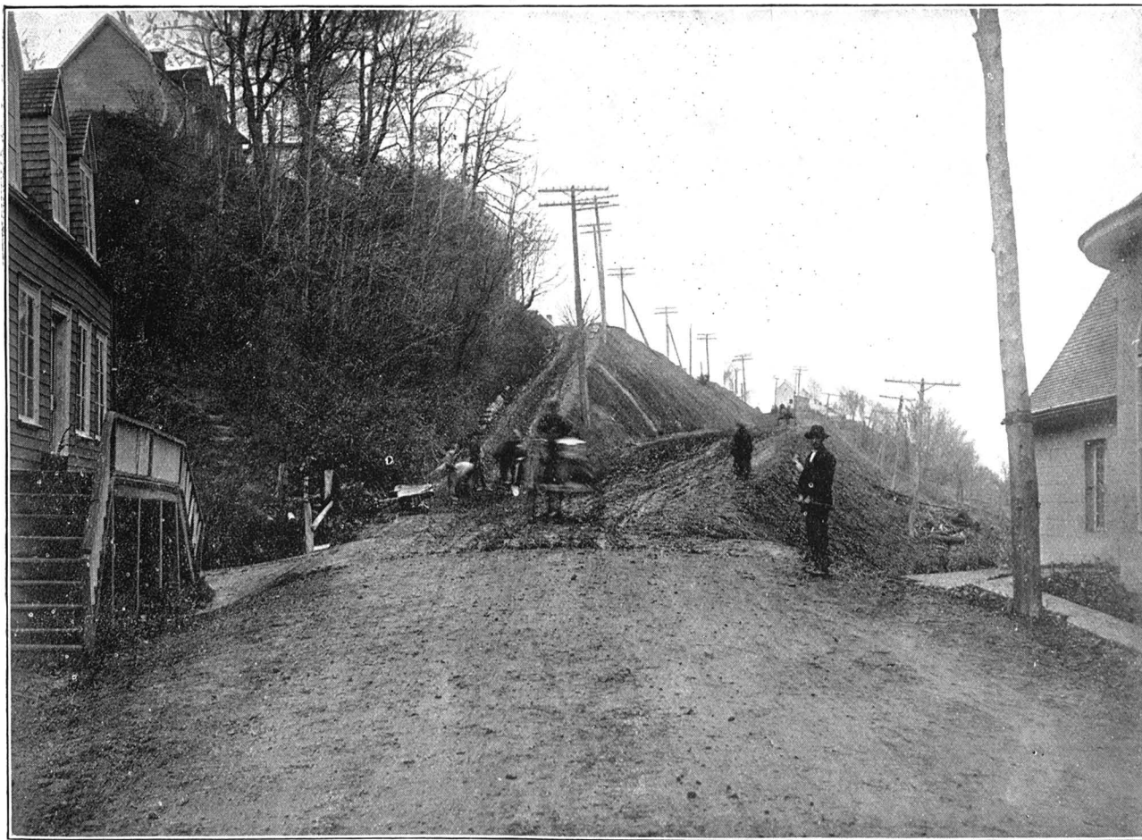
N° 36—Montreal-Quebec road. Les Ecureuils, county of Portneuf. On the left is the old road, on the right is the cut where the new road will be made
