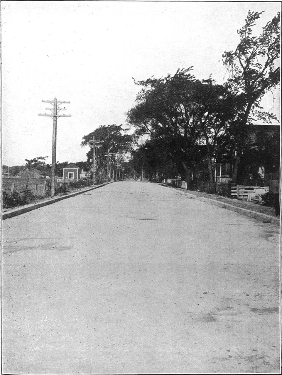
N° 27—Town of Longueuil. Concrete laid in 1913
