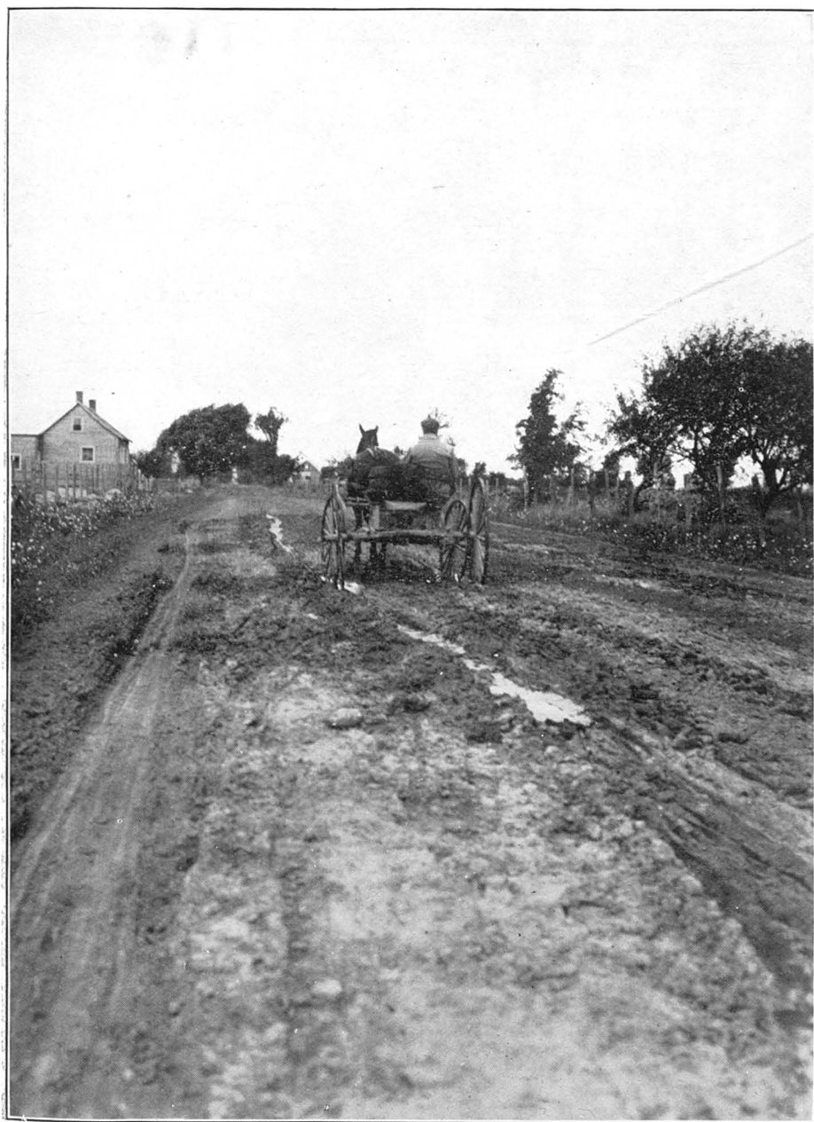
Edward VII Road.—Before macadamizing, municipality of St. James, section No 22, after four days of fine weather.
