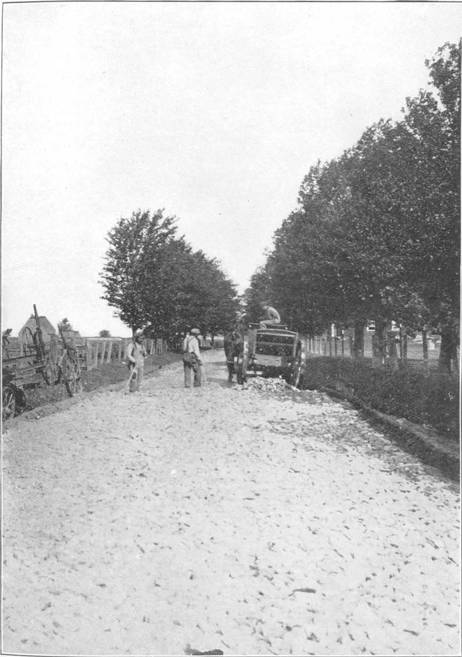
Edward VII Road.—Laying macadam on section No 9, municipality of Napierville, opposite Madame J. Belanger's property, showing the first course of stone.
