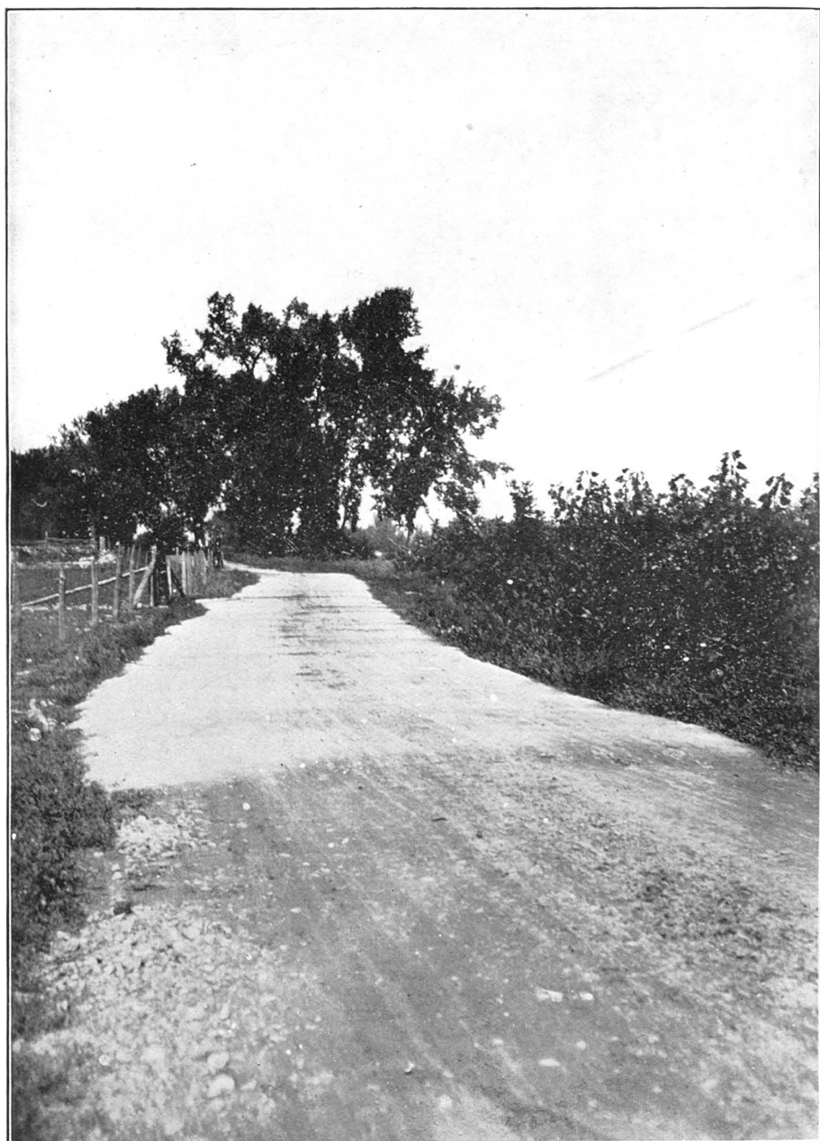
Chateauguay.—Part of road in concrete built in 1911, on east side of River Chateauguay.
