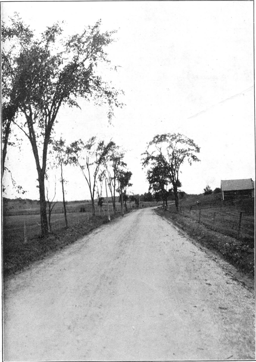
Part of Milby road in township of Compton, macadamized in 1912.
