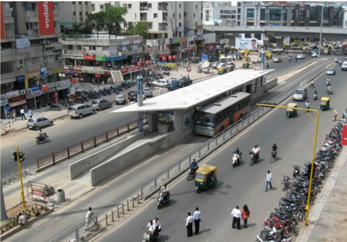
Janmarg, in Ahmedabad, India has stations that are not immediately adjacent to the intersection.
