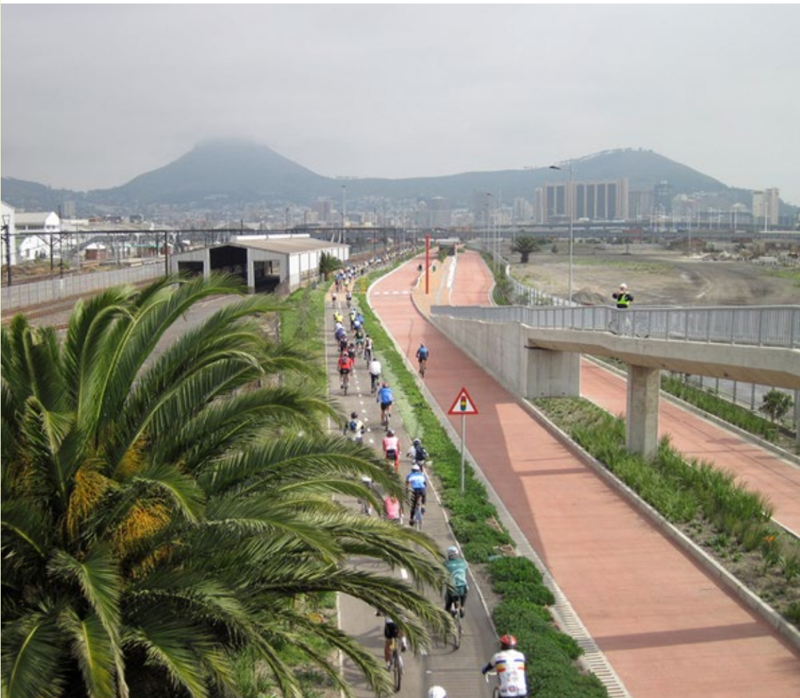
A bikeway is located parallel to MyCiTi, in Cape Town, South Africa.
