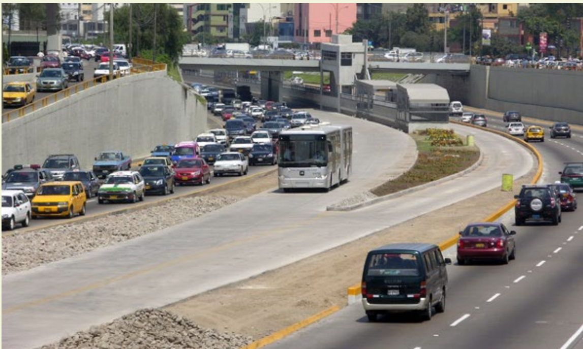
Lima, Peru uses reinforced concrete over its entire busway.
