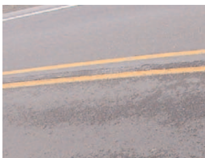
Figure 9-2 Texture non uniforme
