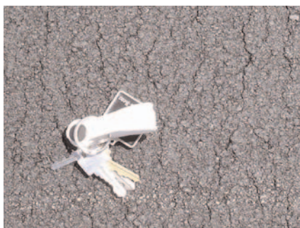
Figure 9-3 Microfissuration transversale
