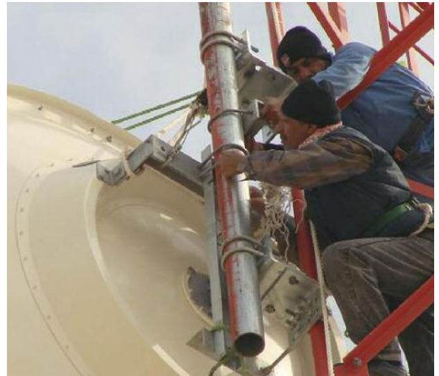
Antenna installation at Umm Qasr. (Photo courtesy Mafeks International, LLC)
