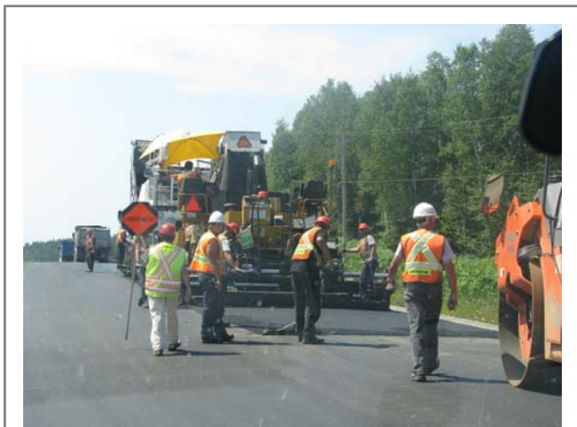
Travaux routiers Route 117 - Arntfield
