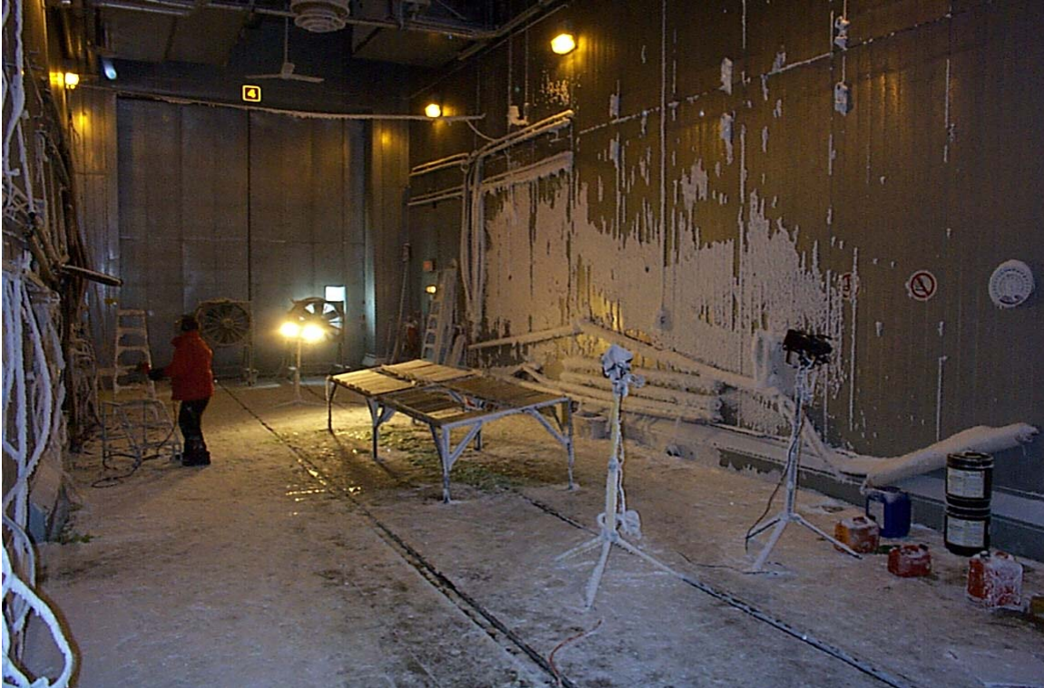
Photo 2.5 Inside View of Large End of Climatic Engineering Facility
