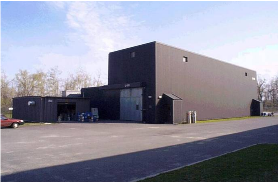
Photo 2.3 Outdoor View of NRC CEF
