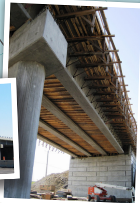
Installation of the formwork for slabs on the Chemin Saint-François-Xavier overpass is underway. This work will be completed by the end of June.
