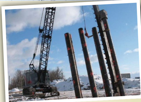
Installation of piles for the Rue Saint-Pierre overpass.
