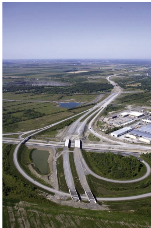
Aerial view of the 15/30 interchange at the approaches to the municipalities of Delson and Candiac.
