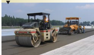
Paver with high compacting capacity.
