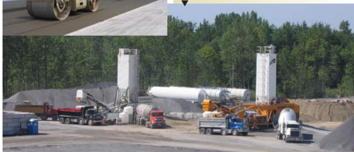
Portable "pugmill" system for the on-site production of RCC
