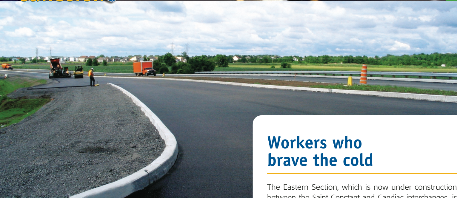
The Haute-Rivière work site in Châteauguay, was the location of a life-sized test bed that served to assess soil quality in the Western Section.
