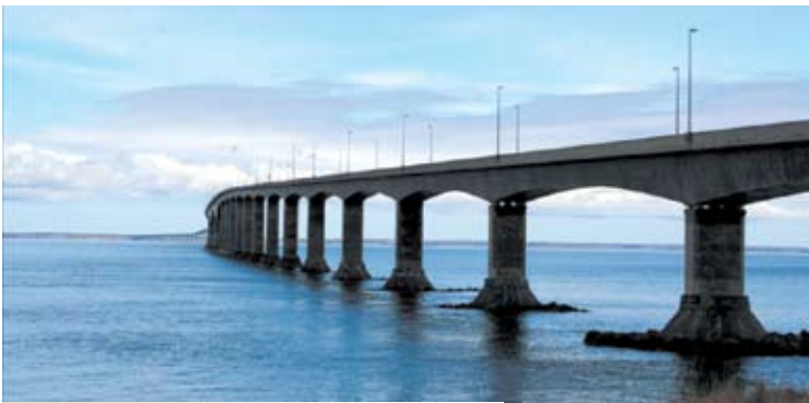
The Confederation Bridge in New Brunswick was built as a PPP. Source: Transports Canada.
