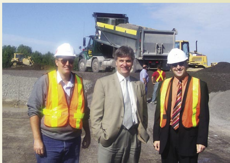
Mr. Fournier visited the work site on Chemin de la Haute-Rivière on August 25, in the company of Mr. Yves Melanson, MTQ Project Manager with the Direction de l'Ouest-de-la-Montérégie, and Mr. Hubert Dubois, Associate Director for Séguin (Séguin-Tecscult is entrusted with the supervision of the site).
