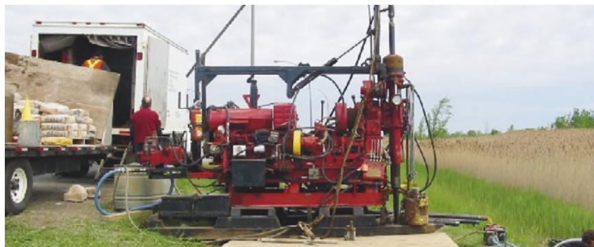
Equipment used for this type of drilling in quick clay.
