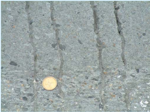
Figure 2 : Rainurage transversal
