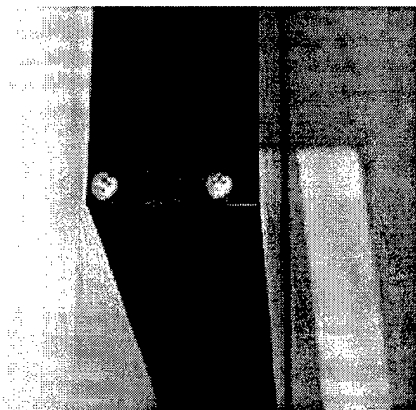
a. Top view of corner connection (pan head sheet metal screws).
