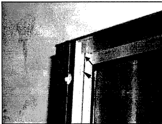
c. Back view of corner connections (arrow points to sheet metal screw in open extruded channel).
