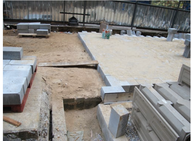
São Paulo, Brazil Drainage channels under construction for a street repaving project.
