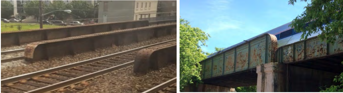
Figure 124. Photos. Railroad bridge girders with turned-down flanges.
