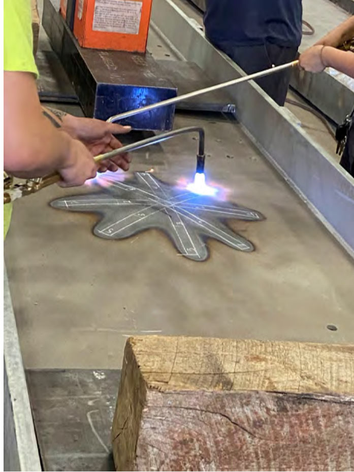
Figure 52. Photo. Web distortion repair with line heats.
