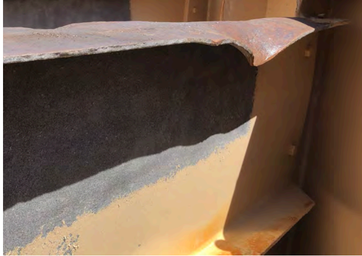
Figure 101. Photo. Typical category L/U damage.
