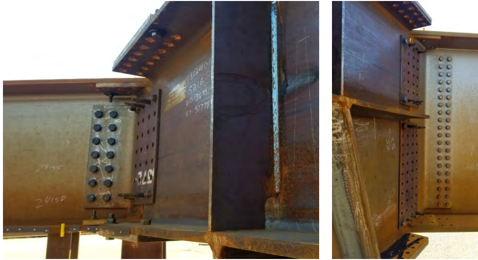
Figure 128. Photos. Cold-bent connection plates.
