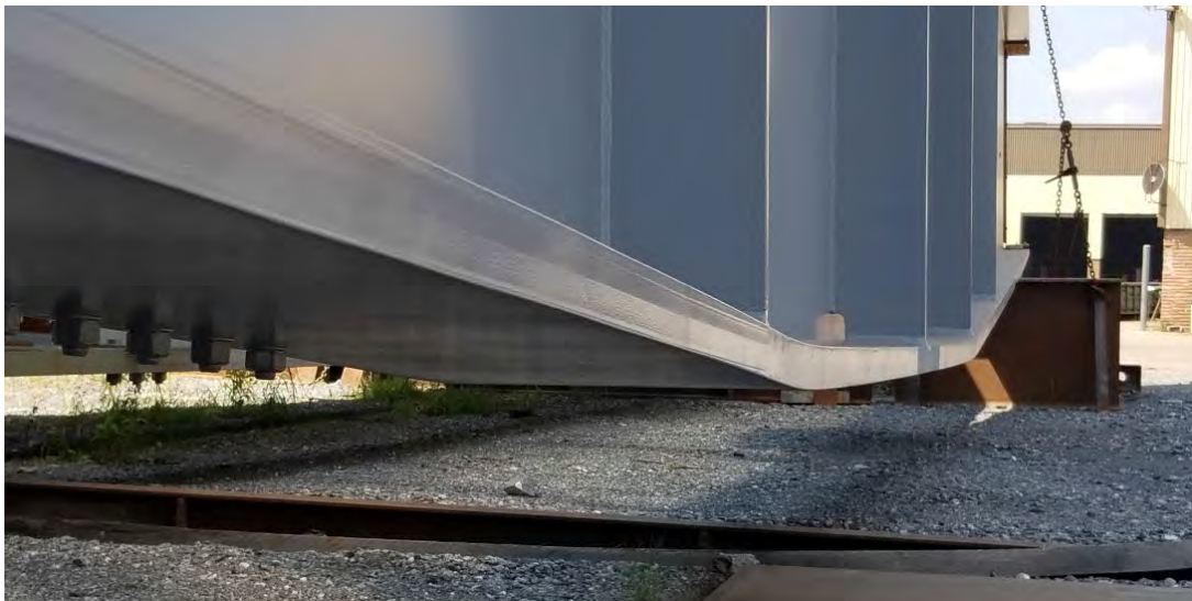
Figure 122. Photo. Cold-bent flange corner on haunch girder.
