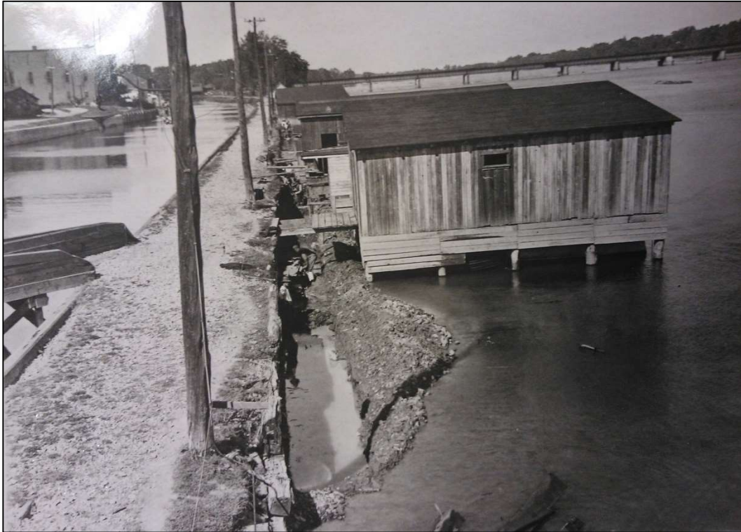
Figure 62 : Wing dam upper entrance Trench for concrete wall on outer side of dam, looking north , 13 octobre 1921 (source: Parcs Canada 156/00/1C-170).
