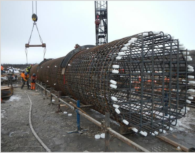
3.40 Large 3.0 m diameter pre-fabricated cage. Extra support / bracing used to retain shape and stability for lifting.
