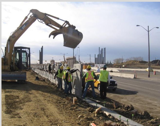
25.5 Installation of first course of panels.
