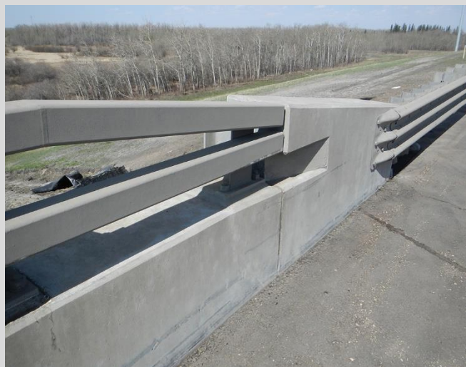
12.5 Bridgerail to guardrail transition.
