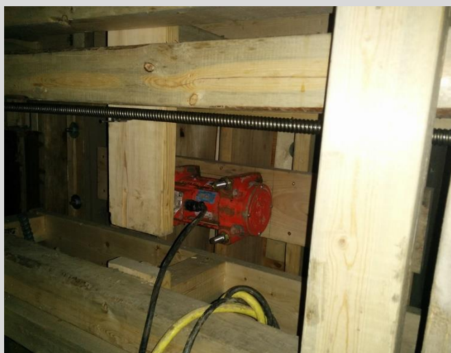
4.27 External vibrator attached to form. Due to congestion of reinforcing steel and post-tensioning ducts, internal vibration difficult.
