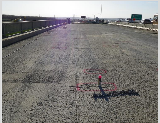
20.2 ACP removed and locations requiring full or partial depth repair are identified and marked out with paint by the inspector.
