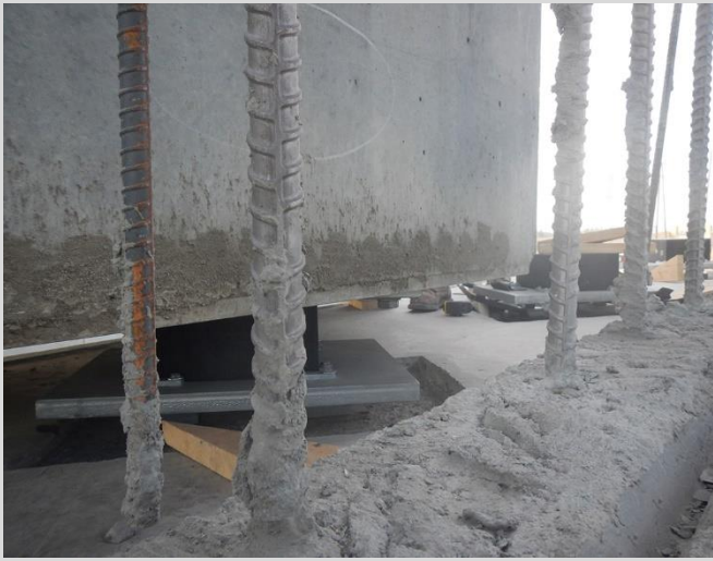
7.9 Concrete box girder on bearing.
