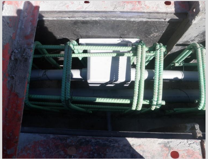
11.6 RWIS junction box cast on outside face of barrier. Box must be sealed to prevent contamination with concrete paste.
