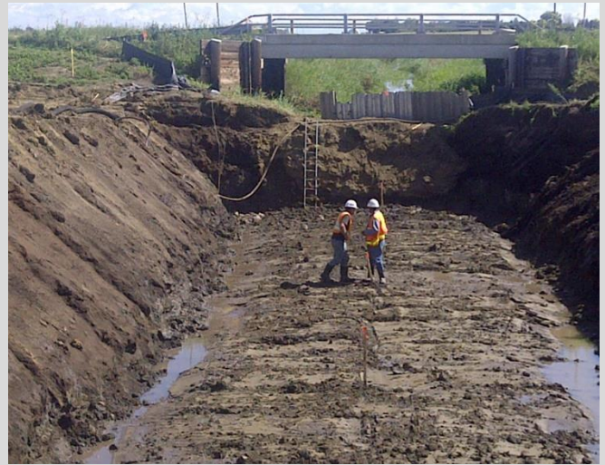
1.2 Channel excavation for culvert construction. Channel bed crowned and graded to shed water. Existing stream diverted with sheet piling and clay berm. Slopes cut at 1:1 for safety.
