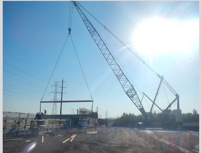
7.12 Erecting concrete box girders from approach fill.
