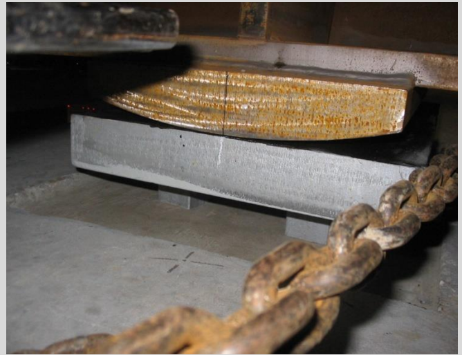
6.10 Girder and rocker bearing. Centre line of bearing marked on rocker, base plate and pier cap. Bottom of rocker plate machine-finished.
