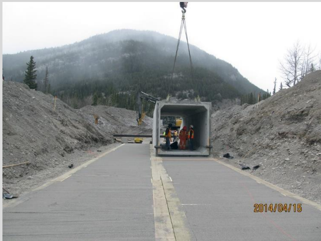
26.17 Erection of PBC units.
