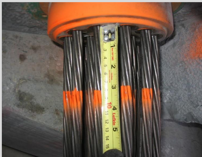
7.28 Tendon elongation measurement taken from wedge plate.
