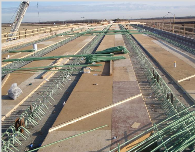
4.45 Deck formwork in place on concrete girders.
