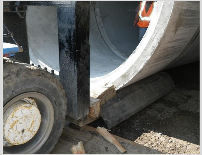
26.10 Joining RCP sections. Typically done with chucks or winches. Rubber softeners and 2x6 blocks used here to lift and push pipe.
