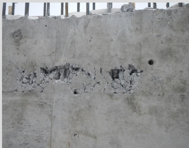
4.95 Honeycomb defect.
