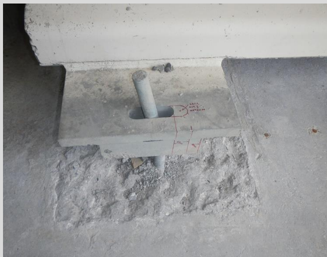
8.16 Improperly set bearing resulting in bent anchor rods and failed grout pad.
