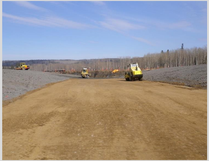
18.2 Compacting of culvert bedding material.
