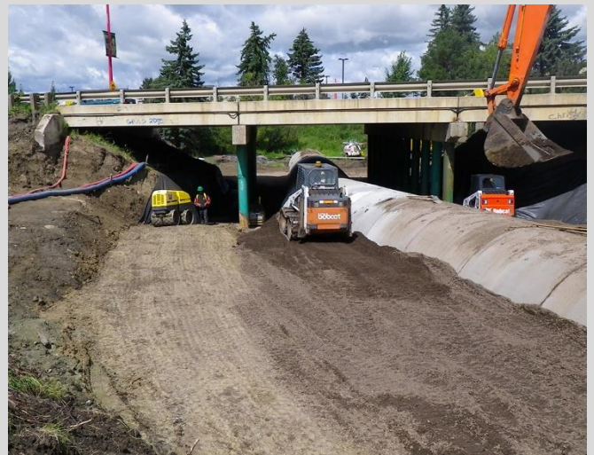
26.12 Both sides of pipe simultaneously backfilled. Skid steer and remote controlled walk behind packer used to compact material.
