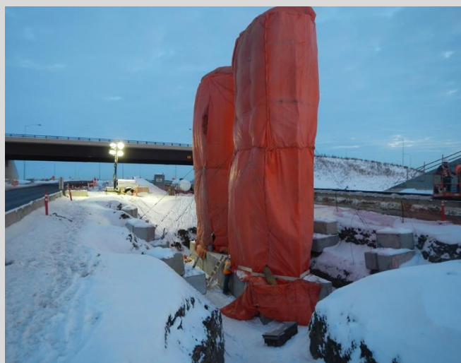
4.28 Cold weather concreting. Hoarding for pier columns consists of insulated tarps and heaters.
