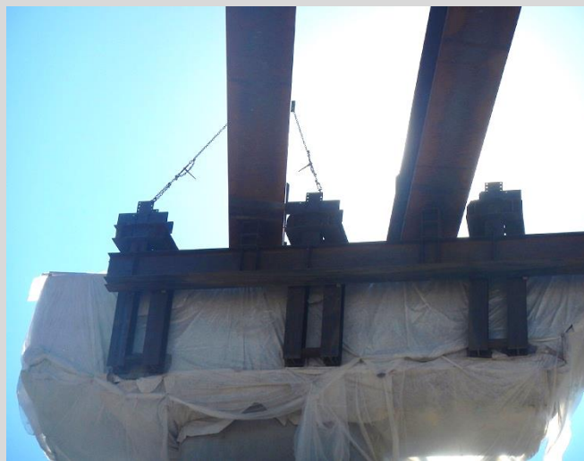
6.6 Temporary bracing, tie downs secured to pier and girder. Diaphragm installation completed prior to release.
