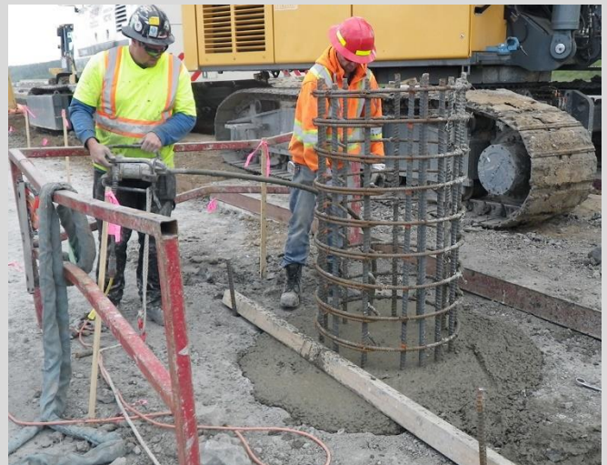
3.35 Vibrating top of pile. Efforts should be made to keep reinforcing steel free of paste.
