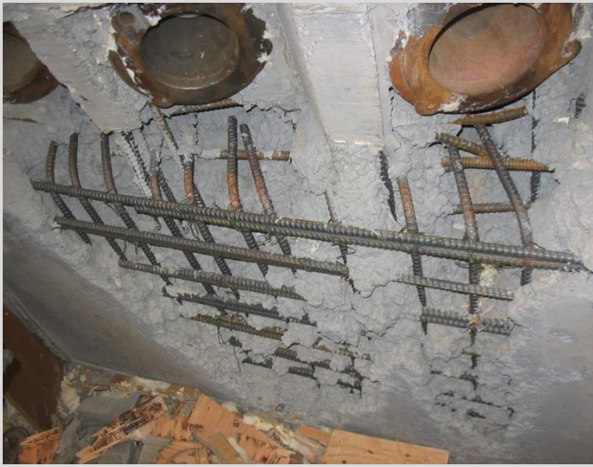
7.40 Severe honeycombing on pier cap due to congestion at post tensioning tendon heads.
