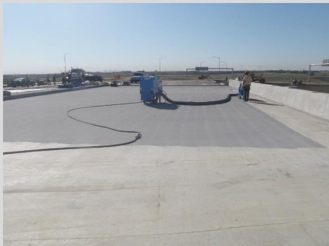
16.3 Surface preparation by shot-blasting.
