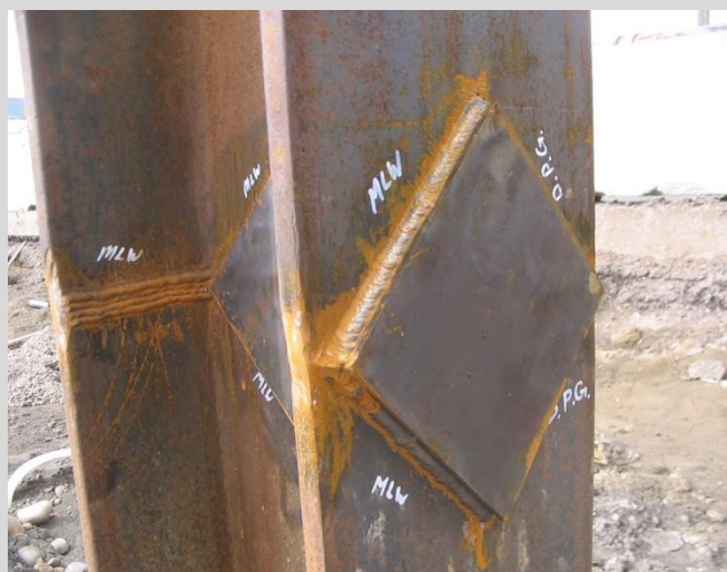
3.10 Completed H-pile splice welds.
