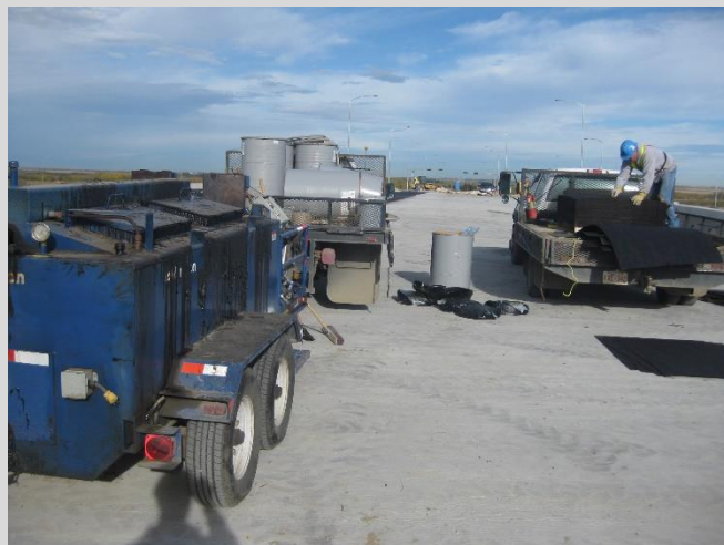
16.4 Waterproofing equipment and materials. Heating and mixing kettle on site. Workers unloading protection board.
