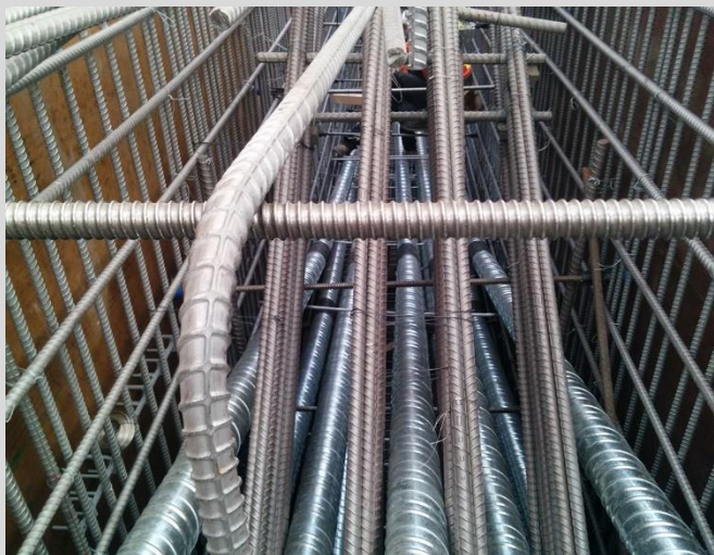
7.22 Post tensioning ducts at pier cap. Smooth profile throughout length of tendon.
