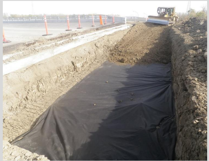
2.2 Soft soil at base of excavation removed and replaced with competent granular back fill.
