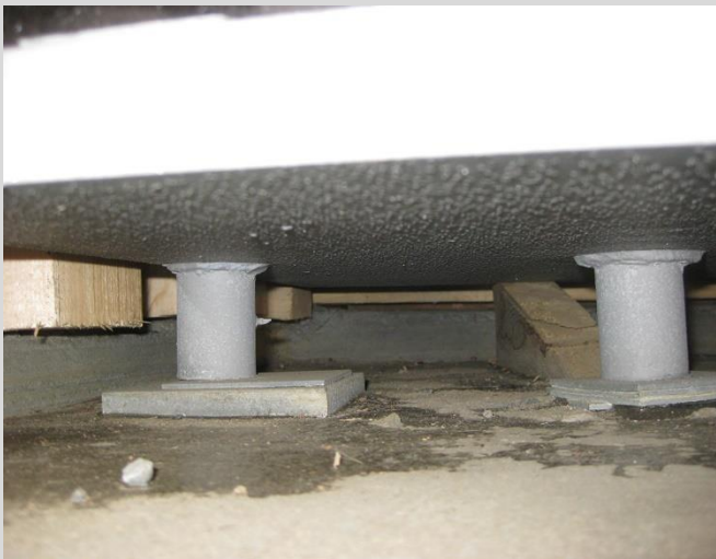
8.7 Bearing elevation set using shim stacks placed under pintles. Pintles allow bearing to rotate. Underside of plate is coated to prevent direct contact between zinc and grout.
