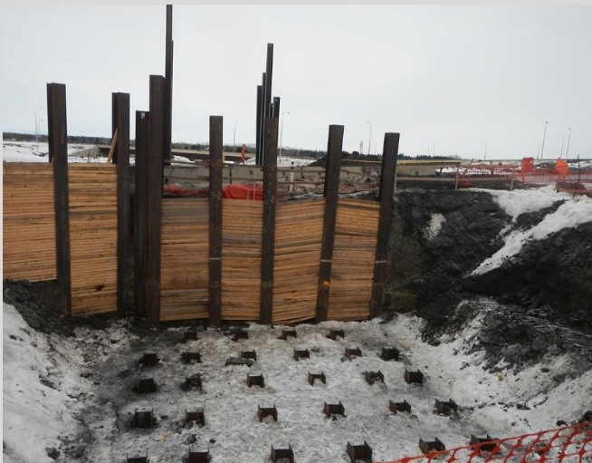
1.3 Pier excavation for pile cap. Piles cut off at elevation. H-piles and lagging for temporary retaining wall shown.
