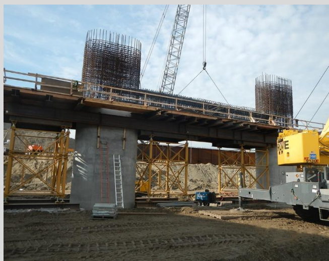
4.13 Pier strut shoring towers and scaffolding. Pre-fabricated reinforcing steel cage installed by crane.
