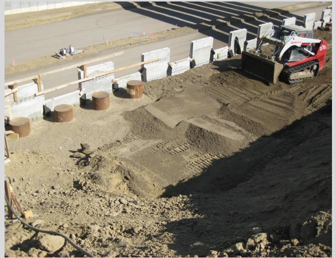
2.6 Skid steer loader used to spread 150 mm granular fill for MSE wall fill.
