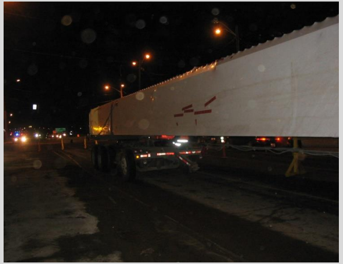
6.23 Steel girder delivery. Girder covered in plastic wrap to protect from road salt and contamination during transportation.
