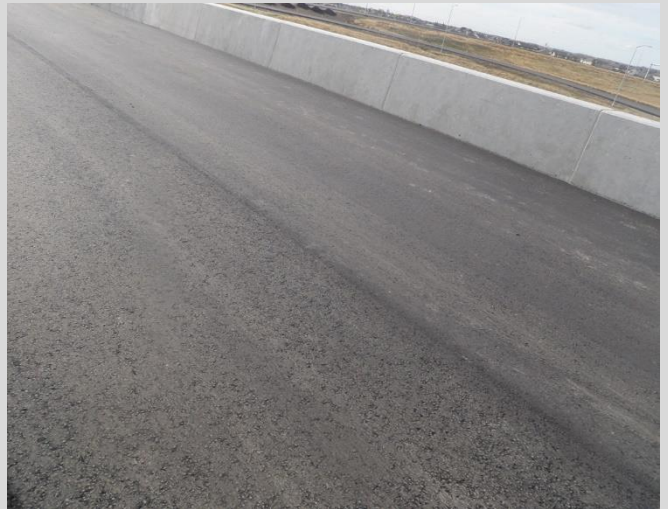
17.12 Unacceptable segregation in travel lanes.
