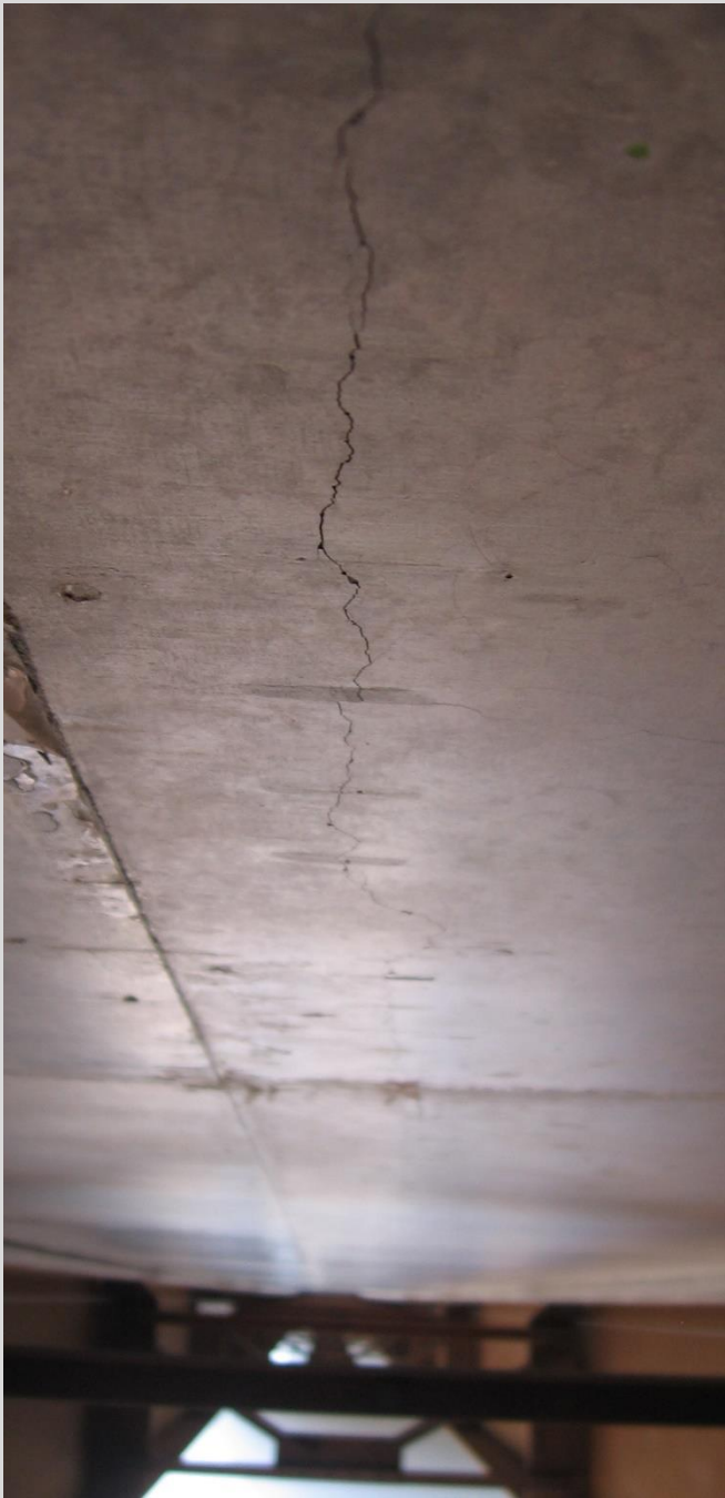
4.99 Deck slab soffit drying shrinkage crack.
