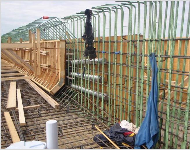
7.17 Cast-in-place girders with post tensioning ducts. U-bars set at 1.0 m spacing to secure duct elevations.
