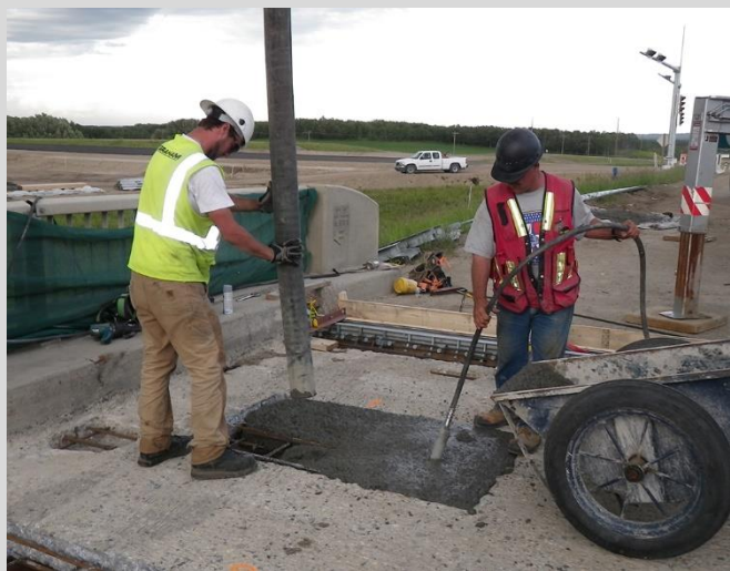
20.9 Concrete being placed into repair area.
