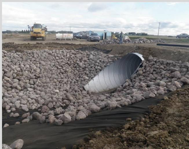
10.4 Riprap placed at the end of culvert bevel.
