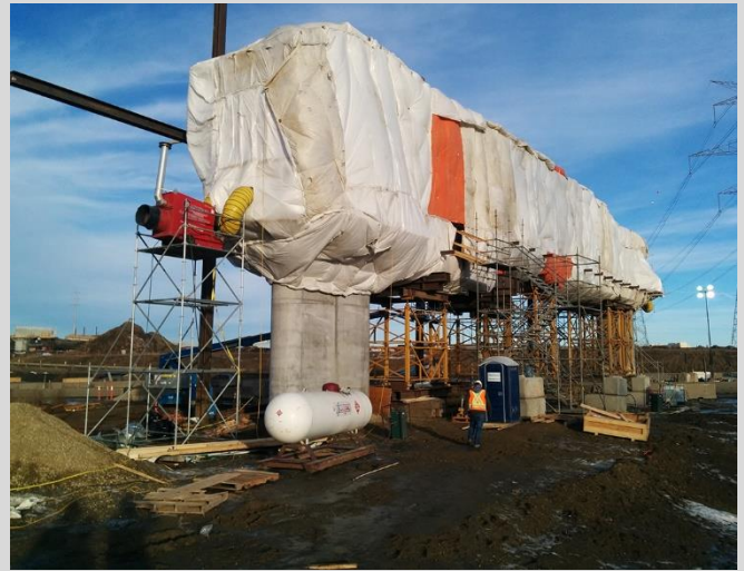
4.24 Scaffolding and shoring towers for straddlebent pier beam. Heating and hoarding for cold weather concreting in place.
