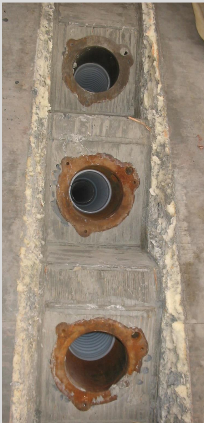
7.23 Post tensioning ducts cast into pier cap. Tendons to be installed, stressed and grouted.
