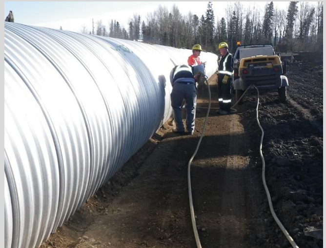
18.32 Backfilling and compacting haunch area.
