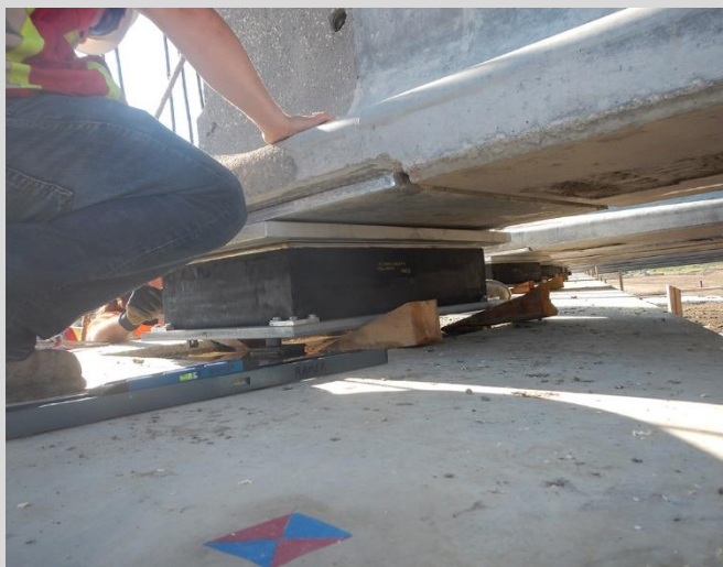
7.13 Setting NU girder onto bearing. Survey layout/control visibly marked on abutment seat.
