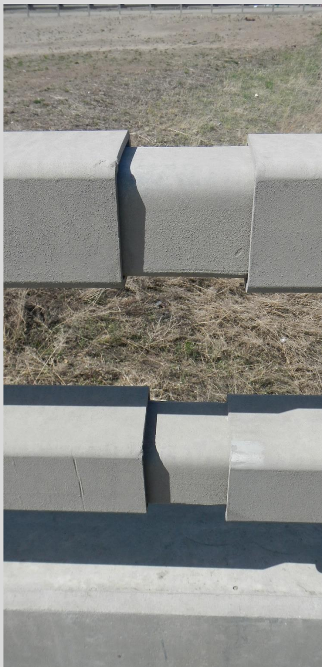
12.3 Expansion joint sleeves between rail sections.
