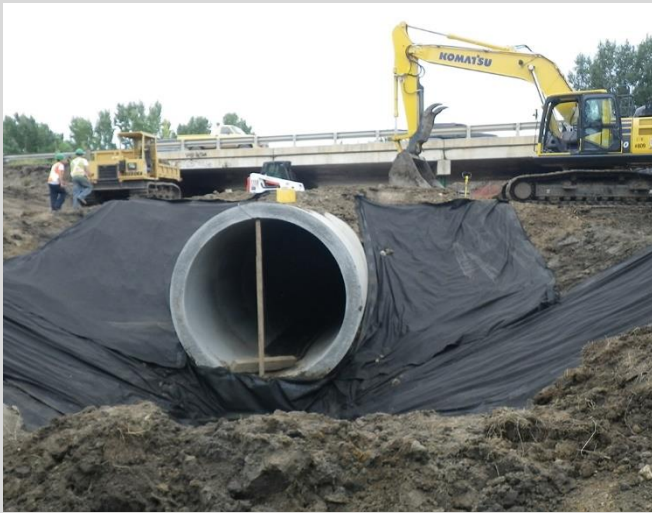
26.13 Clay seal compacted at end of pipe. Filter fabric material in place.
