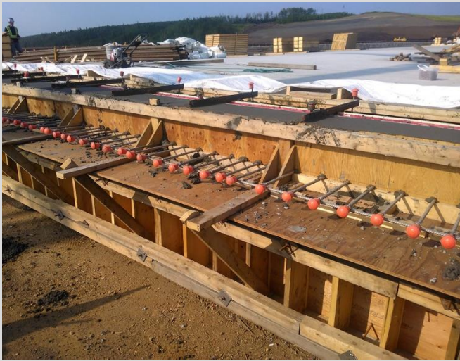
4.31 Backwall corbel formwork.
