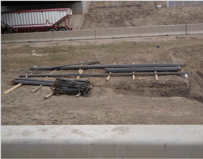
5.1 Proper storage of plain reinforcing steel on timber dunnage in dry location.
