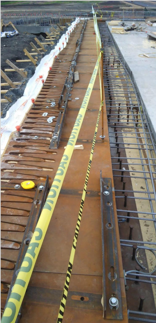
6.20 Finger type joint showing deck-side block-out.
