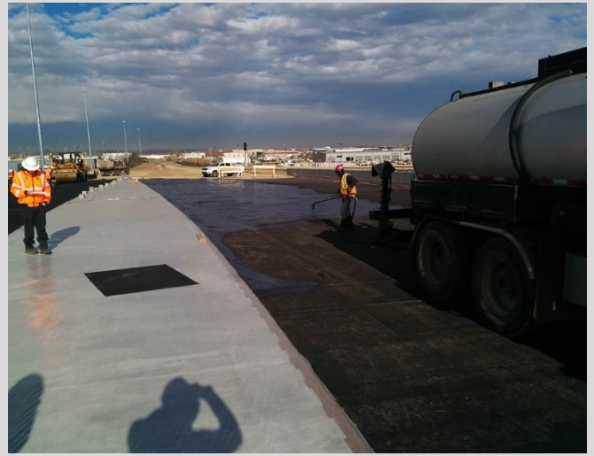
17.2 Application of tack coat by hand sprayer.
