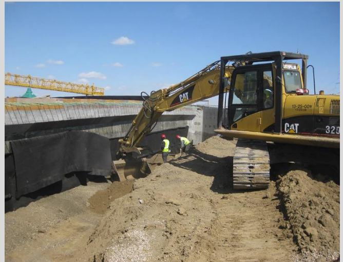
2.4 Hydraulic excavator placing granular backfill material against abutment backwall. Sheet drain placed against abutment seat.
