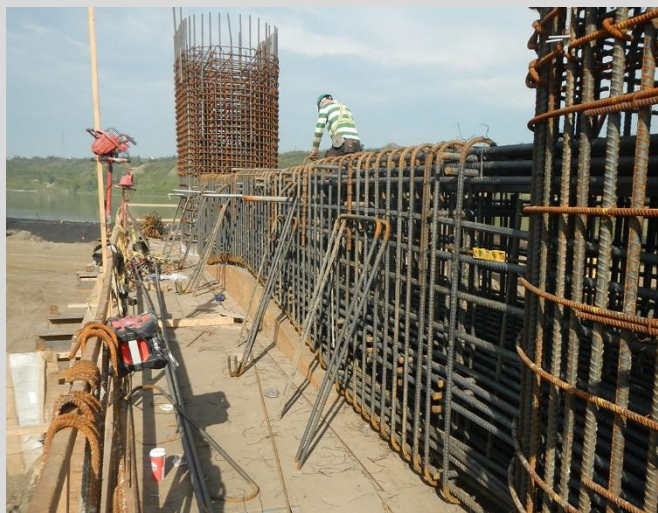
4.14 Pier strut with plain steel reinforcement.
