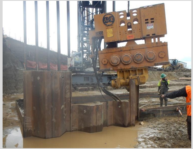
1.13 Sheet piling and frame for pier offerdam. Vibratory hammer advancing sections of sheet piling.
