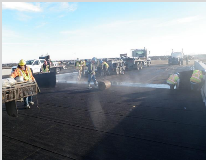
16.11 Protection board is rolled with a water-filled garden roller before membrane cools.
