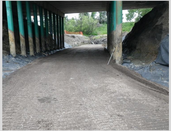
26.2 Bedding material placed and compacted.
