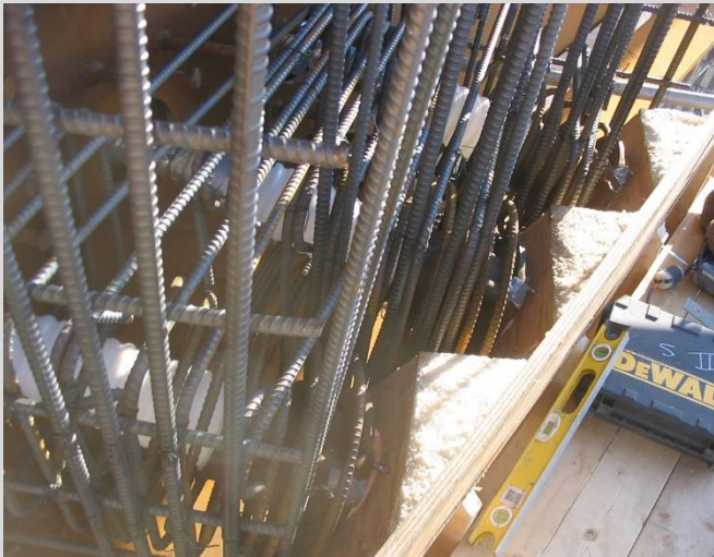
7.19 Post tensioning ducting in pier cap. Congested reinforcing steel exists at pier cap ends.
