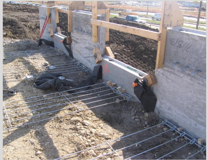
25.10 Wooden wedges used to engage panels. Filter fabric placed over panel joints to prevent loss of material through gaps.
