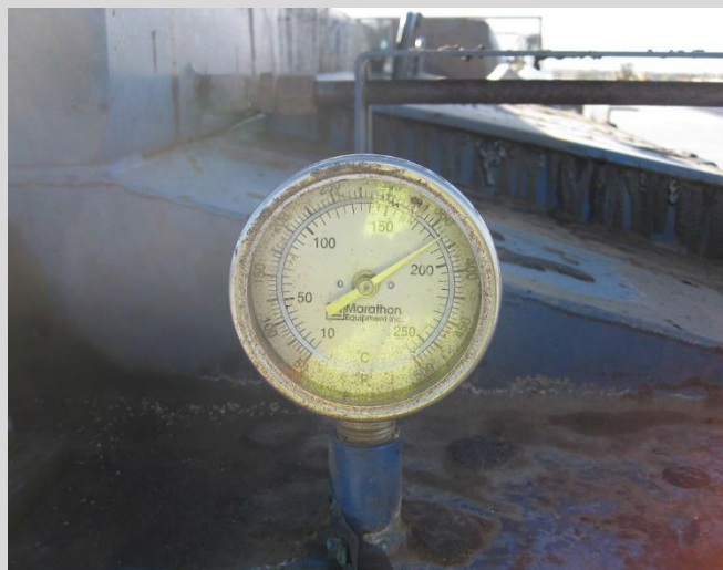
16.6 Asphalt membrane heating in kettle.
