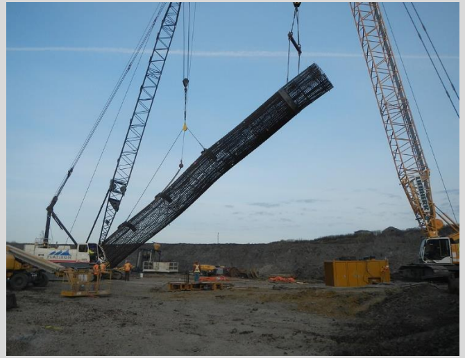
3.41 Double crane pick for reinforcing steel cage installation. Halo ring and extra reinforcement required to pick large cage.
