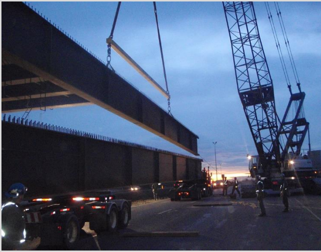
6.1 Steel girder delivery and erection. Spreader bar used for unloading and erecting girders when using a single crane.
