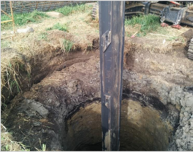
24.1 Drilling foundation pile.
