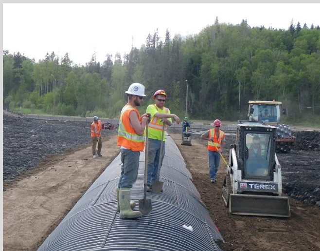
18.9 Backfilling of SPCSP. Small equipment only permitted to work within 1.0 m of pipe. Backfill progressing evenly on both sides of the pipe.
