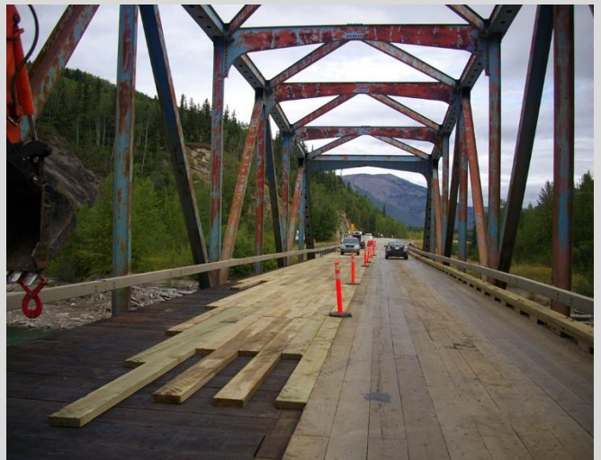
23.4 Strip deck replacement ongoing, boards staggered.
