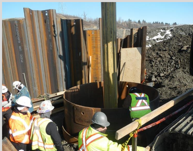
3.39 Piling ongoing. Checking depth of pile and condition of base.
