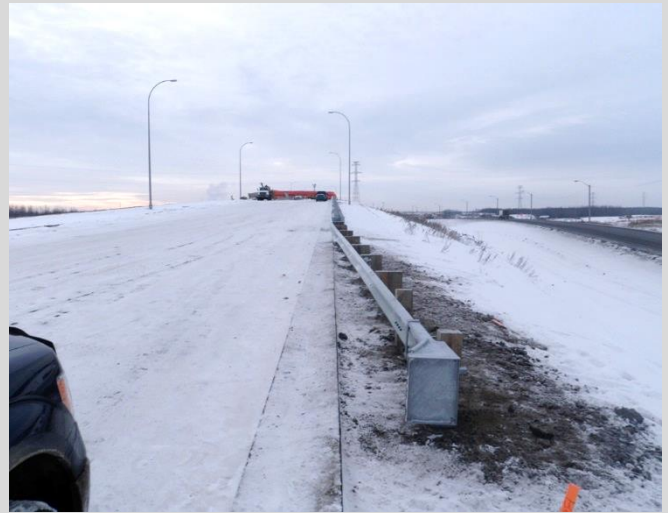
14.6 Guardrail and posts with end treatment.
