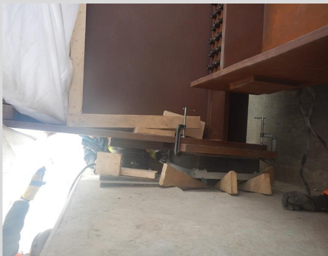
6.26 Setting elastomeric bearing. Wood wedges used to adjust and secure the bearing until girder is in place.
