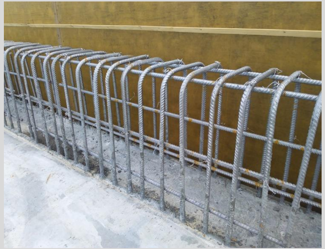
4.79 Typical rough vibrator-finish at barrier construction joint. Note that concrete surface at construction joint slopes towards deck and away from outside face of barrier.
