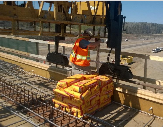
4.41 Cantilevered formwork at deck overhangs must be pre-load tested to determine anticipated deflections during concrete placement.
