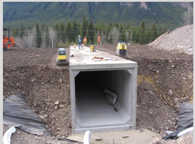
26.20 Backfilling of PBC culvert.
