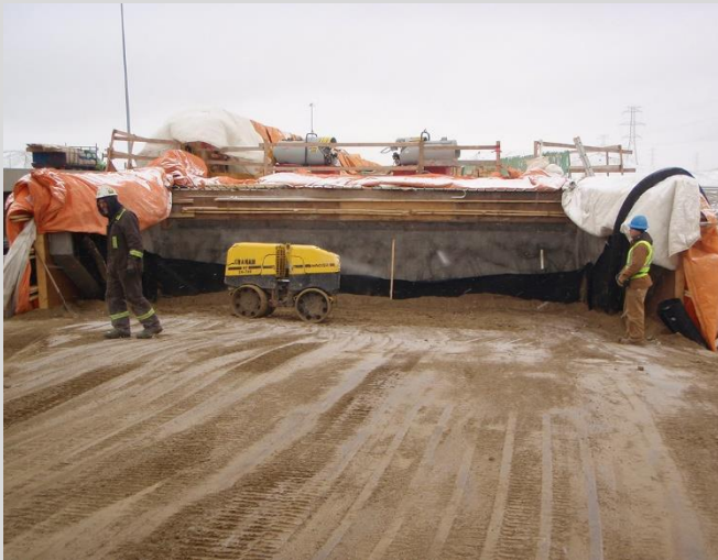
2.3 Compaction of granular backfill behind abutment diaphragm and wingwalls using walk behind remote controlled compaction equipment.
