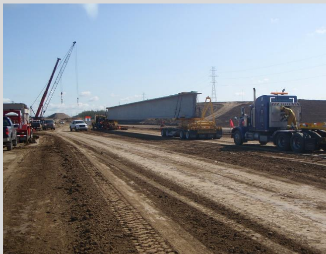
7.1 Precast concrete NU girder delivered to site.
