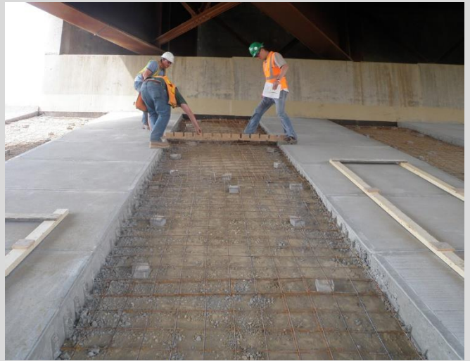
4.114 Checking cover and alignment.
