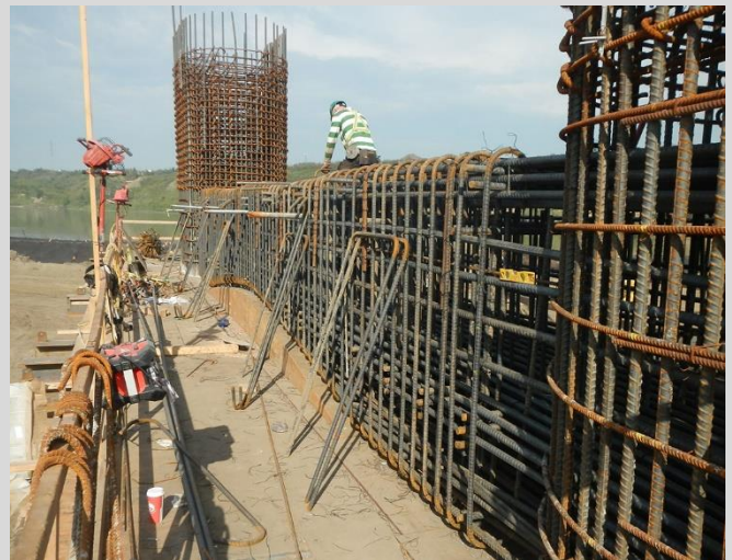
5.4 Pier strut consisting of plain reinforcing steel.
