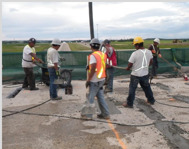
20.10 Concrete being placed into repair area.
