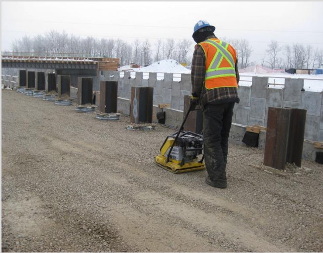
2.5 Hand-operated plate tamper used for compacting granular material between H-piles and against MSE wall fascia panels. Smaller compaction equipment must be used near fascia panels.
