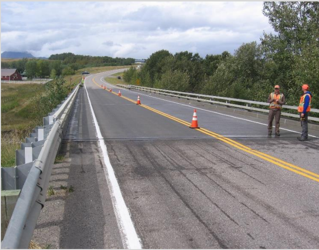
19.1 Protecting paint with cones during curing period.
