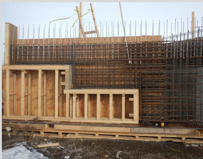
5.5 Wingwall reinforcing steel. CRR projecting for barriers.
