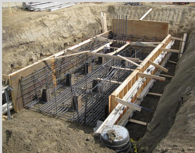
4.2 Pile cap partial formwork and reinforcing steel. Formwork braced from excavation walls.
