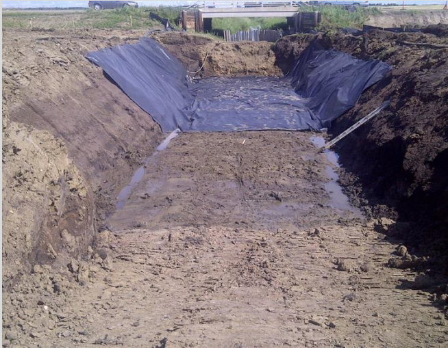
18.15 Excavation for culvert bed. Excavation crowned and sides trenched to control water.
