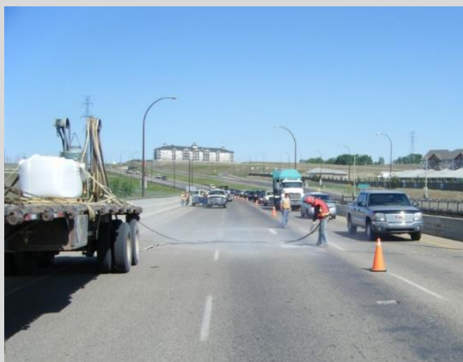
15.3 Surface preparation completed by sandblasting.
