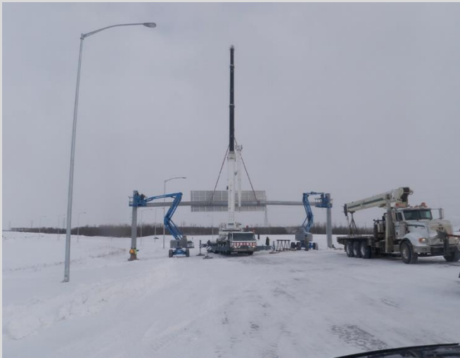
24.7 Sign structure erection. Workers tightening bolts to connect horizontal and vertical columns using aerial lifts.
