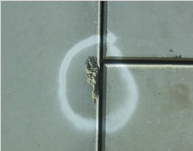
25.21 Panel damaged during erection.
