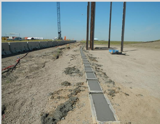
25.3 Levelling pad poured.
