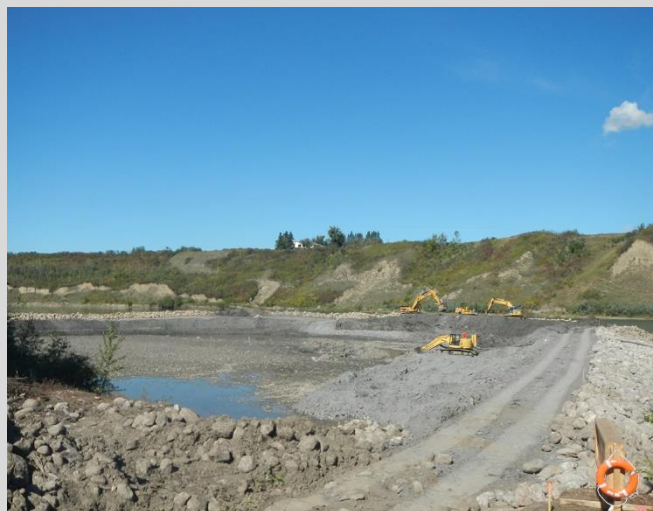
1.8 Berm construction and infill work. Pumping water from work area. Equipment access from top of berm.
