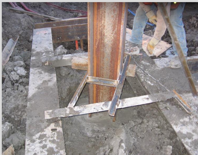
3.36 H-pile set into centre of concrete pile. Steel frame used to set location and elevation.
