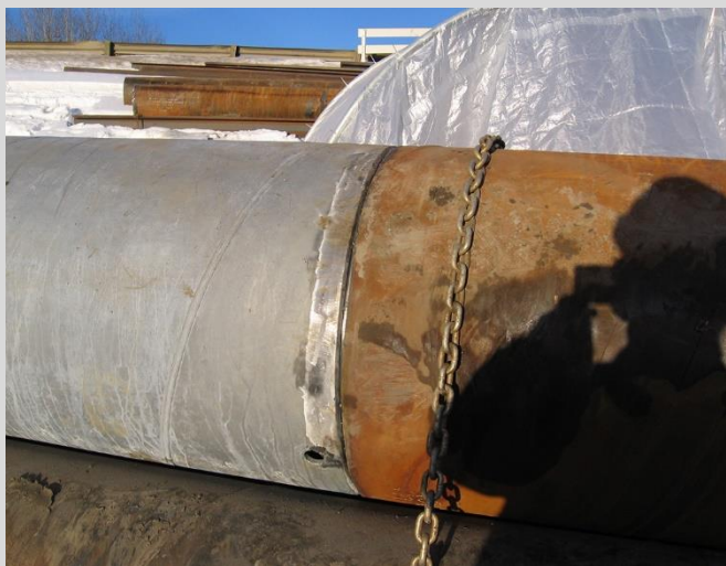
3.26 Splicing of galvanized and plain pipe piles. Galvanized pipe piles used above grade.
