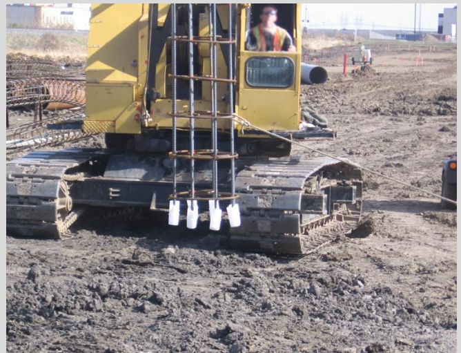
3.31 Plastic spacer chairs attached to bottom of reinforcing steel cage to prevent the cage from punching through the base of the excavation.
