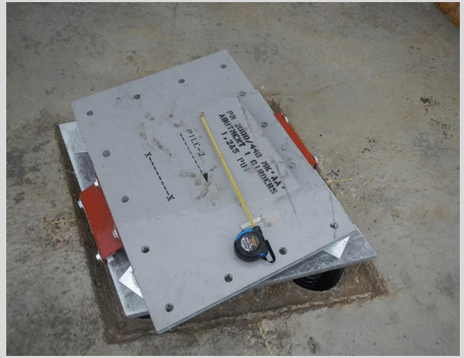
8.2 Longitudinal pot bearing on abutment seat. Erection hardware still in place to hold the bearing components together during transportation and installation.
