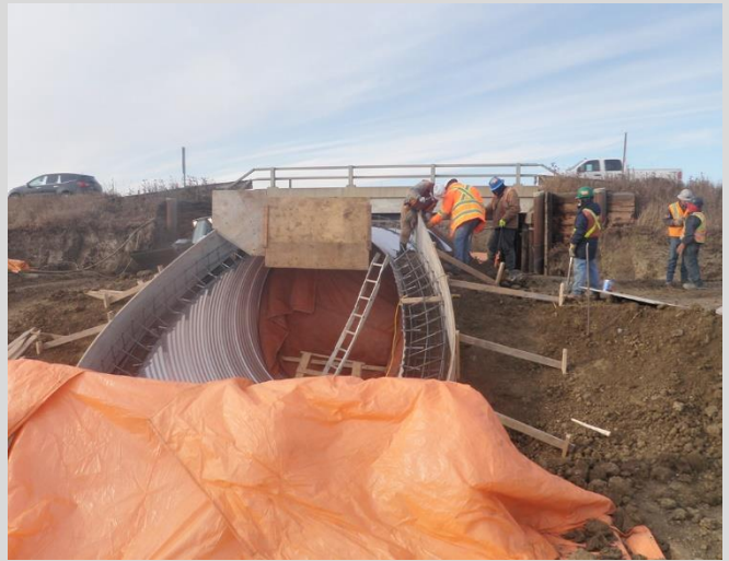
18.22 Concrete placement for collar.
