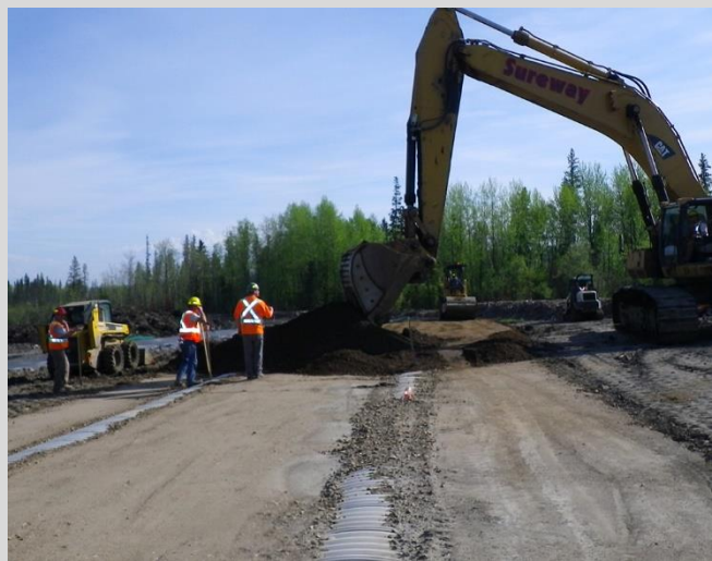
18.34 Completing backfill placement at crown of culverts.
