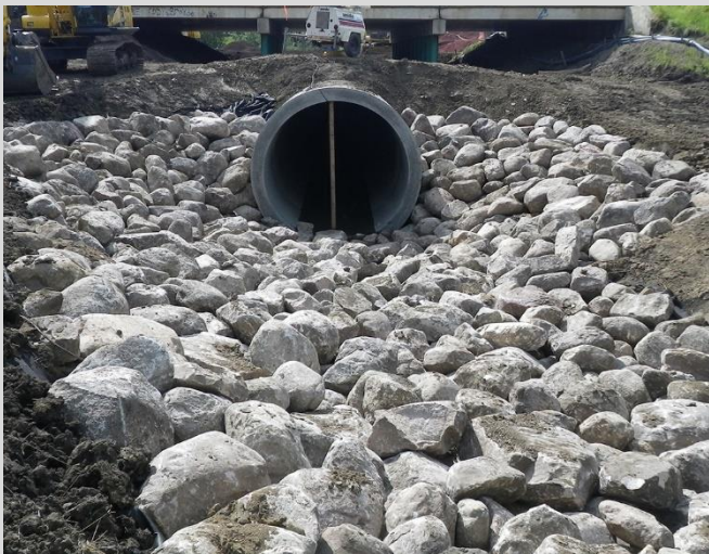
10.7 Riprap apron placed at RCP end.
