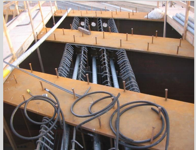
7.20 Post tensioning tendons in pier cap. Survey at every 1.0 m to confirm proper tendon profile.
