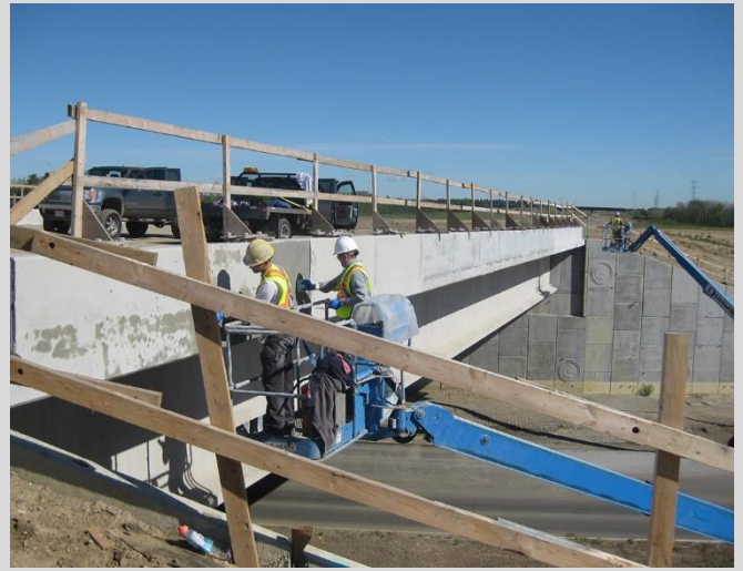
4.89 Concrete surface finishing at exterior faces of barriers. Workers using aerial work platform to access work. Class 2 rubbed surface finish followed by two applications of pigmented sealer.
