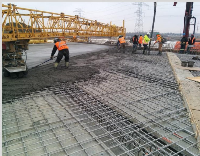
4.55 Bridge deck pour. Screeding closely following placement. Workers avoiding walking on screeded concrete.
