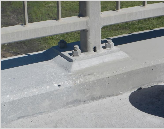
12.8 Completed pedestrian rail grout pad.
