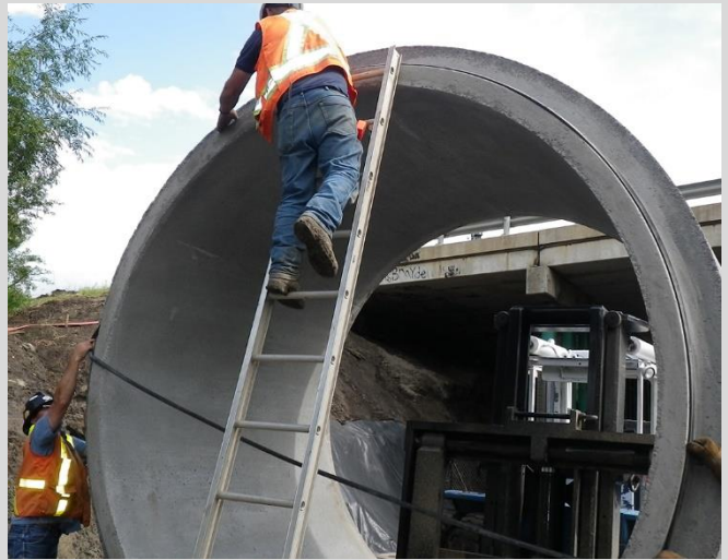
26.6 Gasket placed at spigot end of pipe.
