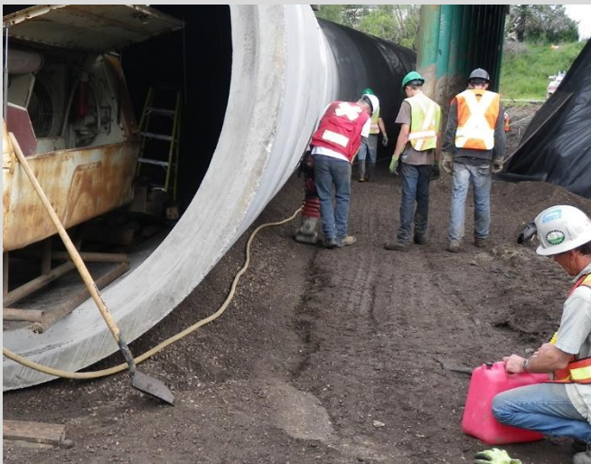
26.11 Compacting haunch area with a rammer.
