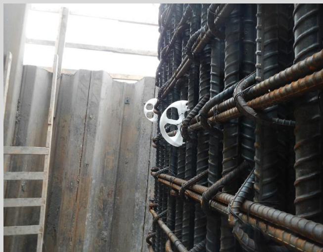
5.8 Pier shaft plain reinforcing steel. Wagon wheel chairs attached.
