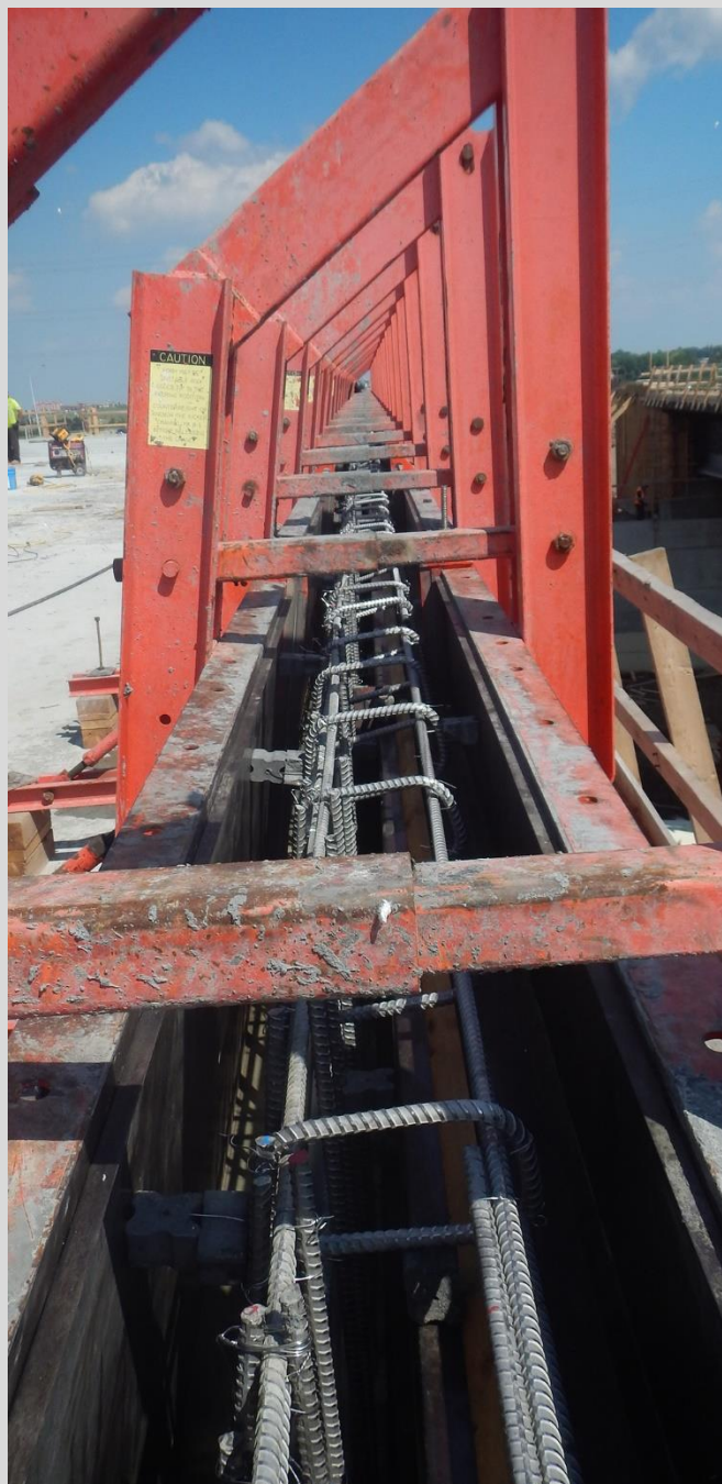
4.86 Re-usable steel forms for barriers.
