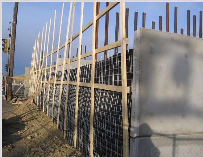
25.14 Two stage wall construction. Backfilling against wire wall. Fascia panels not in contact with fill.
