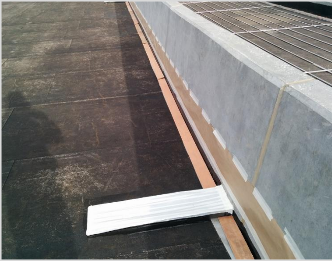
17.1 Protection of deck drain and barriers prior to tack coat and ACP placement.
