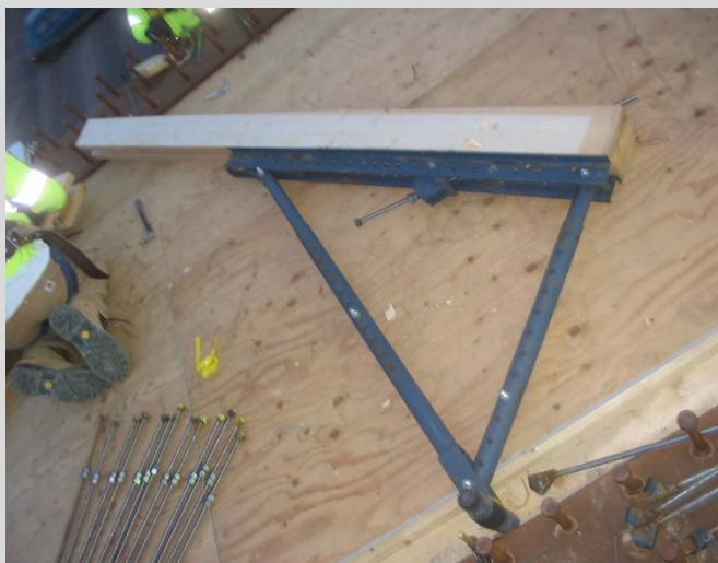
4.43 Adjustable deck overhang brackets.
