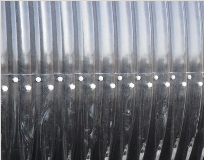
18.7 SPCSP showing that bolts in the valley of each longitudinal seam are nearer to the visible edge of the plate than the bolts in the crest.
