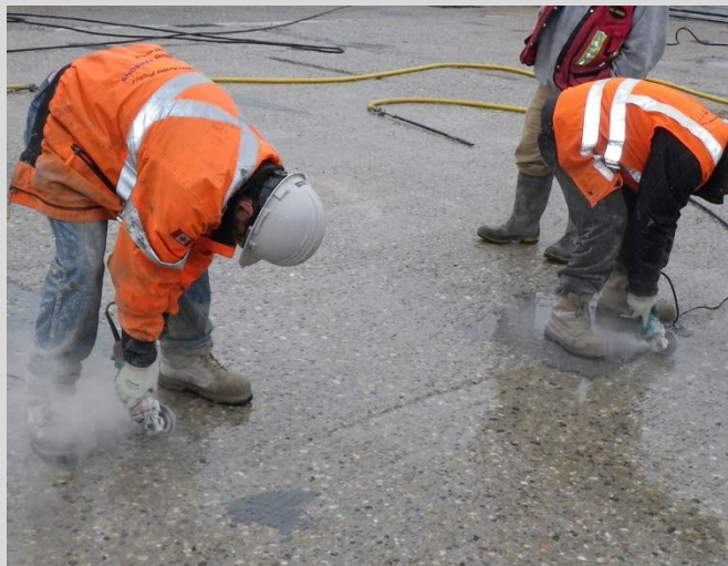
20.11 Workers routing cracks in preparation for epoxy.
