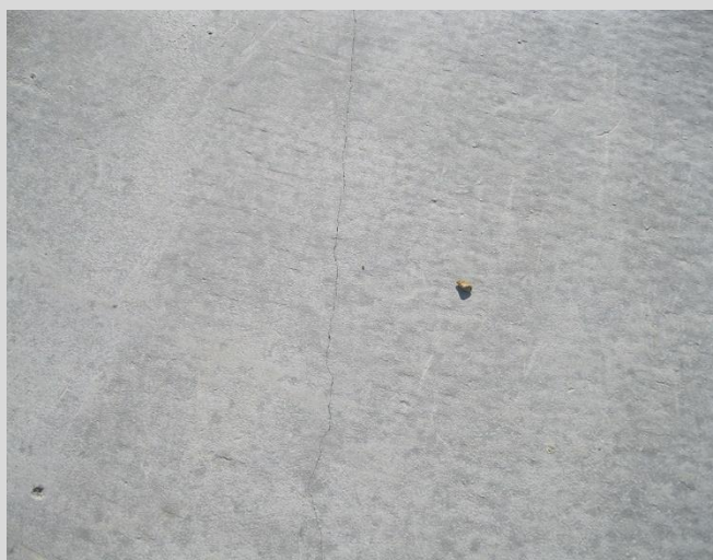
4.96 Transverse-direction deck slab drying shrinkage crack.
