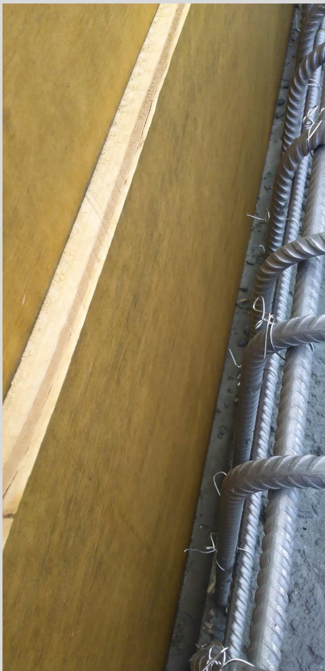
4.83 Typical formwork and pour strip at outside face of barrier. Note that forms are tight to the hardened concrete to prevent paste leakage.
