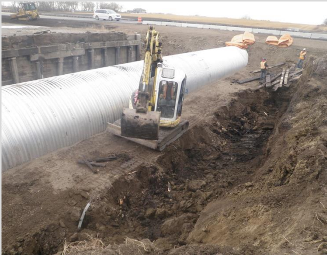
18.19 Removal of existing bridge structure. Abutment piles removed to specified depth below streambed.
