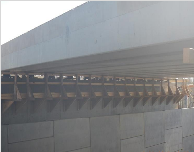
7.11 Completed erection of concrete box girders.
