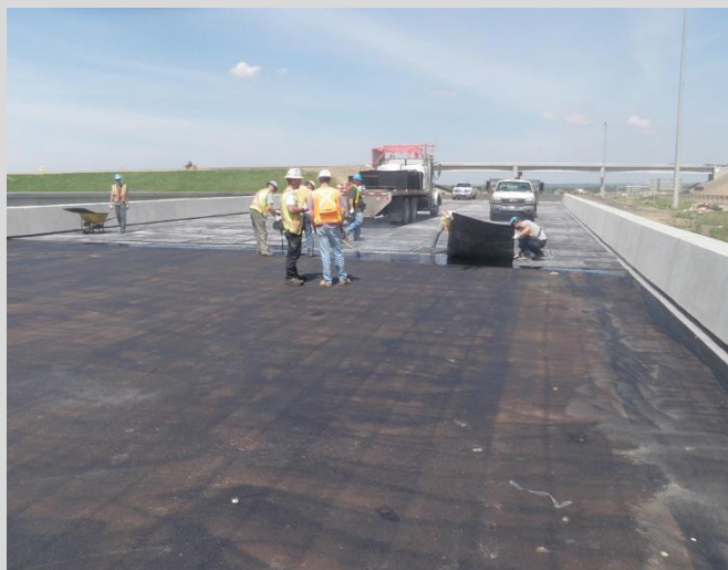
16.5 Tack coat on deck surface. Tack has changed from a dull black to a dull brown, indicating the tack coat has cured and is ready for the next stage.
