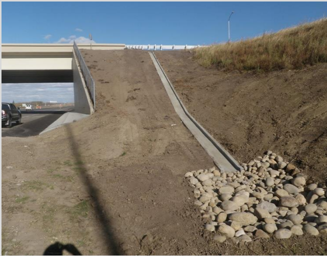
9.1 Riprap drain trough terminal protection.
