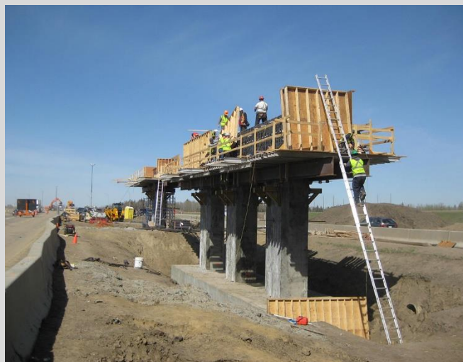
4.4 Pier cap formwork being erected.
