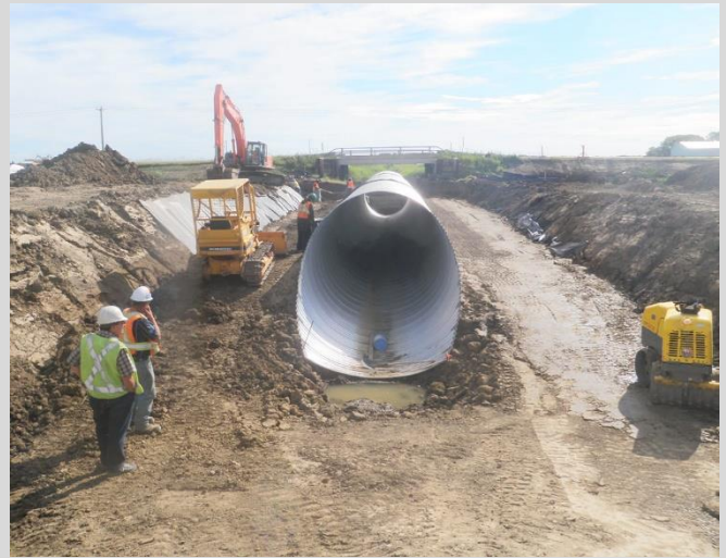
2.10 Backfill placed at culvert haunches.
