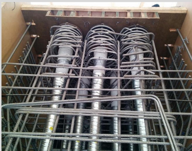
7.21 Post tensioning duct anchors in straddle bent. Congested reinforcing steel at pier cap ends.
