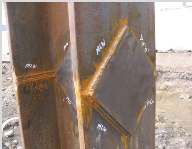
13.3 Completed H-pile splice plate detail.
