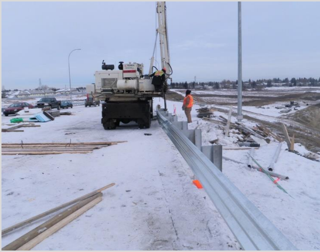
14.9 Post installation drilling.
