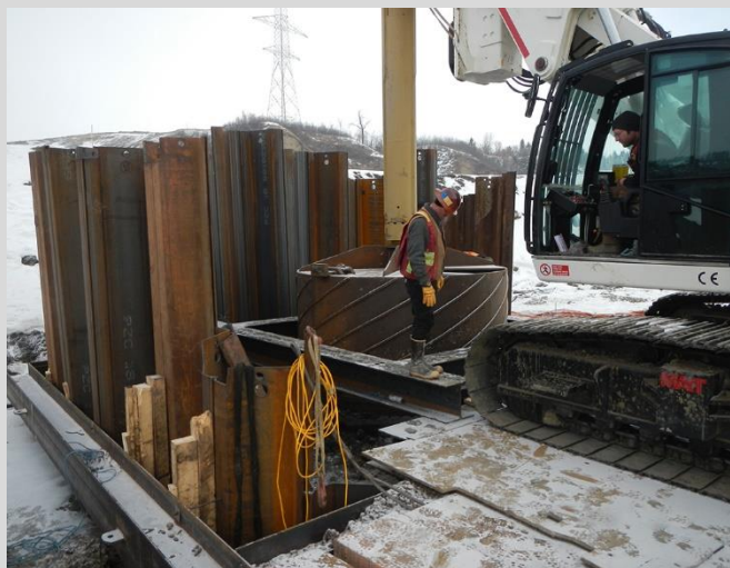
3.38 Large 3.0 m diameter pile. Muck bucket attached.
