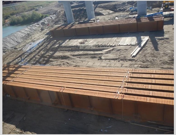
6.2 Girders stored at bridge site. Storage of girders is on timber dunnage and free-draining ground.
