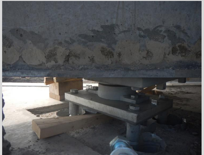
8.15 Pot bearing assembly. Once the girder is set in place, the wooden wedges are no longer needed.
