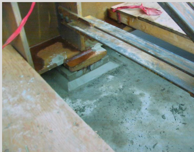
8.20 Grout pad constructed at 45 degree slope from abutment seat to bottom of base plate.
