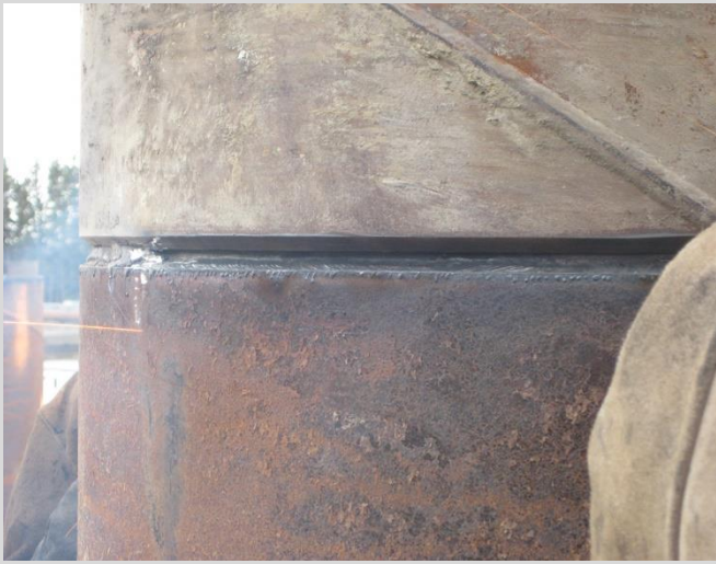
13.5 Pipe pile splice ready for field welding.
