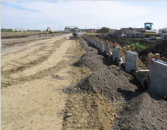
25.11 Two types of backfill material placed. Drainage layer backfill material placed within 1.5m of back face of wall.
