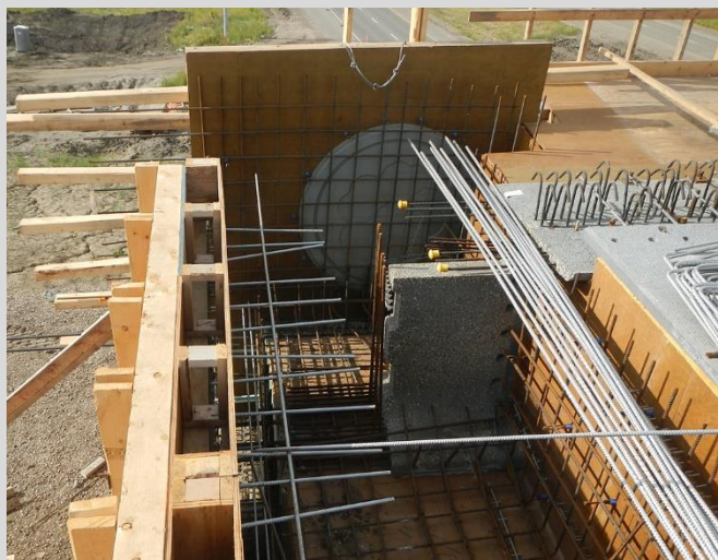
4.10 Abutment diaphragm formwork and reinforcing steel. Aesthetic enhancement motif cast into exterior face of diaphragm.
