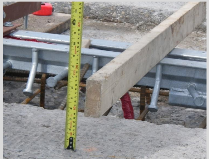
20.16 Checking deck joint elevation.
