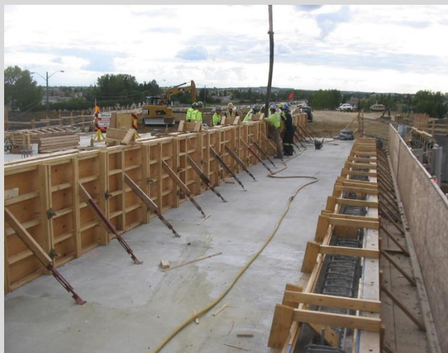
4.82 Wooden forms for barrier and curb formwork. Form attachment to deck concrete must be avoided.
