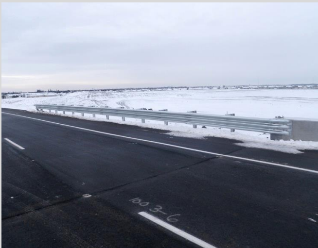
14.7 Guardrail and posts with end treatment.
