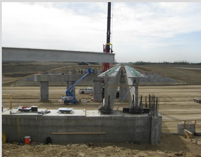
7.3 First girders erected and stabilized with temporary shoring and bracing. Short H-pile section bolted to the abutment to provide additional lateral stability at the bearing.
