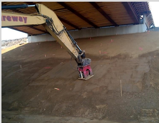
4.107 Headslope compaction with hydraulic excavator.
