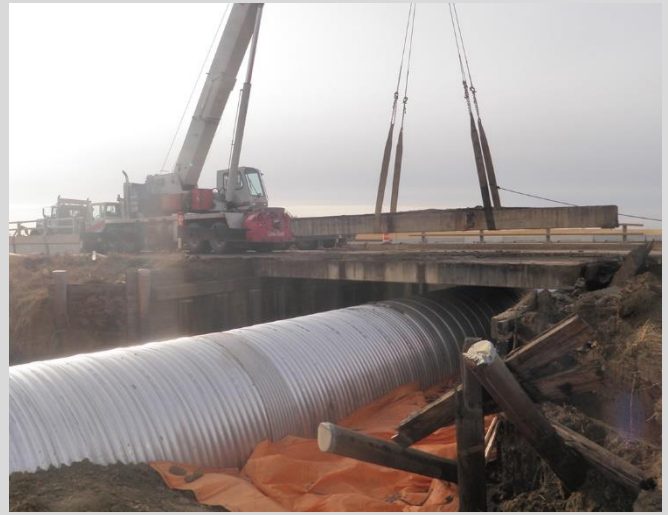
18.18 Removal of existing bridge structure.
