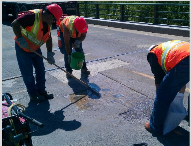
15.7 1st polymer layer placement seeded with aggregate.
