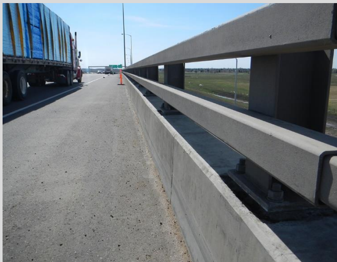
12.2 Bridgerail alignment and elevation adjusted prior to grouting. Alignment and elevation to required lines is important for overall functionality and appearance of the bridgerail.
