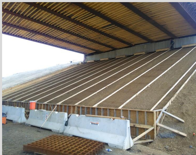
4.110 Forming of vertical concrete slope protection courses.
