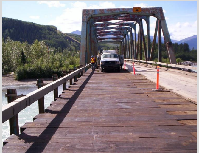
23.2 Strip deck partially removed.
