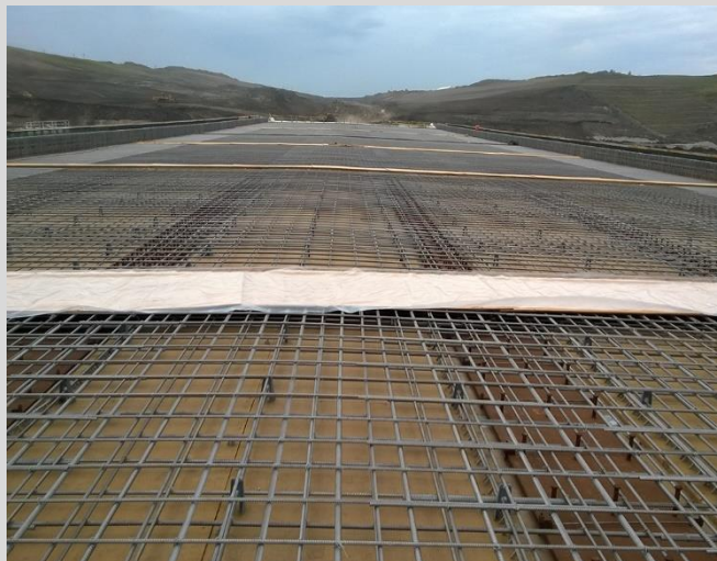
4.46 Deck reinforcing steel installed, tied, and chaired. Bulkheads constructed at planned termination of deck placement sections.
