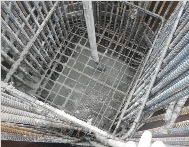
3.42 Concrete discharge down centre of pile by pump. Pump hose centred so that concrete does not impact reinforcing steel.
