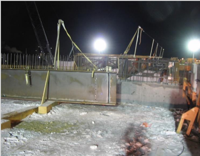
6.24 Fall protection system consisting of uprights and cables used during girder erection and deck overhang bracket installation.
