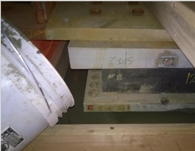
8.10 Placing grout.
