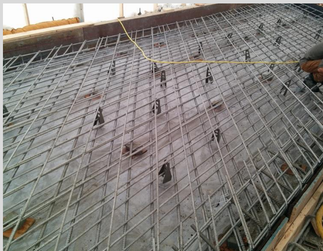
4.73 Approach slab reinforcing steel. Plastic chairs used to separate reinforcing mats. Reinforcing steel placed on skew with deck.
