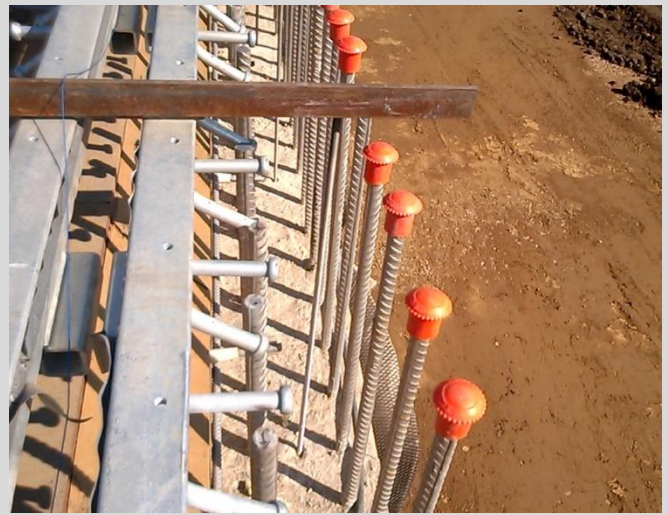
6.17 Abutment side coil rod supports shown.
