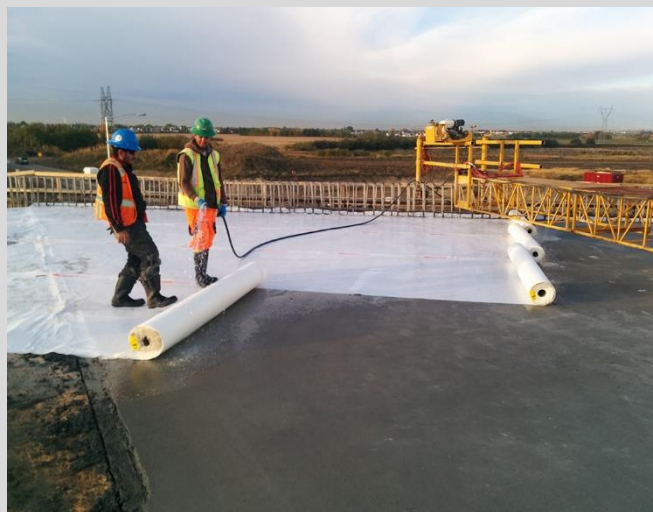
4.68 Once the concrete will not be marred, crews apply pre-soaked curing fabric.
