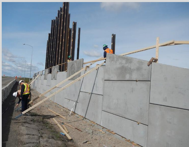
25.7 Panels set at batter. Turnbuckle on bracing used to set batter. Panels clamped together at edges to maintain alignment.
