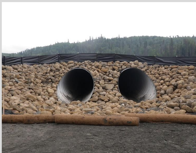
18.35 Completed culvert outlet.
