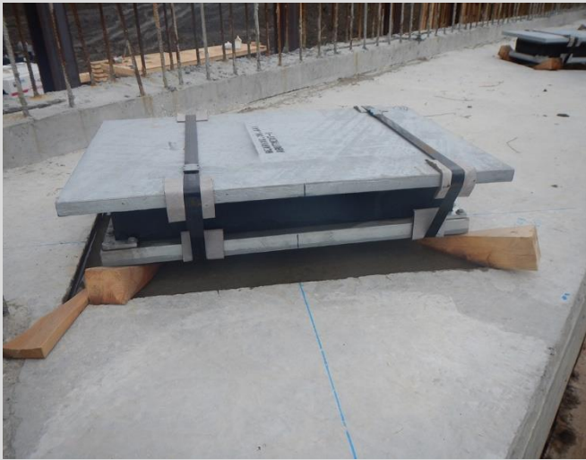
8.5 Bearing assembly centred and blocked in position.
