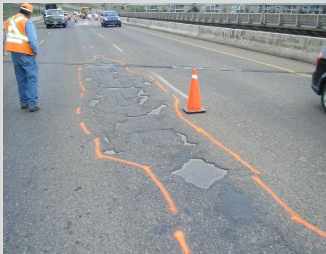
15.1 Repair area for polymer wearing surface identified.
