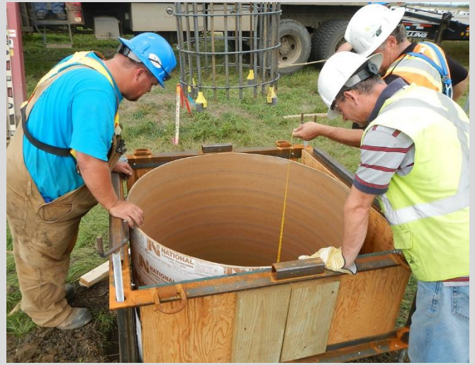
24.2 Checking depth of pile.
