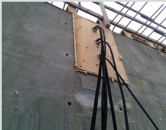
7.33 Diaphragm end ready for grout. Blockout formwork is sealed to prevent grout leakage.
