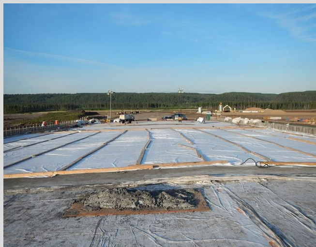
4.70 Dunnage is used to secure filter fabric.
