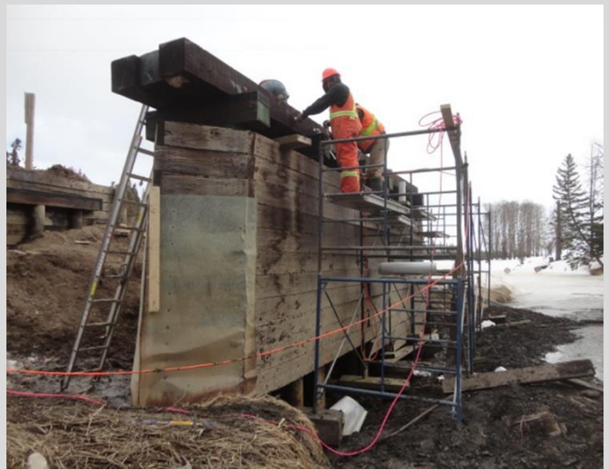
23.6 Treated timber pier cap replacement.
