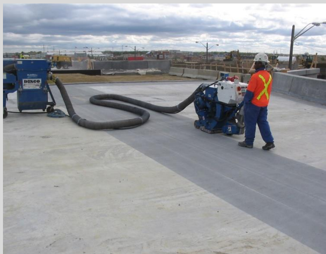
16.1 Deck surface preparation by shot-blasting.
