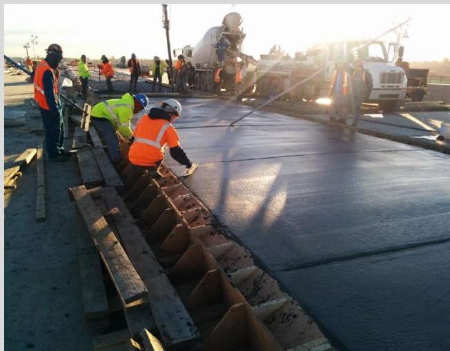
4.87 Crews tooling joints at 3.0 m spacing. Broom finish to be applied.
