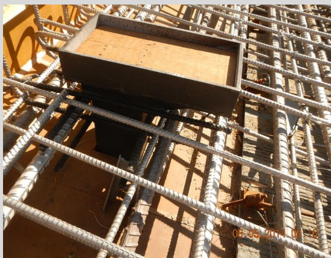
13.1 Polyurethane coated and galvanized deck drain.
