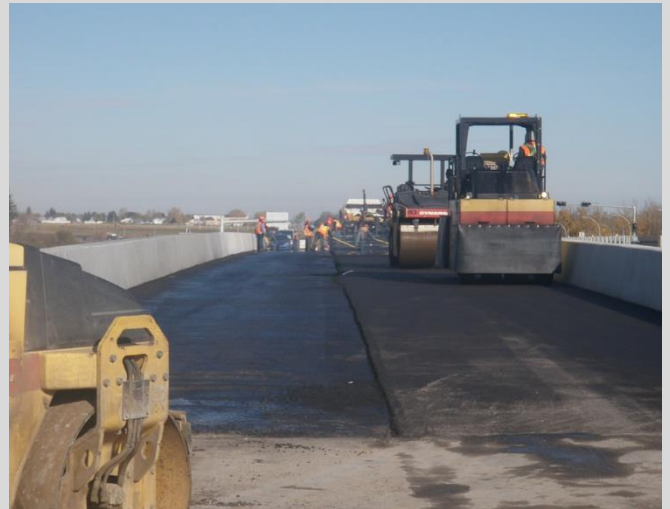
17.8 Longitudinal joint shown. Compaction equipment must be capable of travelling immediately adjacent to curbs, barriers and median as required.
