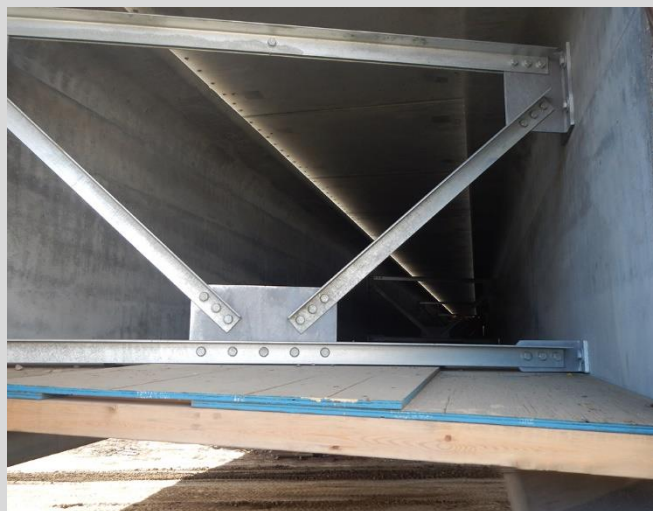
7.16 Galvanized diaphragm cross bracing installed. False deck used as a work platform.
