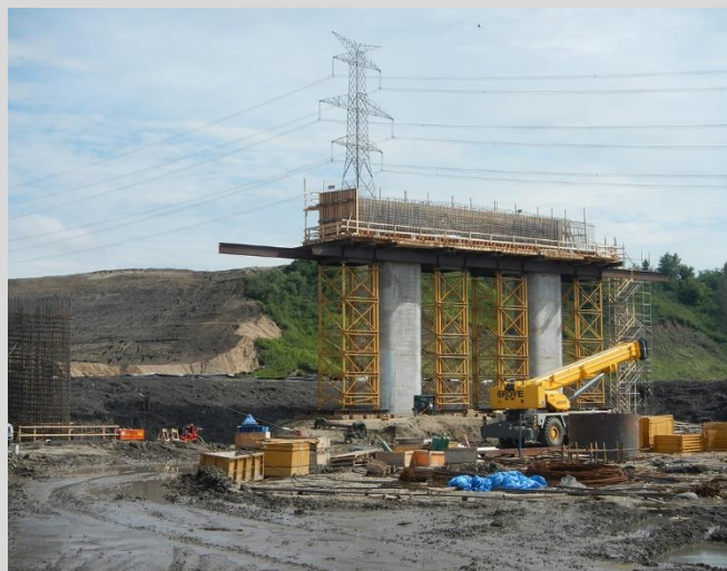
4.15 Pier cap shoring towers and scaffolding.
