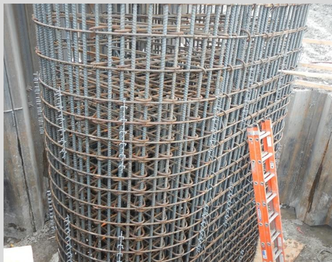
5.6 Pier column plain reinforcing steel.
