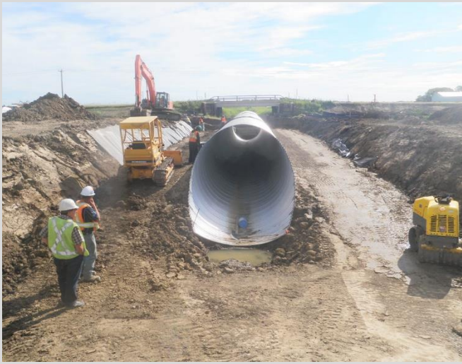
18.17 Backfill being placed at haunches.
