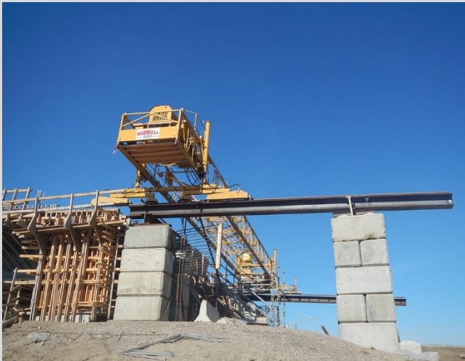
4.53 Deck finishing machine run-off rails.
