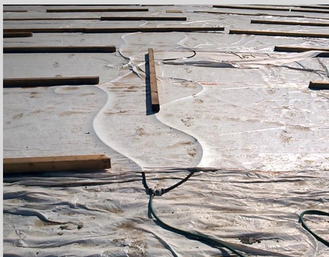
4.71 Soaker hoses are used at the crown to maintain wet filter fabric throughout the curing period.
