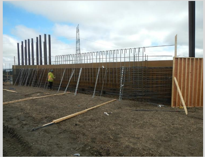
5.2 Abutment seat formwork and plain reinforcing steel.
