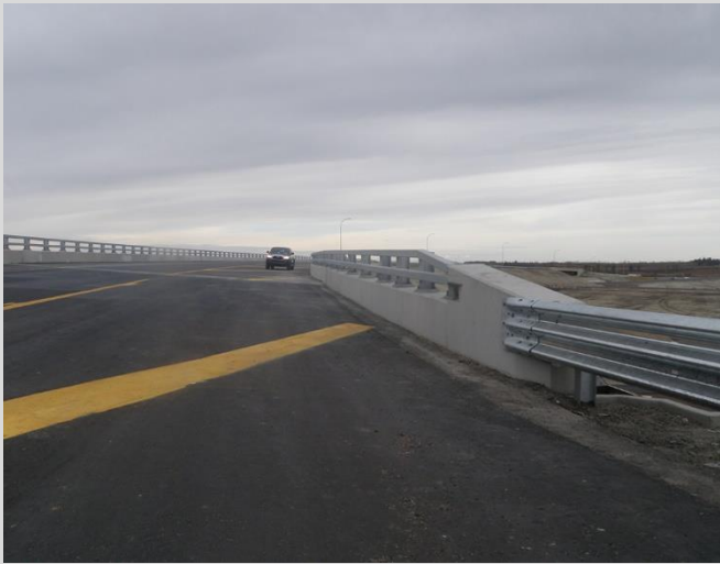
14.1 Guardrail to bridgerail transition.
