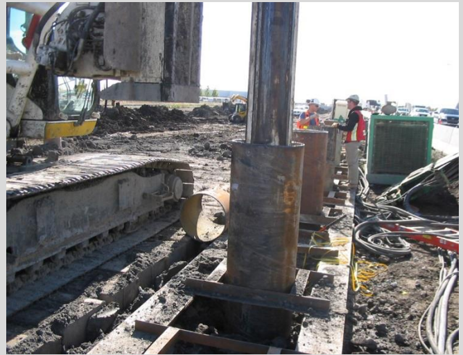
3.21 Drilling pile holes with casing installed. Casing is used temporarily to keep the excavation from caving in, or to stop seepage. Casing is removed during concrete placement.
