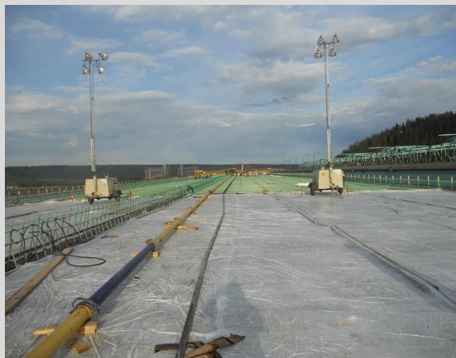
4.64 Line pump used to place deck concrete.
