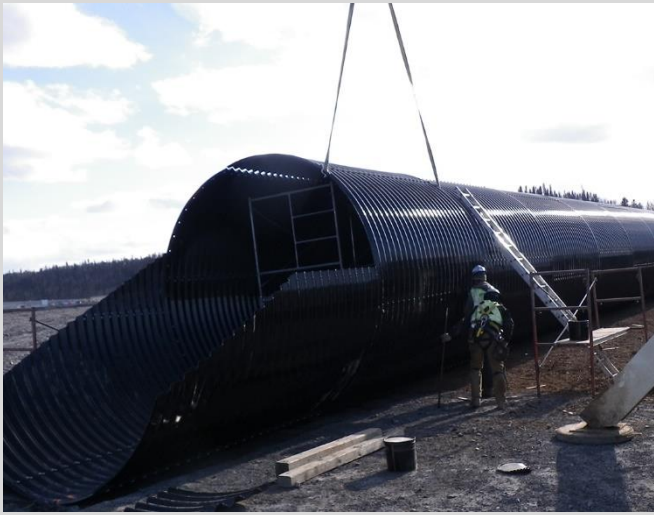
18.5 Assembling SPCSP culvert.
