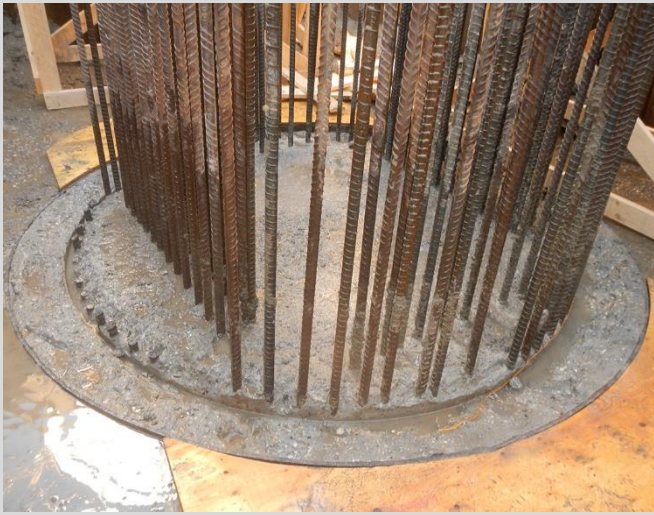
3.44 Construction joint at pile top.
