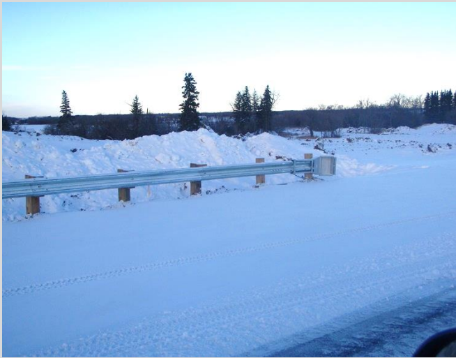
14.5 Guardrail and posts with end treatment.
