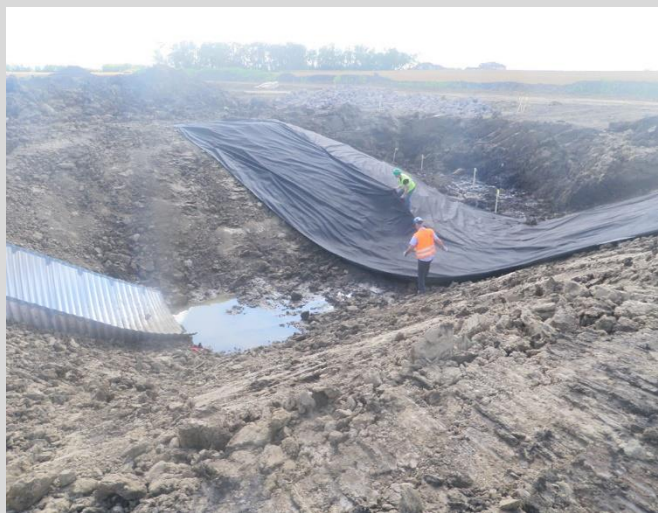
10.3 Crews placing filter fabric material prior to heavy rock riprap placement. Filter fabric keyed into top of slope.
