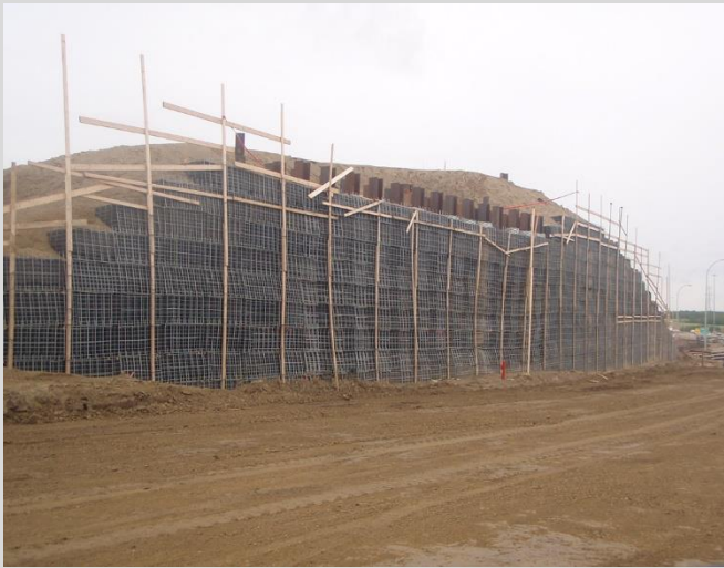
25.27 Wire wall completed at two stage wall.
