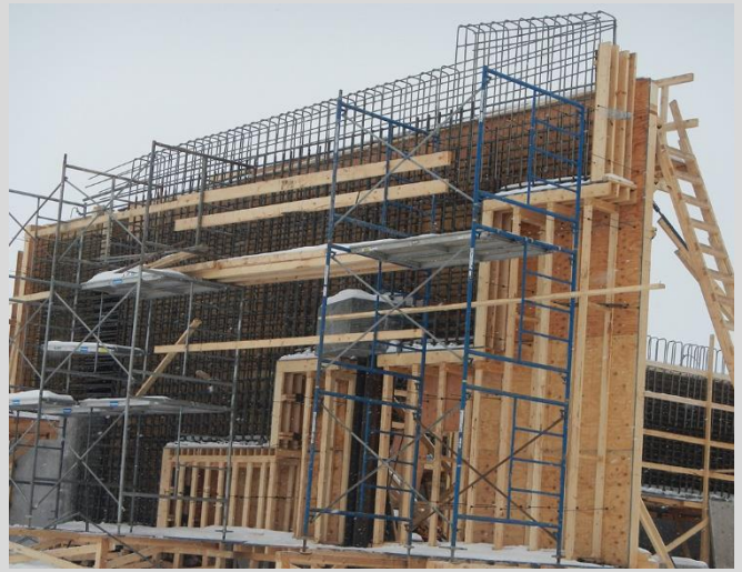
4.5 Partial wingwall formwork.
