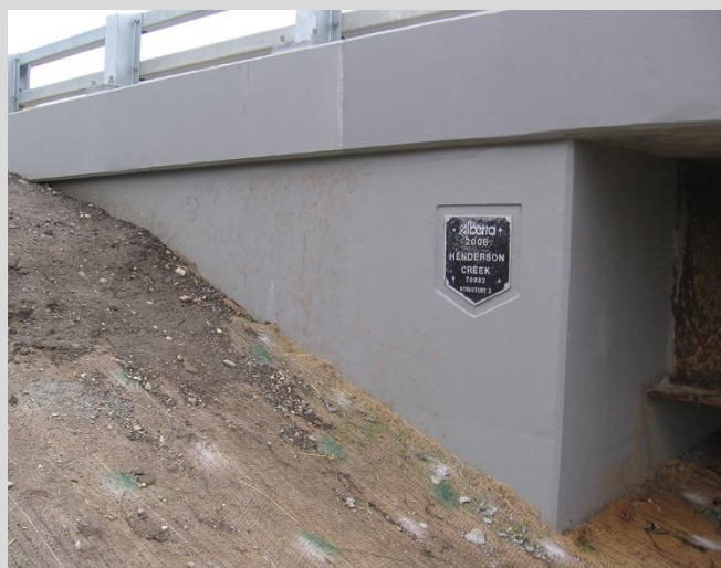
13.2 Cast-in-place bridge plaque. Bridge plaques must be set true to wingwall and barrier lines.
