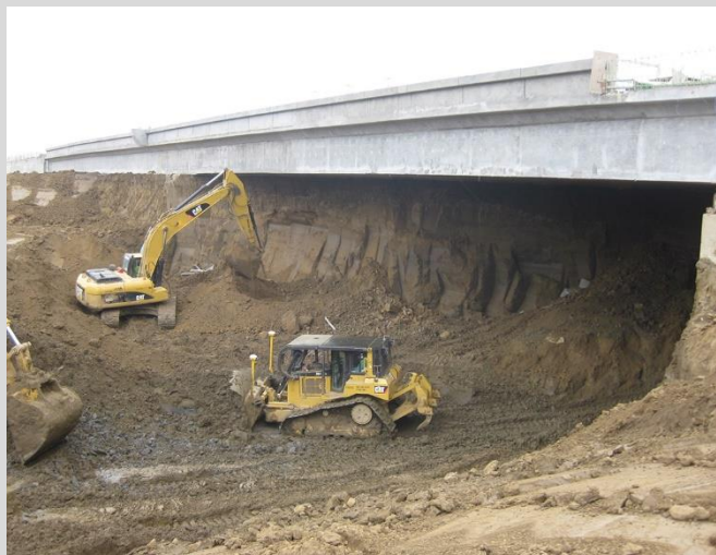
1.10 Cast-in-place concrete bridge constructed on existing grade. Excavation of roadway beneath, after superstructure is cast.
