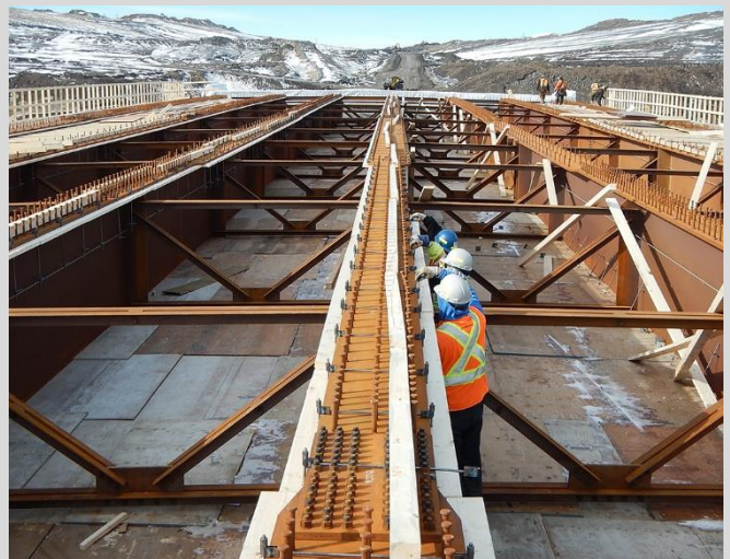
4.34 Timber deck formwork is typically hung from coil bolt hangers supported on girder top flanges. False deck working surface shown.
