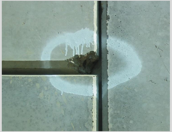
25.20 Panel damaged during erection.
