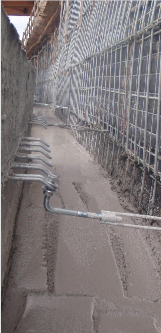
25.30 Space between 1 st and 2 nd stage. Panel anchorages shown.
