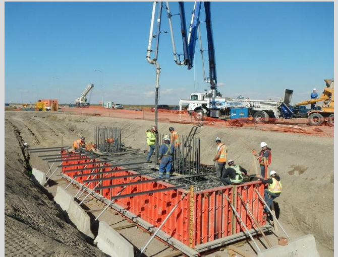
4.19 Concrete pump used for pile cap pour. Forms braced against precast concrete deadmen.
