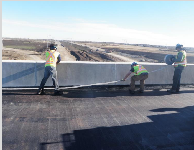
16.7 Wick drain placement along edges of barriers. Wick drains are installed over the asphalt membrane while it is still tacky. Protection boards are not placed over wick drains.
