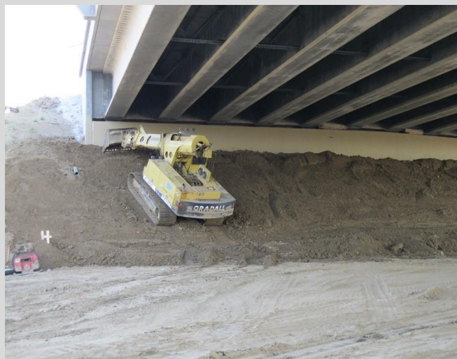
4.106 Preparation of headslope with telescoping boom excavator.
