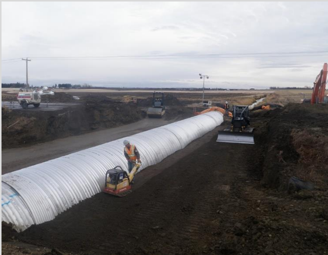
18.23 Compaction of granular backfill material.
