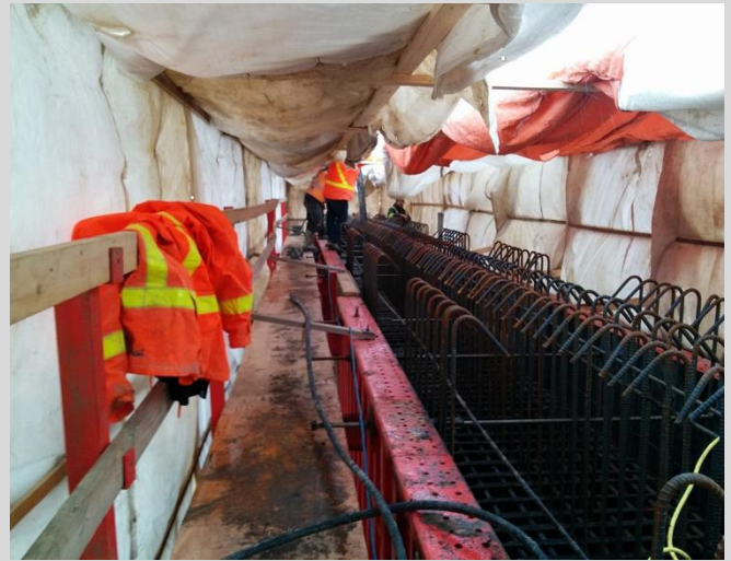
4.32 Cold weather concreting. Hoarding for pier cap pour. Room for workers and equipment to work within the enclosure. Roof tarps open to allow for concrete pump access.
