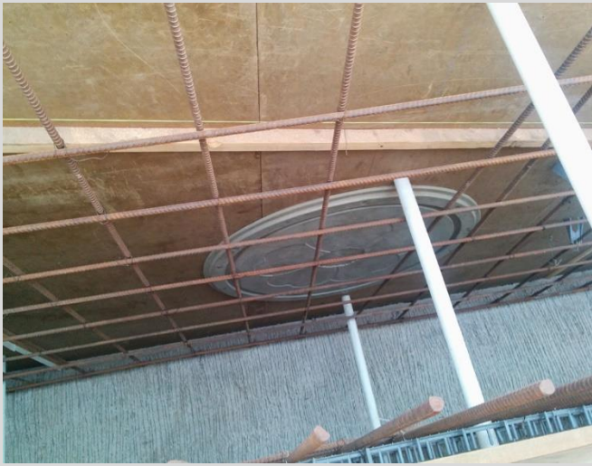
4.16 Wingwall formwork and plain steel reinforcement. Aesthetic enhancement motif cast into exterior face of wingwall.
