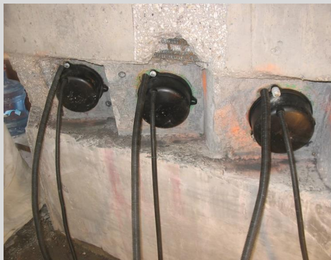
7.29 Tendons cut and capped, ready for grouting. Grout flow tubes protruding from cap.
