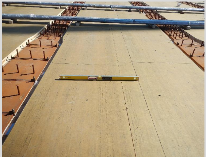
4.38 Prior to installation of reinforcing steel, it is important to check form cross-fall to confirm form position accuracy.
