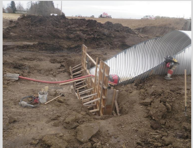
18.20 Formwork for cast-in-place collar cut-off wall.
