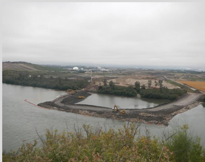
1.6 River berm construction. Perimeter placed first to isolate the work area. Riprap being placed for scour control.
