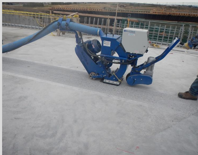
16.2 Deck surface preparation by shot-blasting.
