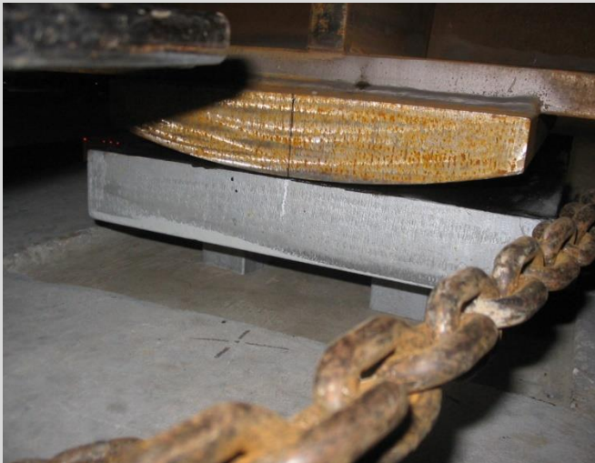
8.3 Rocker bearing. Centre line of bearing marked on masonry plate, rocker plate and top of pier. Grout pad recess smooth and providing an even bearing on the shim stacks.
