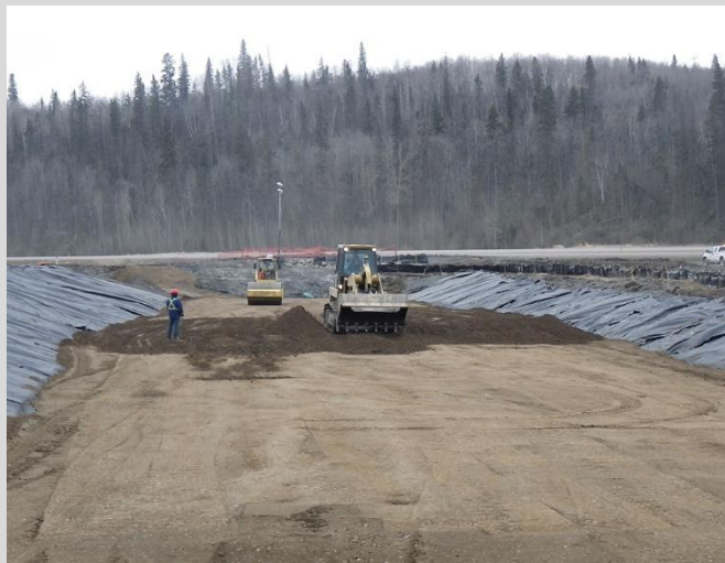
18.27 Backfilling at culvert bed.
