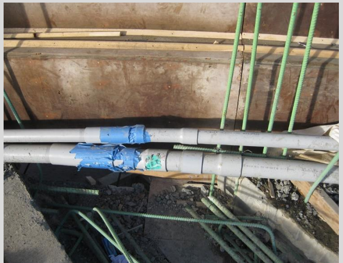
11.8 Poorly aligned connection at expansion joint.
