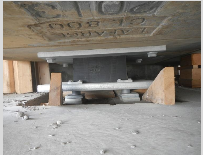
8.4 Reinforced elastomeric bearing pad. Wooden wedges and pintles to set masonry plate level.
