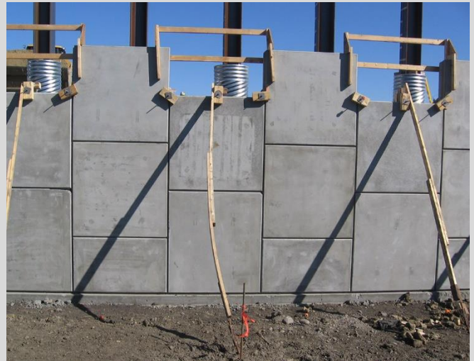
25.12 Adjustment of wall batter using turnbuckles.
