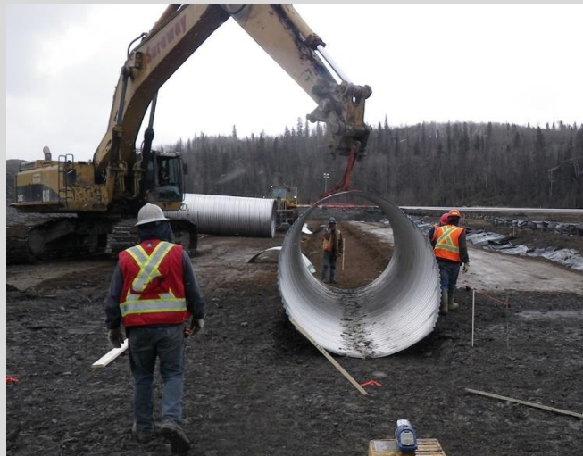
18.28 Installation of CSP structure at pre-shaped bed.
