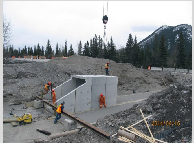
26.18 Winching of PBC unit into position.
