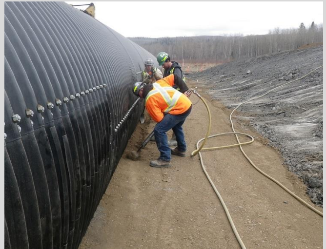
18.8 Compacting haunch area with pogo stick. Shovels and small equipment are also used to fill all corrugations.
