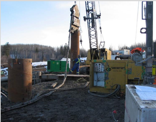
3.22 Vibratory hammer used to advance drilling casing. Worker checking if casing is plumb.
