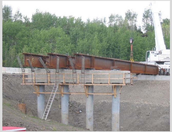
3.45 Galvanized pipe piles at exposed pier columns.
