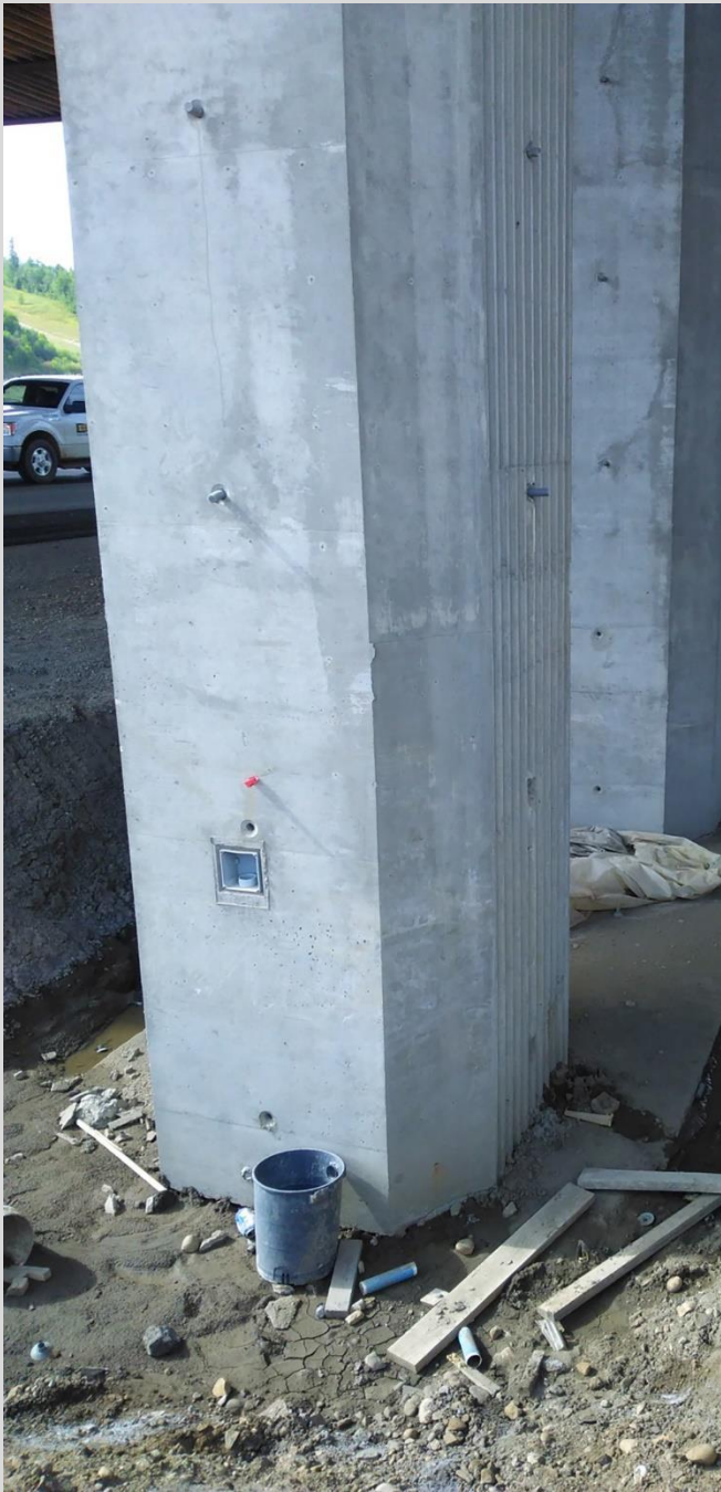
4.6 Mudslab shown at pier columns.
