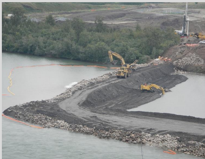
1.7 River berm construction. Infill material and riprap being placed, pumping out water from work area.
