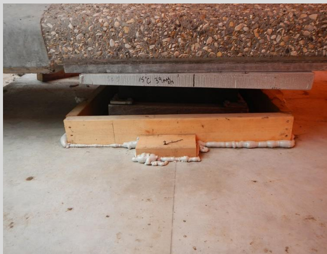
8.21 Bearing pad form work for grouting.
