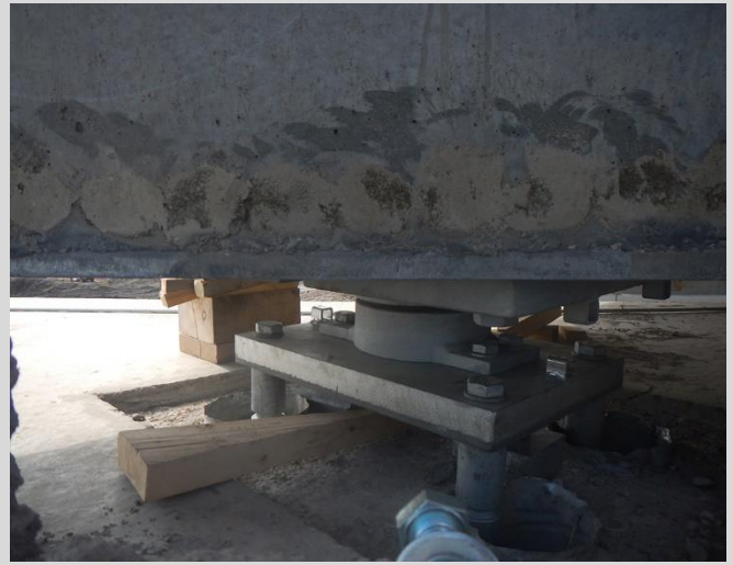
7.10 Concrete box girder on pot bearing.
