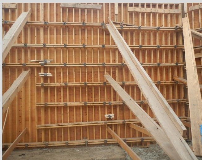
4.9 Formwork and bracing for wingwall. Full sheets of plywood used to reduce form lines.
