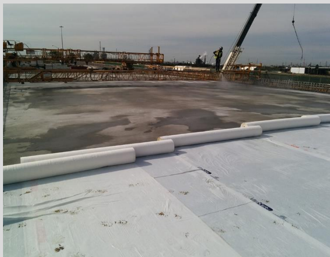
4.67 Crews applying pre-soaked curing fabric.
