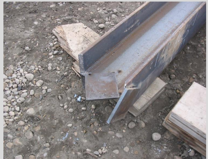
3.8 H-pile splice detail. Splice plates are welded to the pile extension, the pile is stacked on the previously driven pile, and the extension is then welded to the pile.
