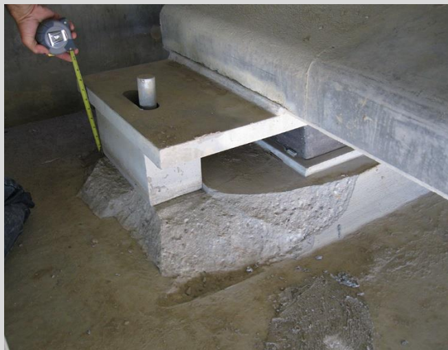
8.18 Damage to grout pad due to improperly set bearing.
