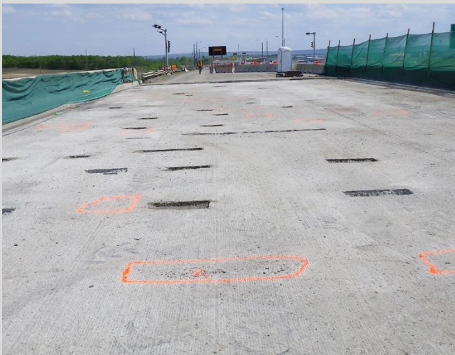
20.3 Partial or full depth repair areas prepared.
