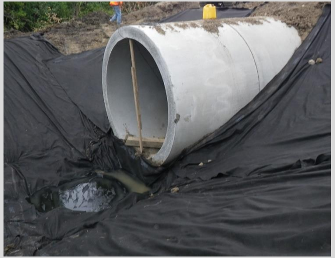
10.6 Filter fabric placed around end of RCP.
