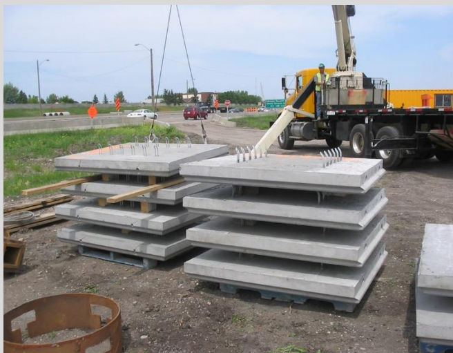
25.25 Storage of fascia panels onsite. Panels should be stacked neatly with blocking between panels.
