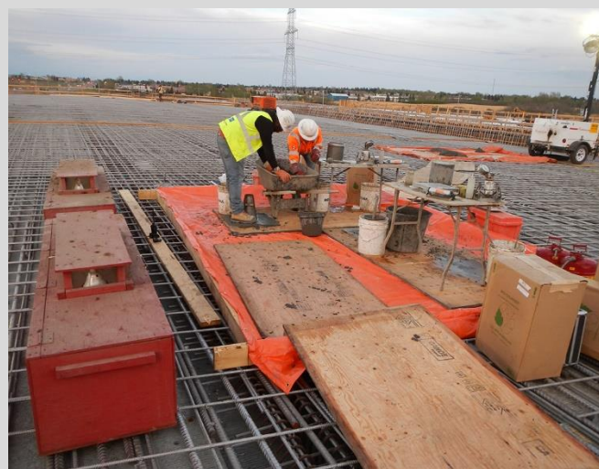
4.58 Concrete testing station set up on deck.
