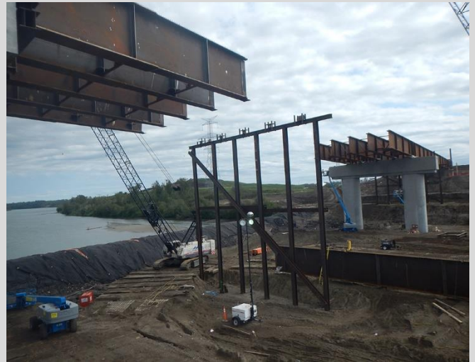
6.4 Girder erection. H-pile shoring towers used to support girders at splice connection between girder segments.
