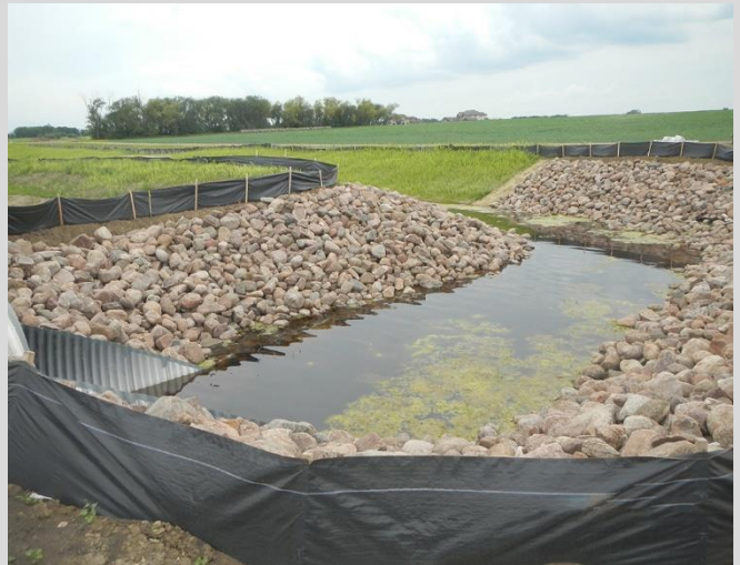
18.24 Completed culvert outlet.
