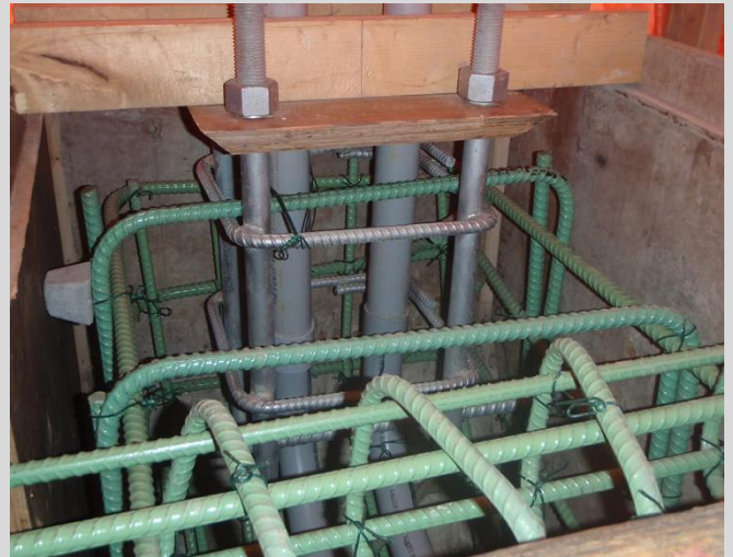
11.4 Ducts in barrier for overhead lighting.
