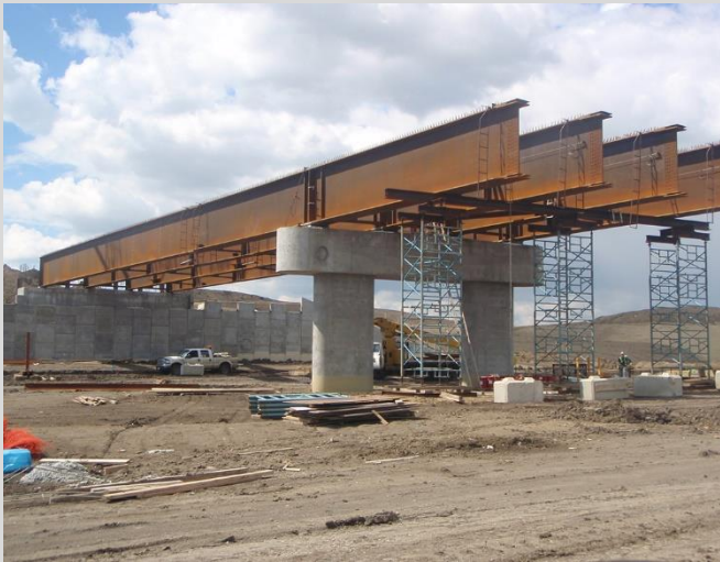
6.3 Girder erection. Scaffolding shoring towers used at splice connection between girder segments.
