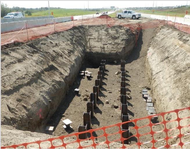
1.1 Pier excavation for pile cap. Piles cut off at elevation. Safe slopes and good access to excavation shown.
