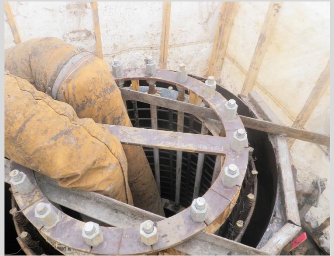
24.6 Anchor rod assembly installed. Angle iron on formwork to hold anchor rod assembly at correct elevation.
