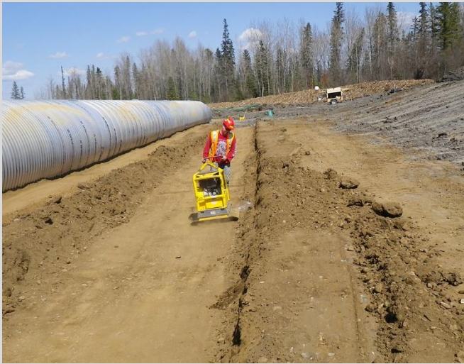
2.9 Compaction of bedding.
