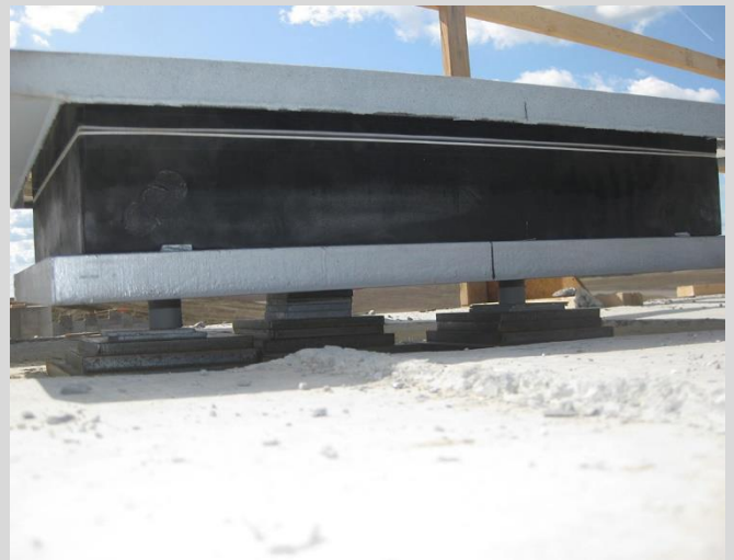
8.8 Bearing set to elevation.
