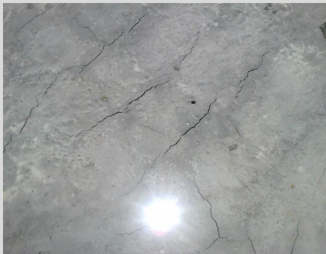
4.98 Plastic shrinkage cracks on deck slab surfaces.
