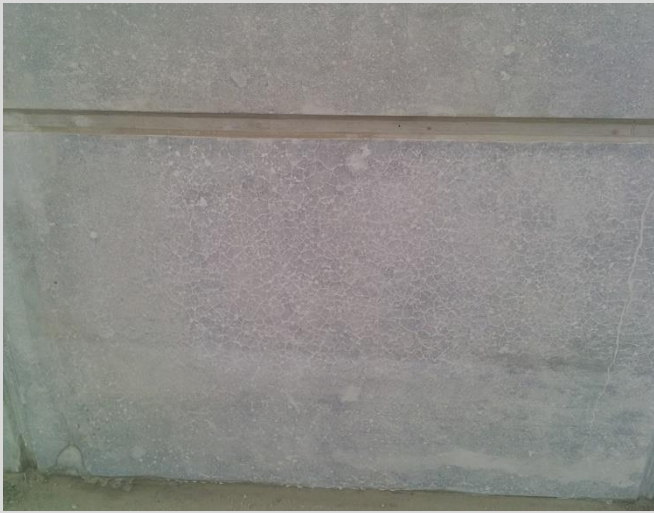
4.101 Crazing -type cracking seen on formed surfaces.
