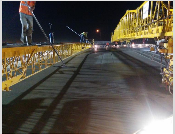
4.60 Concrete finishers bull floating concrete deck immediately after screeding. Finishing done from work bridges.
