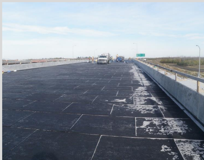
16.12 Waterproofing complete. Clean up of sand and debris from protection board required before tack coat for ACP. Joints and laps in protection boards shown.
