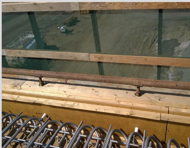
4.47 Finishing machine screed rail cups are installed and rail is set by instrument to the design gradeline.
