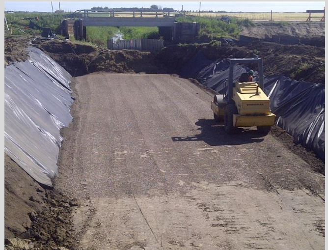
2.8 Smooth-drum roller compacting culvert bedding material. Geotextile and safe side slopes shown.
