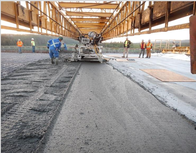
4.61 It is important that concrete be screeded and raked before consolidation. Workers must not walk through or place additional concrete at locations where vibration has already taken place.
