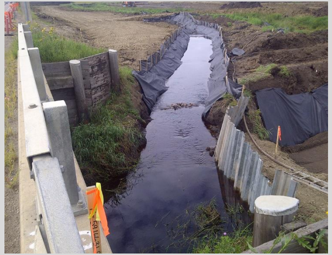
18.14 Temporary diversion for watercourse. Silt fence and filter fabric lining the temporary streambed.
