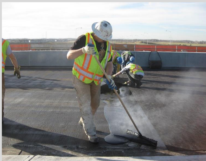
16.9 Asphalt membrane is poured from a pail and spread with a rubber squeegee.
