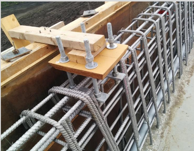
12.10 Anchor bolt assembly cast into barriers. Wooden blockouts form grout recesses. Bolt projection to be protected to prevent contamination from concrete during barrier placement.
