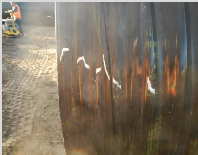
18.36 Damage to polymer coated CSP structure. Special adhesive tape or approved brush on coating is required.
