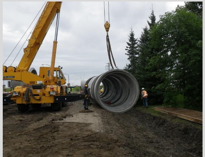
26.4 Crews unloading RCP. RCP lifted with slings from truck bed. Small swale dug at unloading area.
