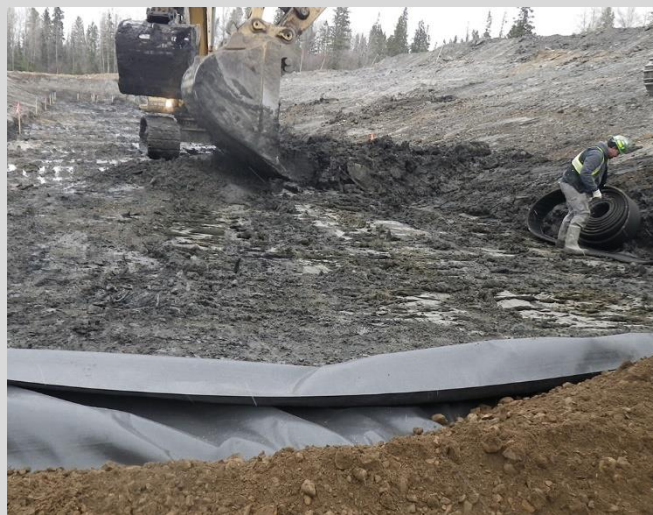
18.26 Soft conditions at culvert bed elevation.
