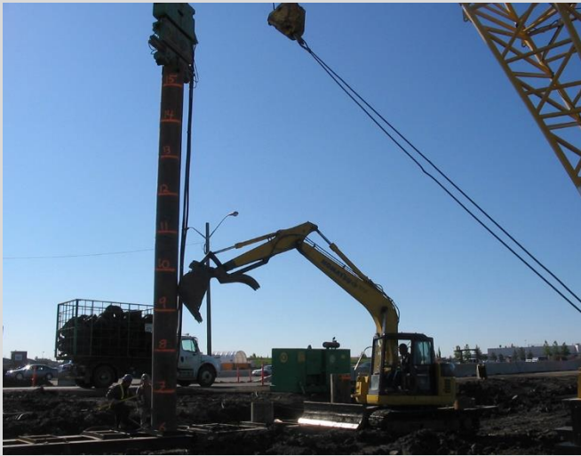
3.28 Vibratory hammer used to advance drilling casing.
