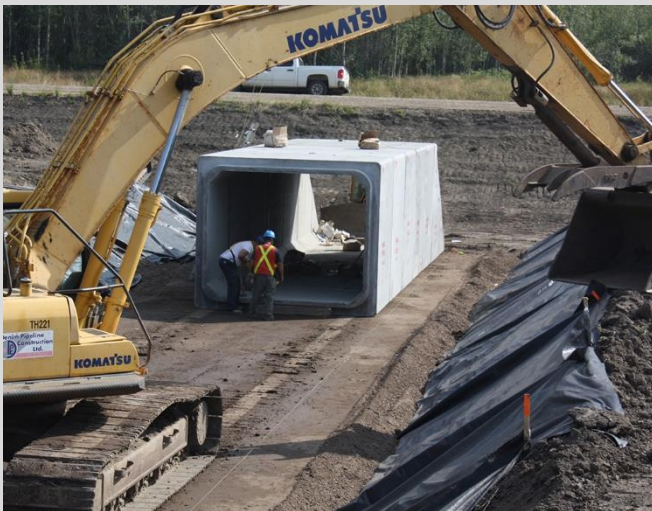
26.15 Installation of PBC units onto prepared bed, using string for alignment control.
