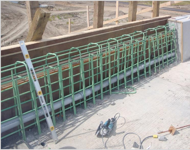
11.1 Duct for electrical conduit in barrier.
