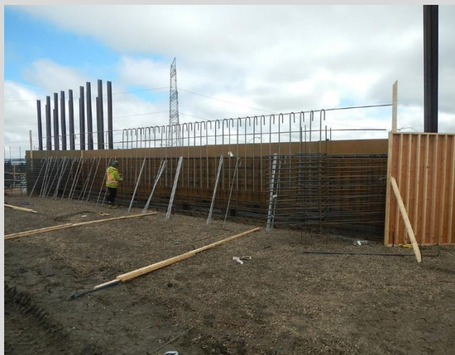
4.1 Abutment seat partial formwork and reinforcing steel.
