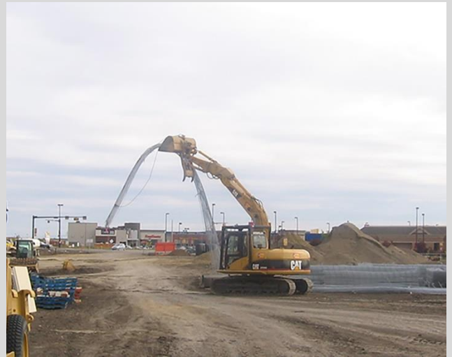
25.22 Poor handling of soil reinforcement. Fabric slings and spreader bar should be used.
