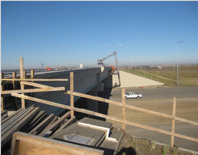
4.90 Concrete surface finishing of exterior faces of barriers. Workers using aerial lift truck to access work.
