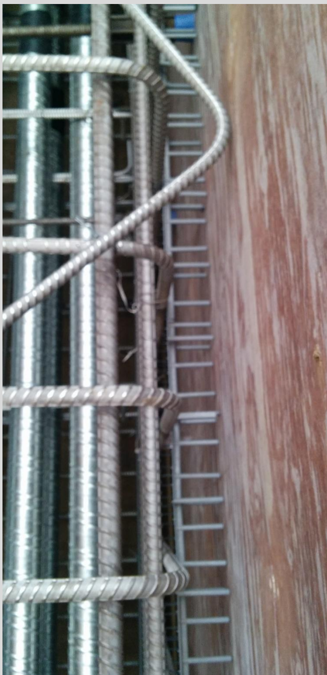
4.21 Plastic supports or chairs used to maintain required cover to edge of formwork.
