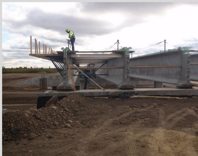
7.14 Installing deck overhangs and galvanized cross bracing. Fall protection system is in place.
