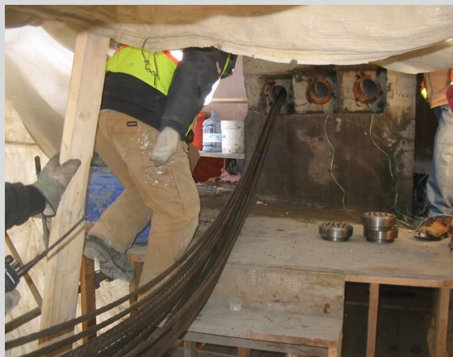
7.25 Tendons pulled through post-tensioning ducts.
