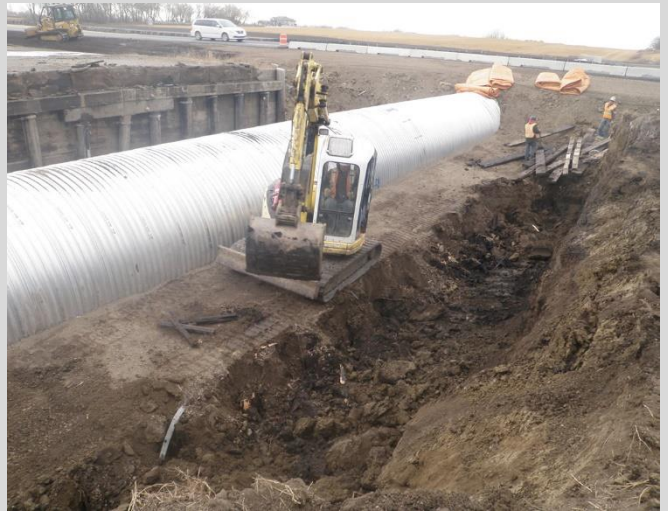
21.4 Demolition of substructure. Piles are removed or cut to specified elevation below streambed.
