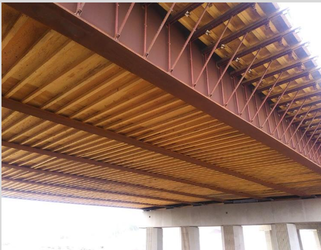
4.33 A false deck is typically constructed at the lower flanges to provide a working surface.
