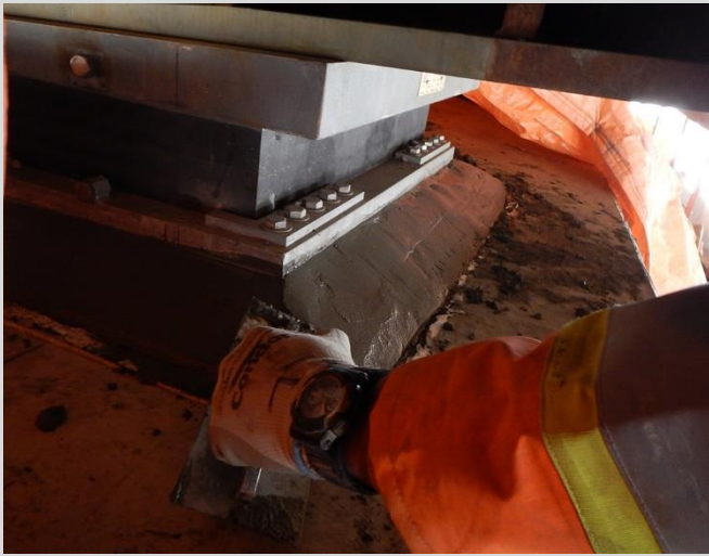
8.12 Trimming grout after form removal. Note that top of grout pad elevation is not higher than the underside of masonry plate elevation.
