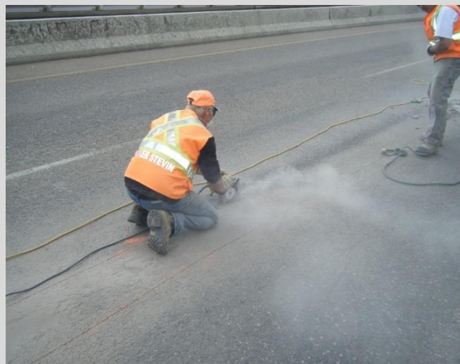
15.2 Sawcutting perimeter of deteriorated polymer repair area.
