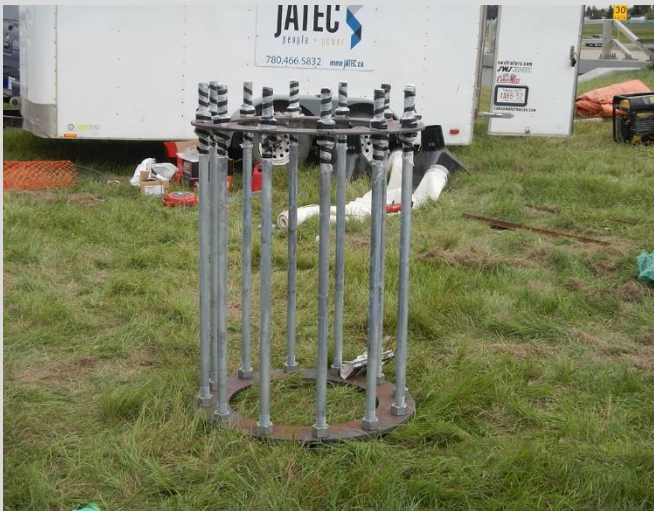
24.3 Anchor rod assembly. Threaded ends wrapped in poly to maintain cleanliness, and tubes sealed to protect from concrete paste.
