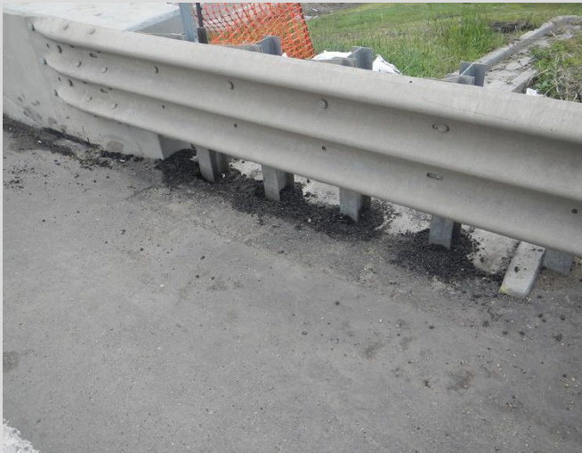
14.3 Guardrail transition posts.
