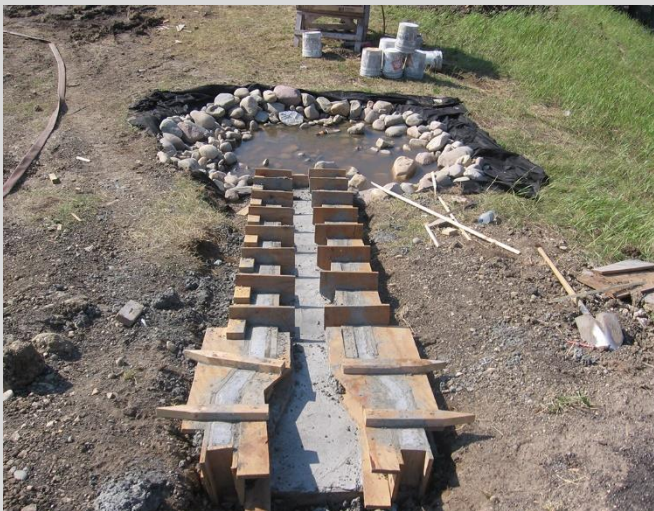
9.3 Drain trough with riprap terminal protection.
