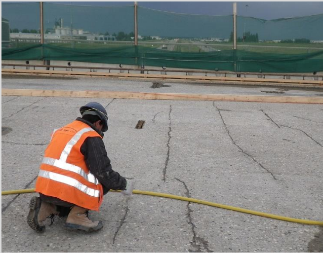
20.13 Cracks being filled with gravity flow epoxy.
