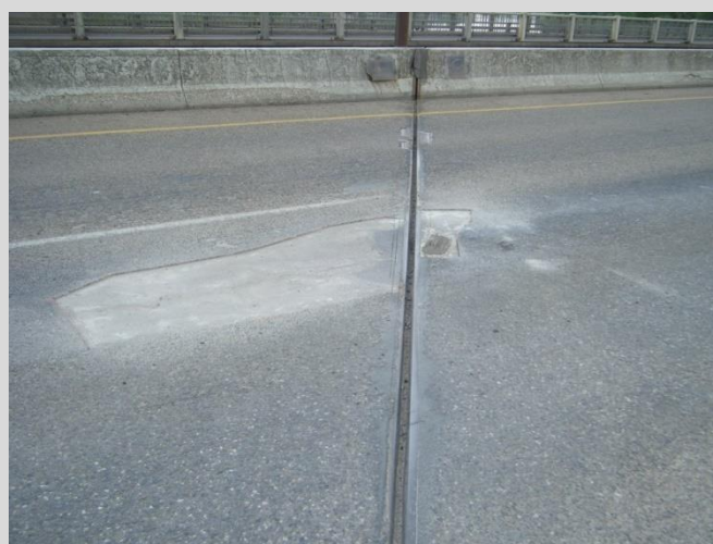
15.4 Prepared surface with completed patch and moisture contents confirmed.
