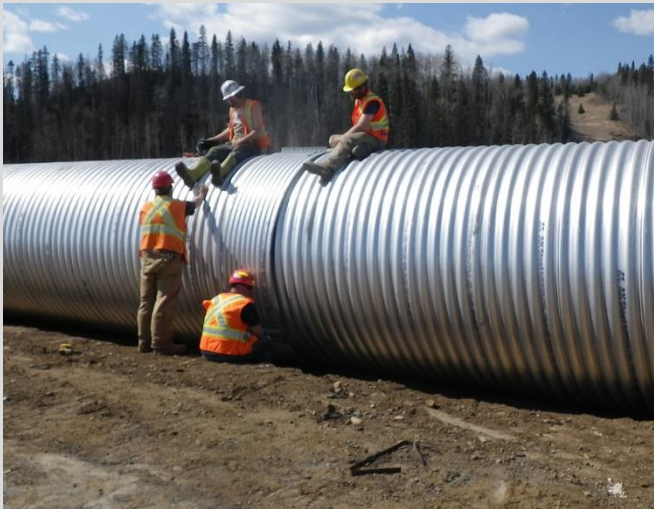
18.31 Installing CSP couplers.
