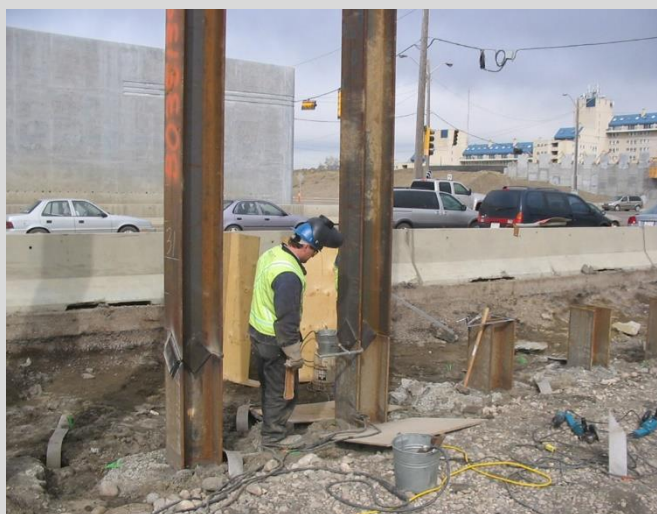
3.9 Tack welding of H-pile splices. 50% of final welds are completed before releasing H-pile from crane.
