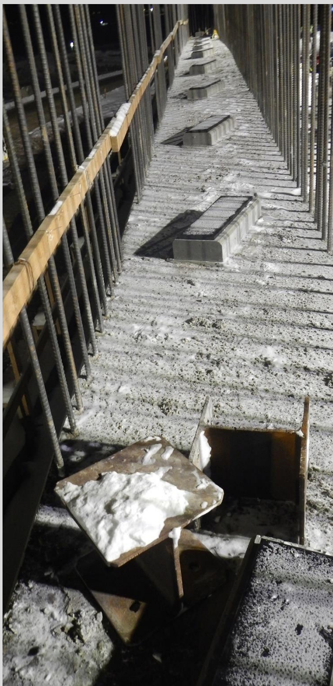
8.17 Concrete plinths on pier cap. Girder to be set on the plinths and cast with the diaphragm.
