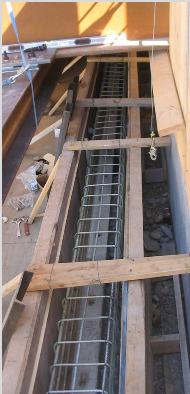
25.18 Cast-in-place coping cap.
