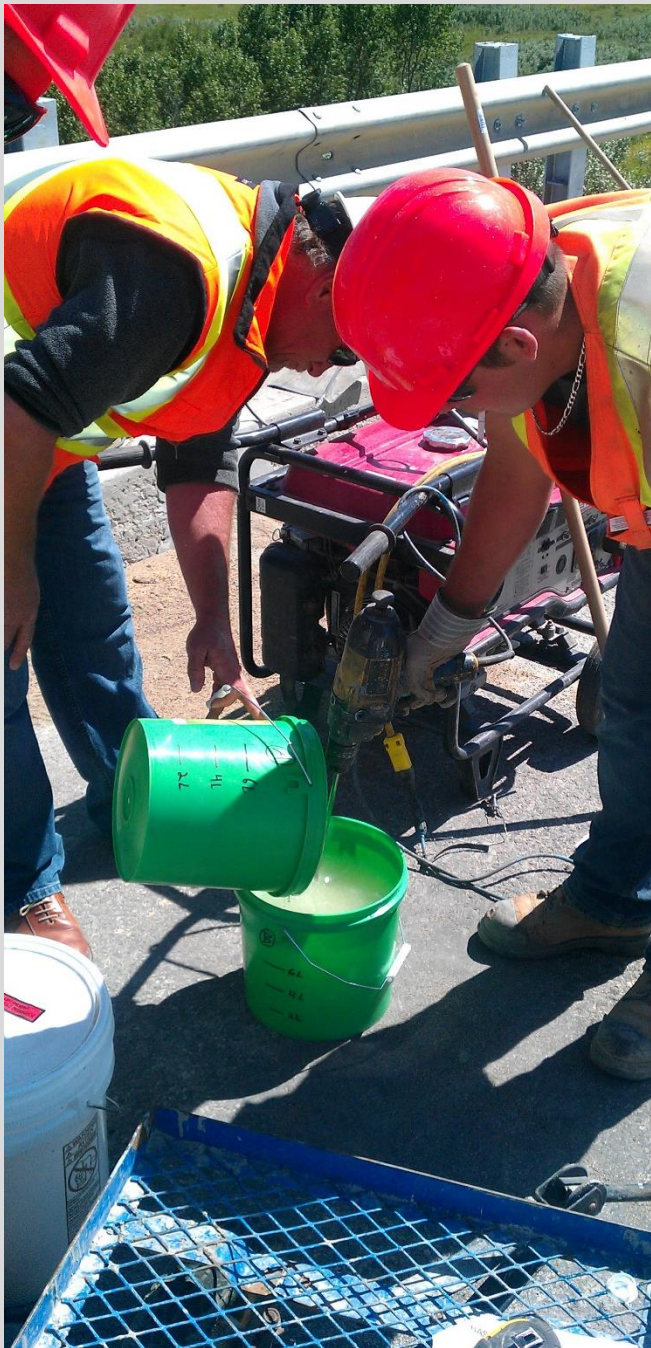
15.6 Polymer component mixing
