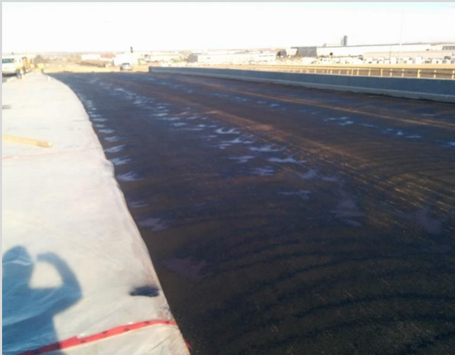
17.3 Application of tack coat by spray truck.
