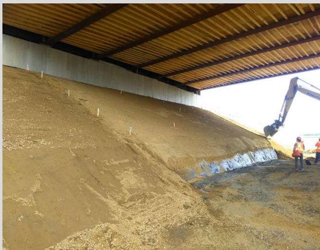
4.109 Excavation for toe cut-off wall
