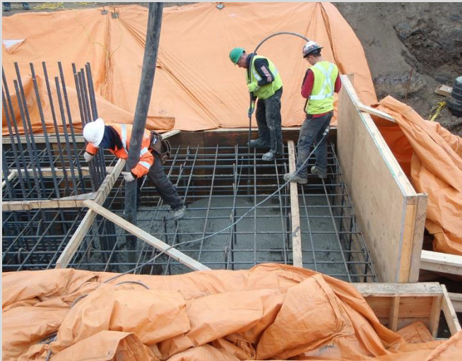
4.18 Substructure concrete placement. Long vibrator used to consolidate concrete for deep elements.
