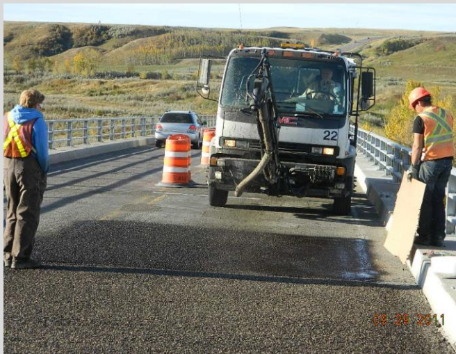
15.10 Spray patching over polymer repairs to blend into existing chip seal coat.
