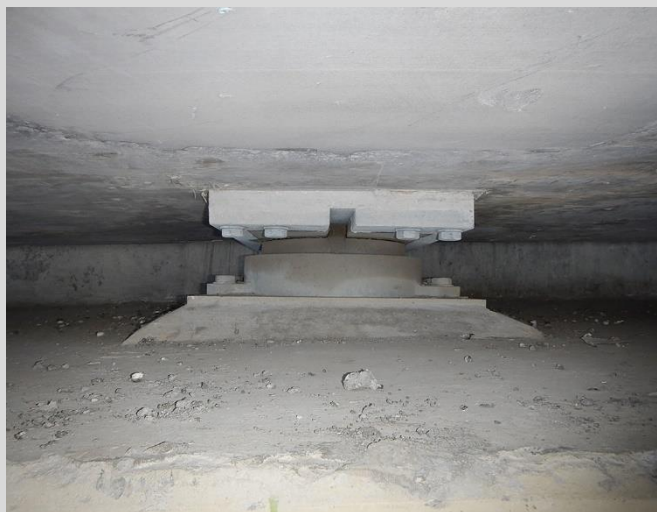
8.19 Grout pad constructed at 45 degree slope from abutment seat to bottom of base plate.
