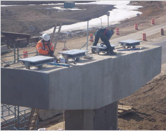
8.1 Placing bearings at pier cap.
