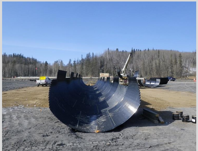
18.4 Assembling SPCSP culvert.
