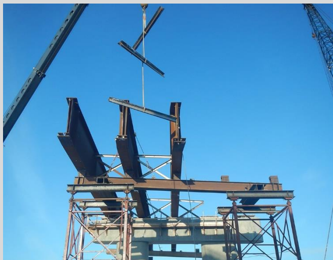
6.7 Steel diaphragm bracing installation with crane.
