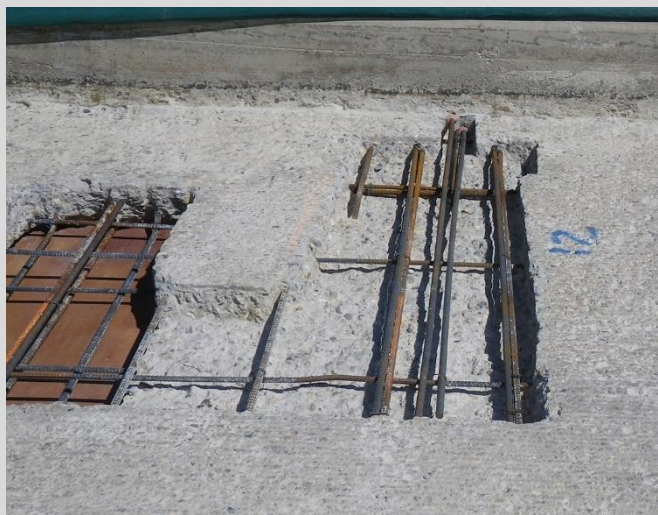
20.5 Full and partial depth repair areas prepared.
