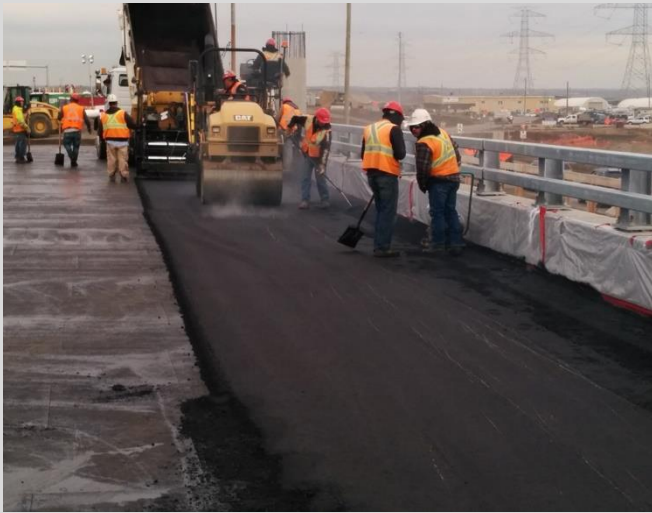
17.5 Placing first lift of ACP. Small smooth drum roller following as soon as practical.
