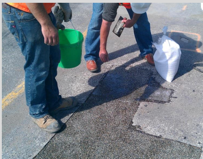
15.8 2nd polymer layer placement seeded with aggregate.
