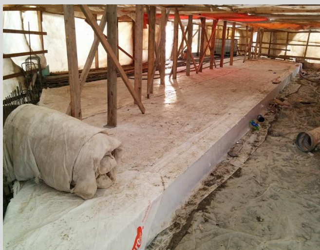
4.75 Heating and hoarding during winter curing.
