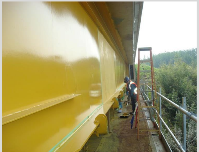
22.8 Applying finish coat of paint.
