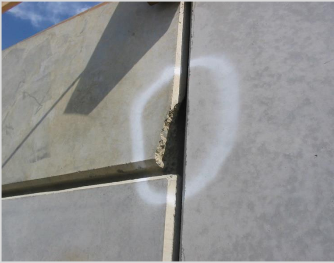
25.19 Panel damaged during erection.
