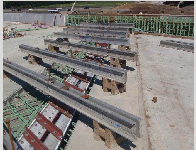
6.12 Deck joint installation. Deck joint gap set in accordance with the "Expansion Gap Setting Table" found in the design drawings.
