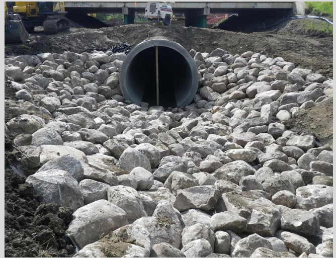
26.14 Completed placement of heavy rock riprap.
