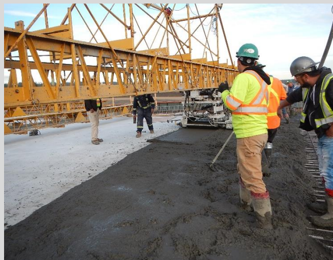
4.56 Deck concrete placement is placed in transverse strips so that it can be screeded as soon as practical after placement and vibration.
