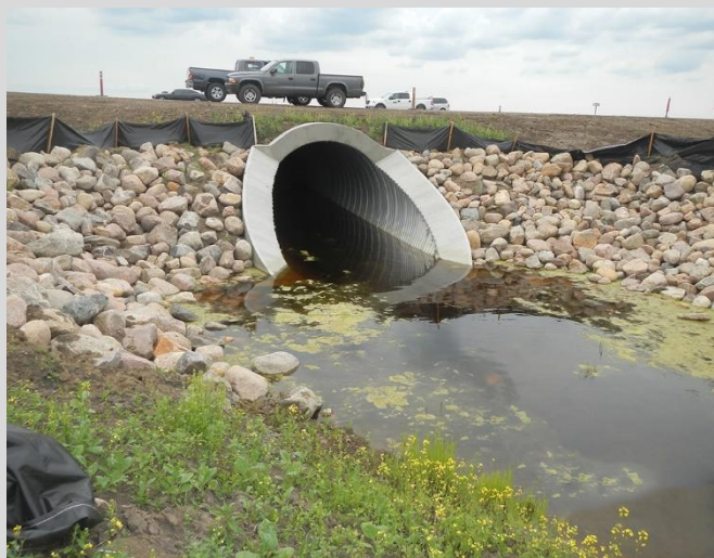
18.25 Completed collar and heavy rock riprap.
