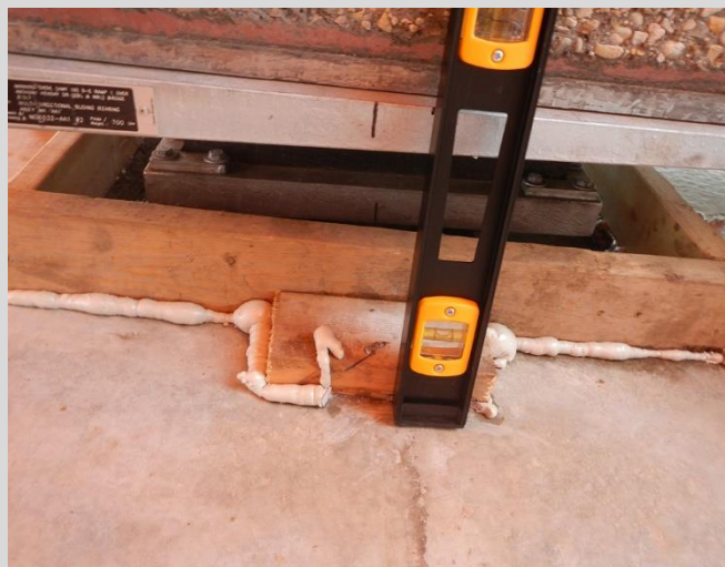
8.22 Setting bearing offset to "X" value in accordance with bearing temperature chart, just prior to grouting.
