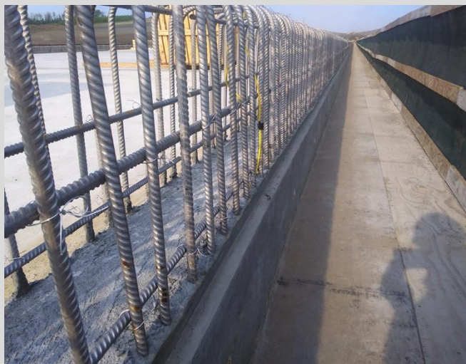
4.78 Typical construction joint at outside face of barrier. Note pour strip detail.
