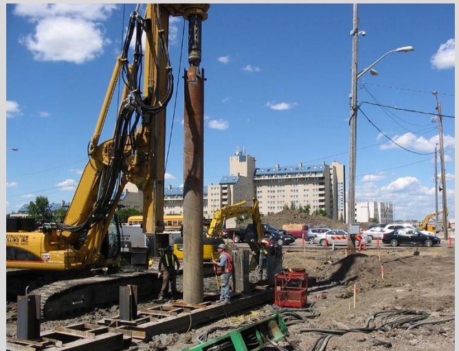
3.23 Drilling rig used to advance drilling casing. Kelly bar advances the casing into the excavation. For larger diameters, a vibratory hammer or an oscillator is used to advance the casing.
