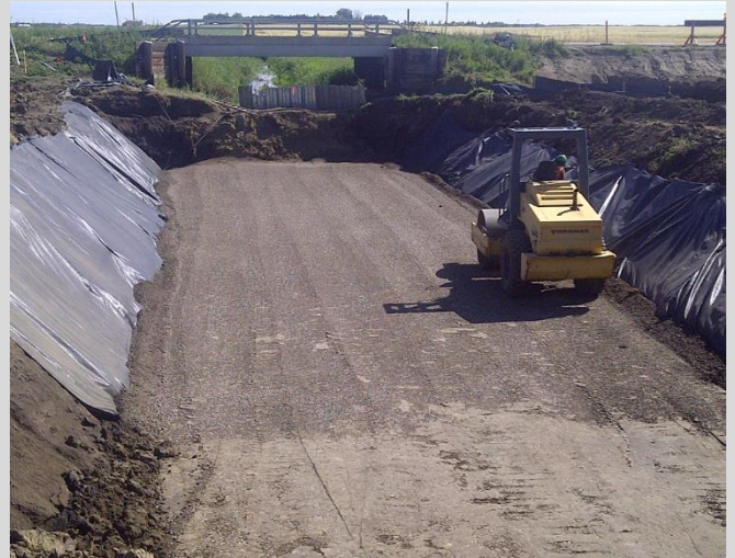
18.16 Backfilling of culvert bed.
