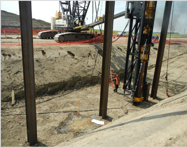
3.5 Diesel hammer piling rig shown. Centre of pile marked out by pins or flags. H-pile orientation painted on ground.
