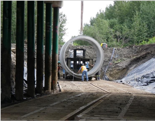
26.5 Placing first section of RCP.
