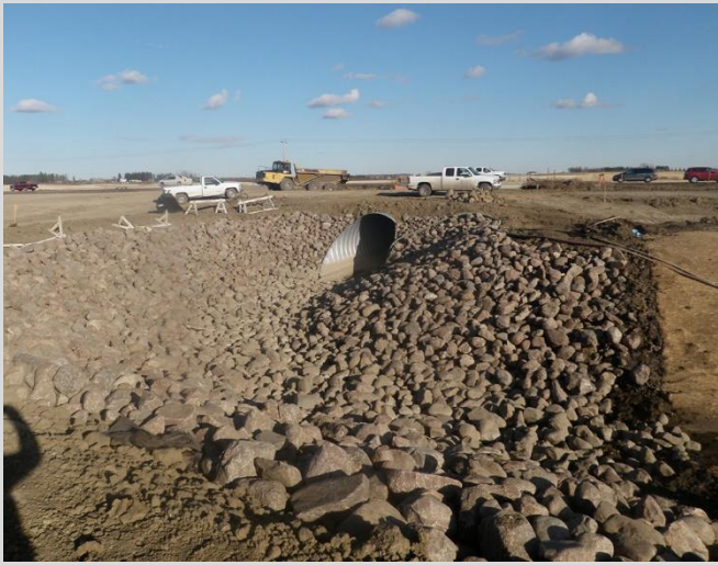
10.5 Heavy rock riprap at culvert bevel.
