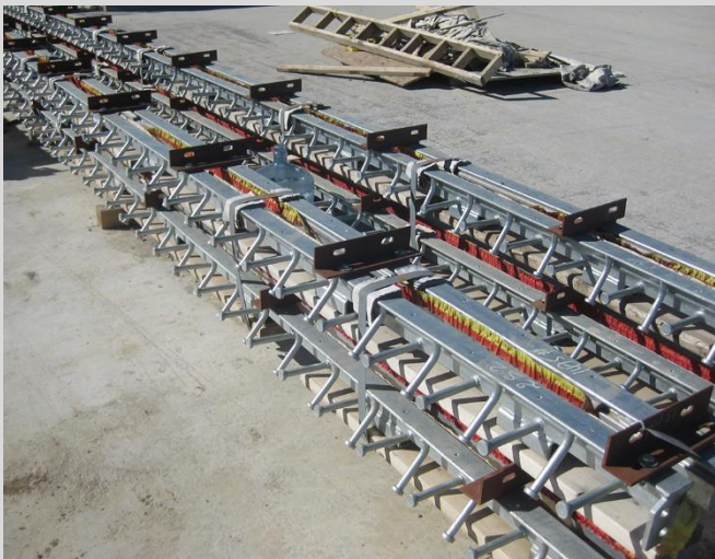
6.11 Deck joints stored on site and on timber dunnage to prevent damage.
