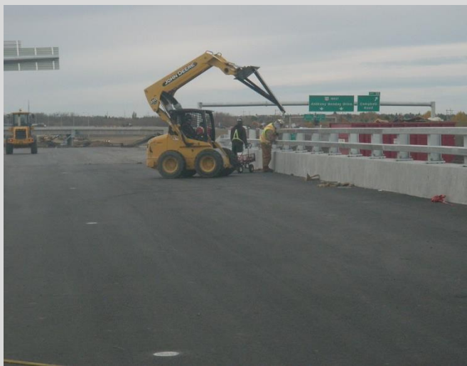
12.1 Installation of bridgerail. Bolting railing to posts.
