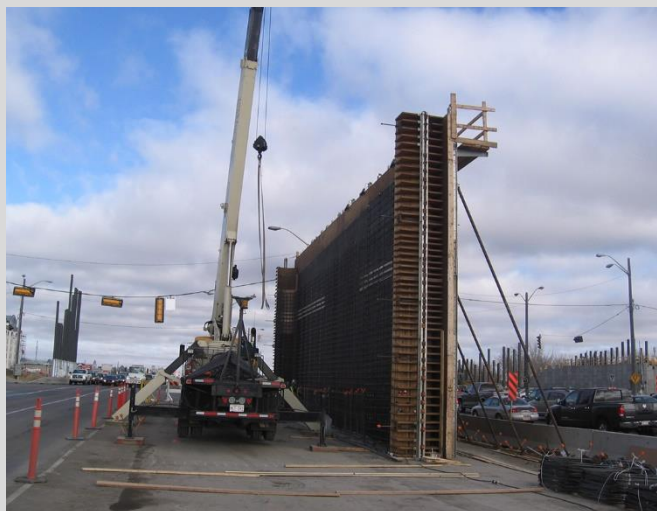
4.3 Pier shaft formwork being erected.
