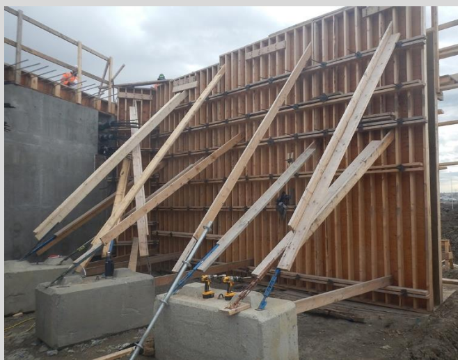
4.8 Formwork bracing for wingwall. Waler form construction used. Forms braced using deadman lock-block anchors.
