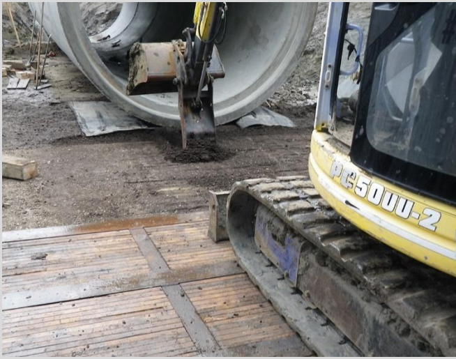
26.9 Loader loosening bedding material at bell.
