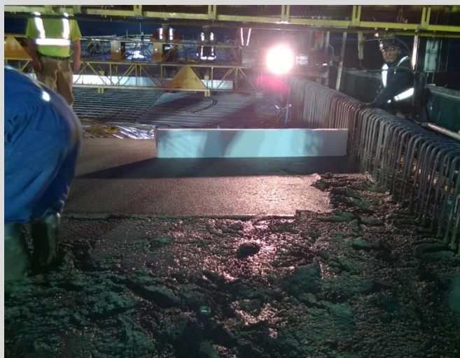
4.63 Straight edge checks must be done in both the transverse and longitudinal directions along the gutter as hand floating is done.
