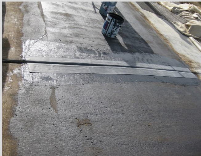
16.8 Membrane reinforcing fabric placed along construction joint.
