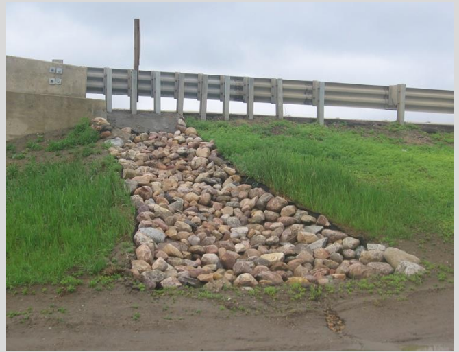
9.2 Riprap drain trough.
