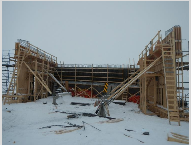
4.7 Partial wingwall and backwall formwork.
