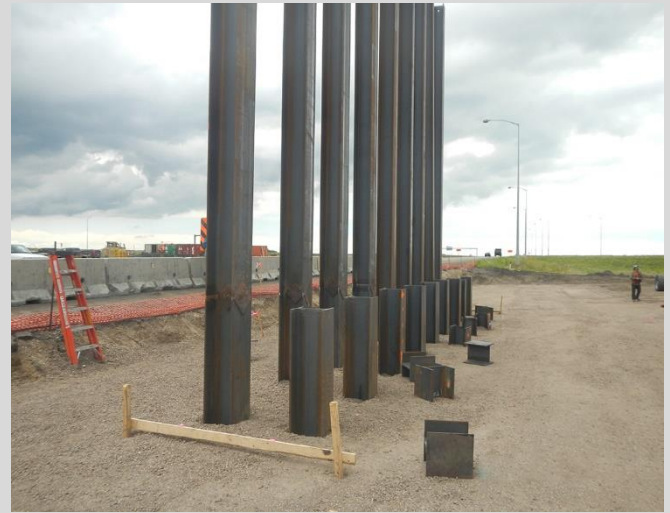
3.6 Batterboards and string line set up with 2x4s. String line offset to re-establish pile location.
