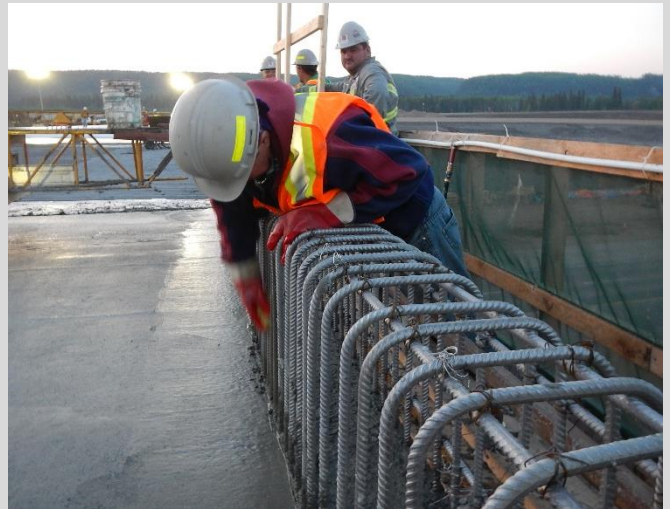
4.62 It is important that paste be removed from barrier reinforcing steel prior to initial set.
