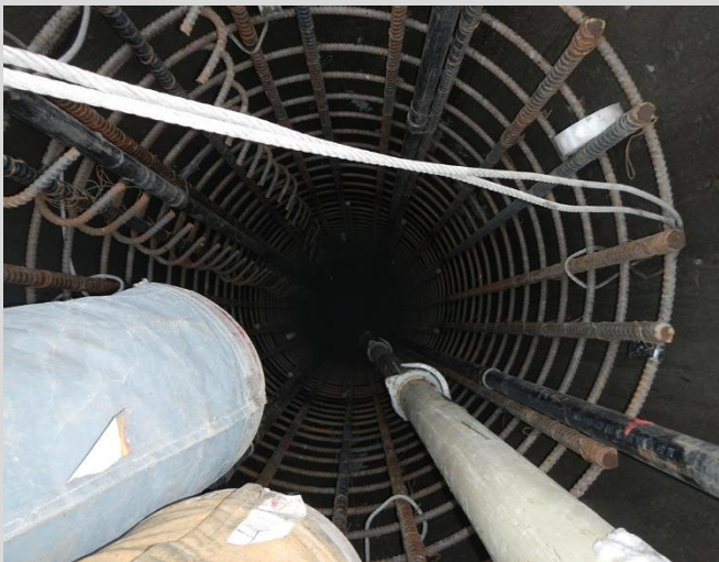
3.34 Concrete pumped through tremmie pipe. Cross-hole Sonic Log (CSL) pipe attached to reinforcing steel (black pipes).
