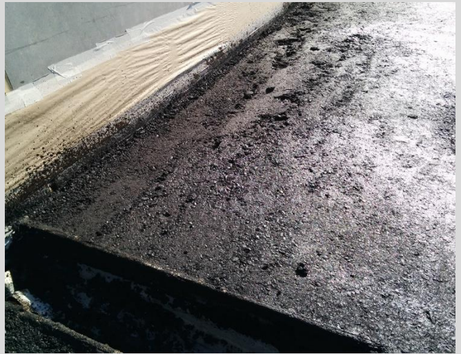
17.10 Unacceptable segregation near barrier face.
