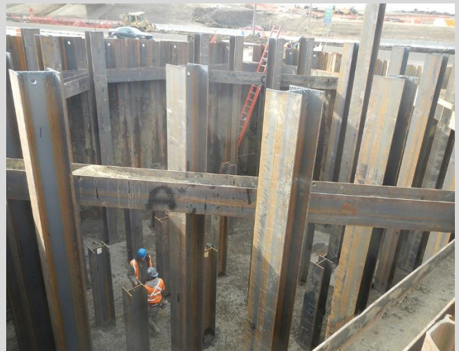
1.4 Sheet piling installed for pier piling cofferdam. H piles placed horizontally as bracing. Ladder access to excavation.
