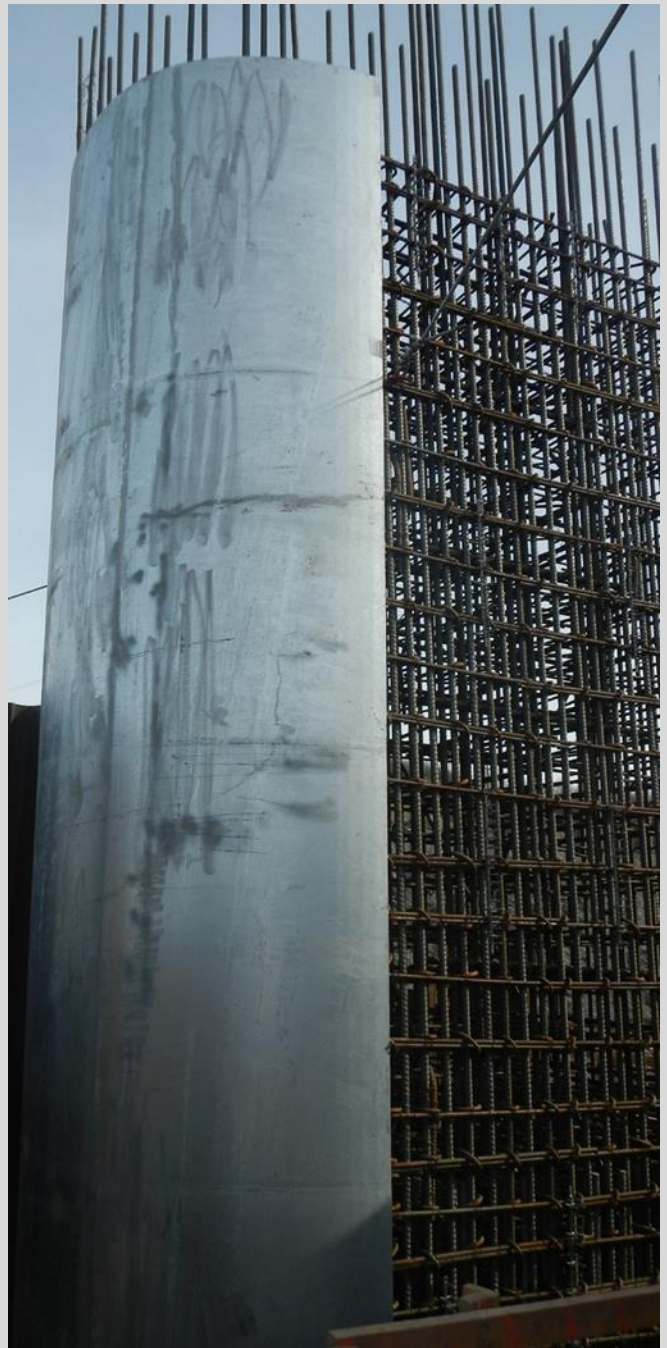
6.21 Galvanized nose plate for river pier protection.
