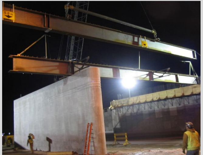
6.25 Steel girders are sometimes erected in pairs and stabilized with steel diaphragms.
