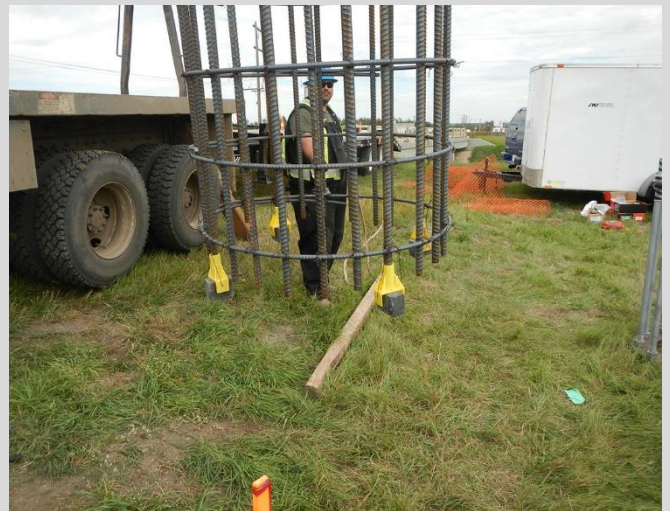
24.4 Plastic chairs used to maintain bottom cover and prevent cage form punching into ground at base.
