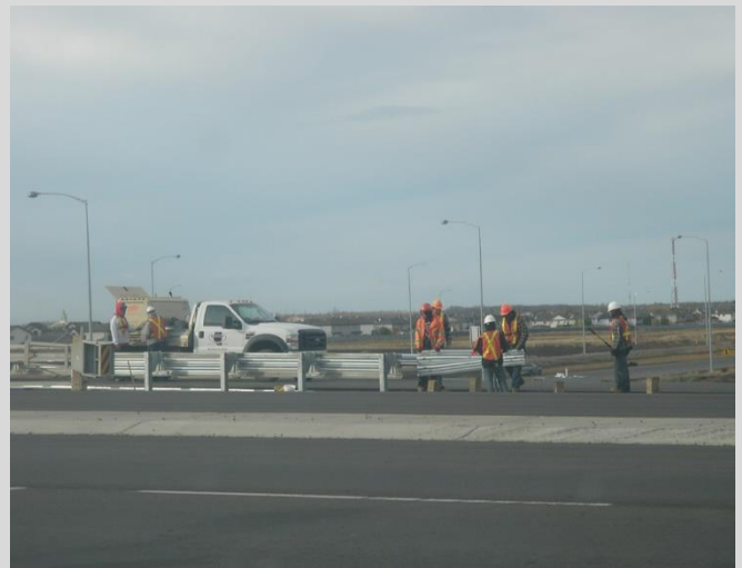
14.8 Installing guardrail to posts.
