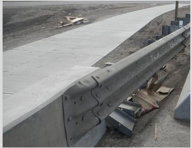
14.2 Guardrail to bridgerail transition.
