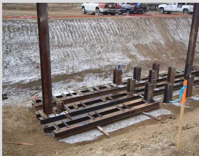
3.4 Pile driving frame used to position piles accurately at the start of driving. Frame is anchored by welding to soldier piles.
