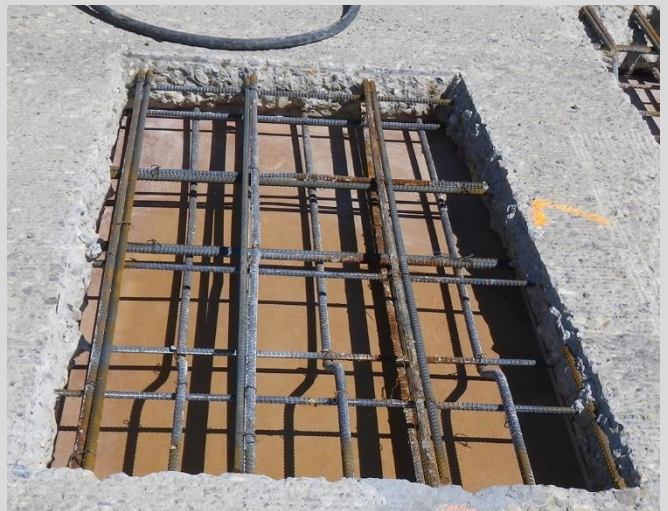
20.4 Full depth repair area prepared.
