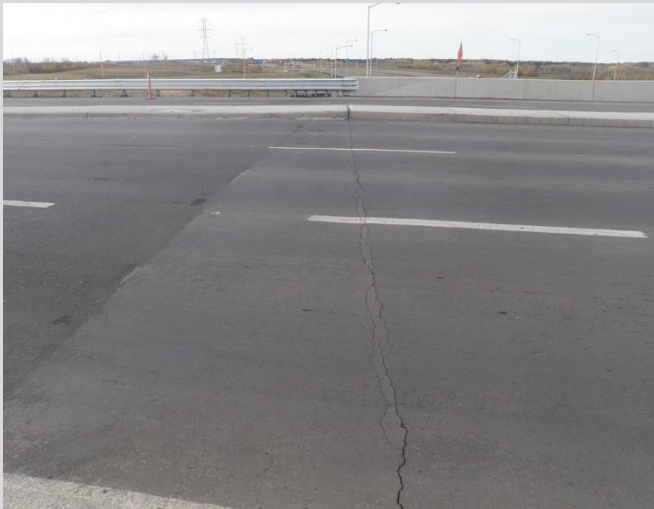
17.11 Cracking at approach slab transition.
