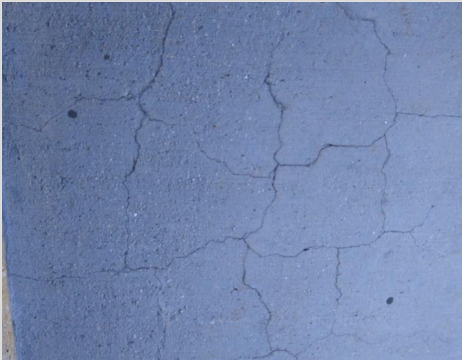
4.103 Drying shrinkage cracks on substructure.
