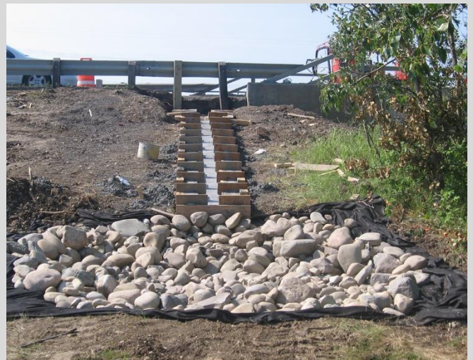
9.4 Drain trough with riprap terminal protection.
