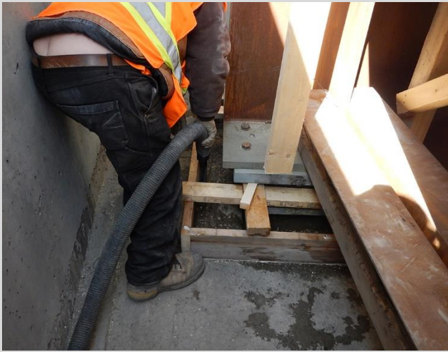
8.9 Clean-out prior to grouting.
