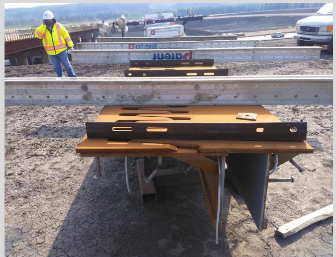
6.19 Finger type joint showing erection angles.
