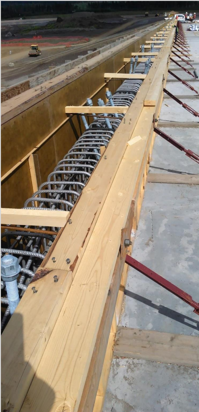
4.80 Barrier formwork showing anchor bolt assemblies, chamfer strip, and control joint crack initiator.
