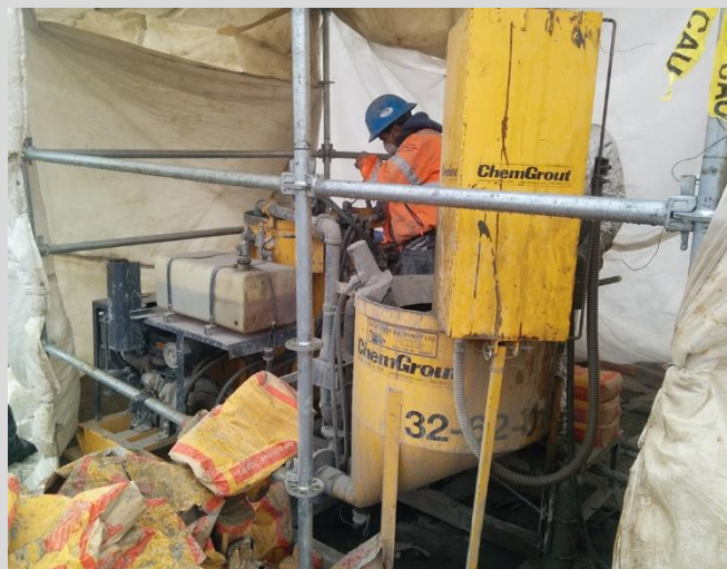
7.31 Grouting operation.
