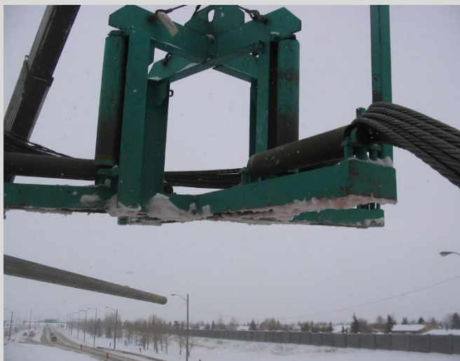
7.24 Strand pack dispenser for tendon assembly.
