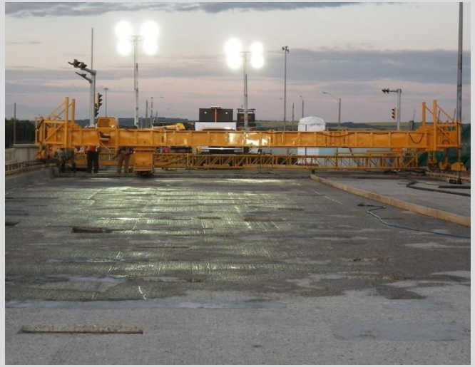
20.18 Deck finishing machine for concrete overlay pour.
