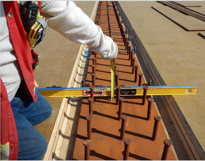
4.39 Prior to installation of reinforcing steel, it is important to check actual haunch values at all girder 10th points to confirm form position accuracy.
