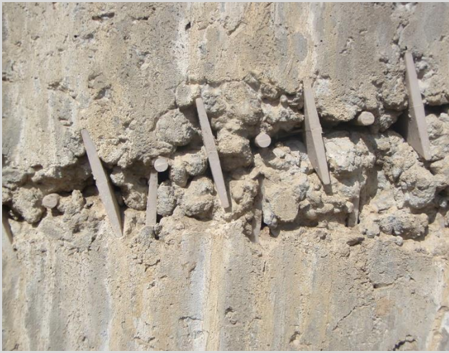
5.13 Improper chair placement or inadequate consolidation does not allow concrete to flow and may cause honeycombing.
