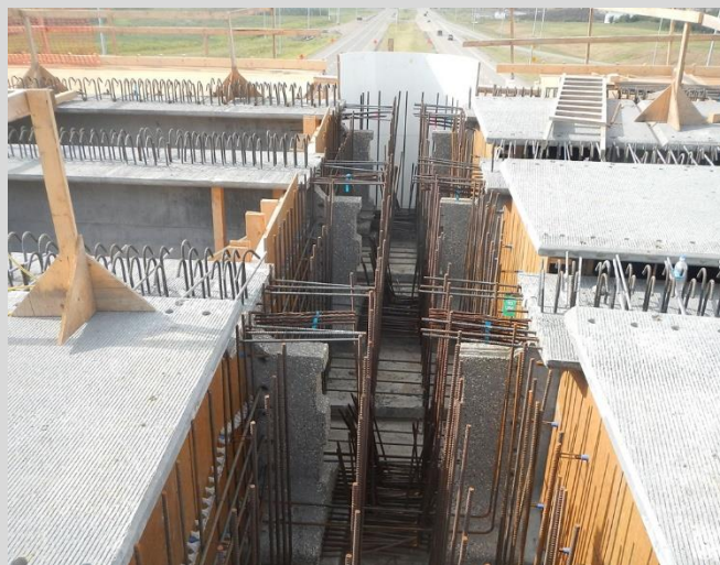
4.11 Pier diaphragm formwork and reinforcing steel.
