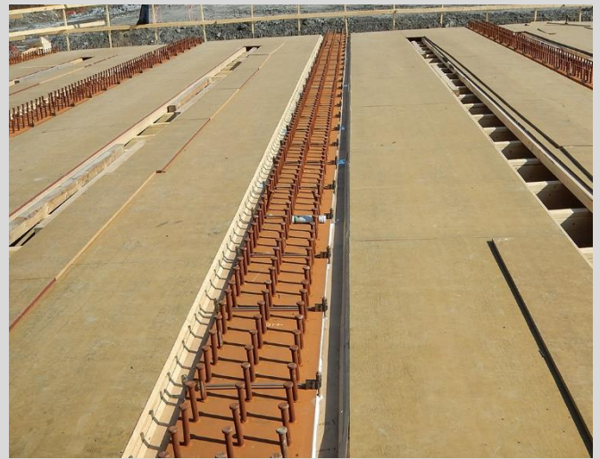
4.36 Joists and plywood are placed onto ledgers. Neat chamfers must separate the haunch and interior bay formwork. Holes through plywood to accommodate coil bolts must be properly sealed.
