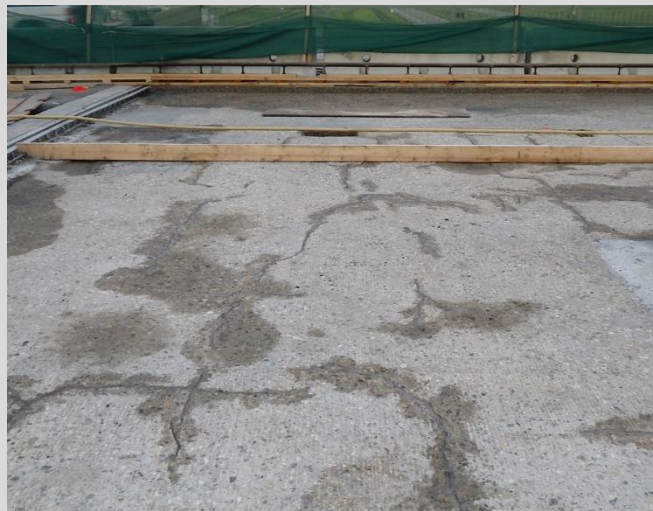
20.12 Cracks prepared for epoxy repair.
