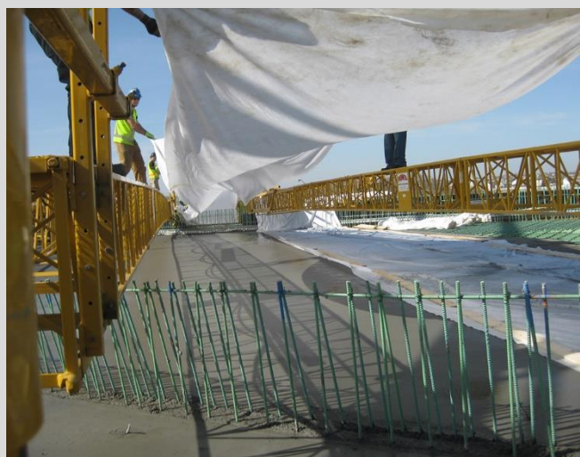
4.66 Placement of curing fabric from work bridges.
