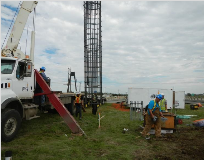
24.5 Installation of plain reinforcing steel cage.
