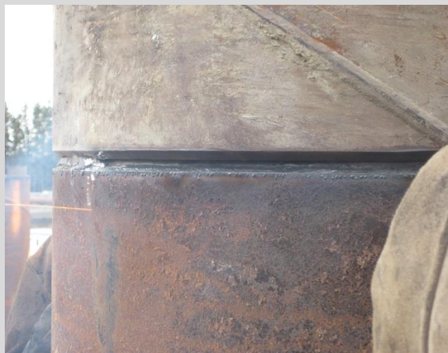
3.25 Splicing pipe pile shown after fit-up.
