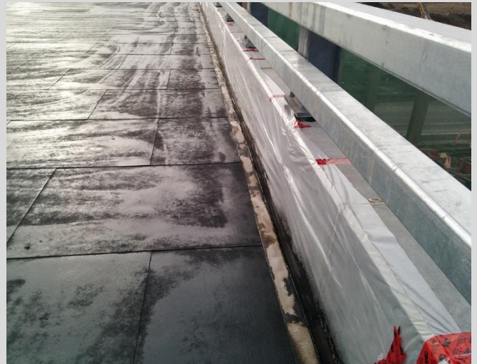
17.4 Wick drain and barriers protected from tack spray. Plastic strip placed over wick drain, and barriers covered with poly during spraying of tack coat.
