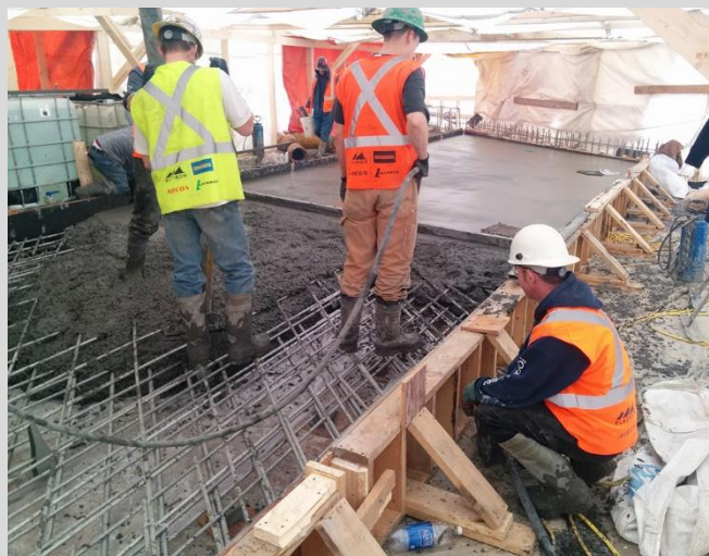
4.74 Placing approach slab concrete.
