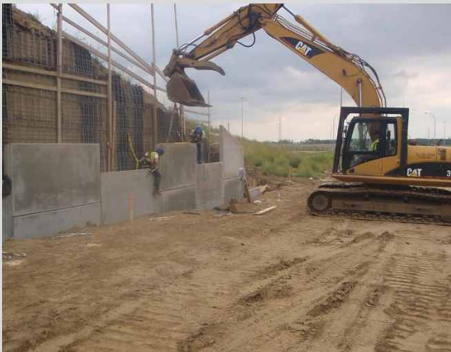
25.29 Installation of 2 nd stage panels.
