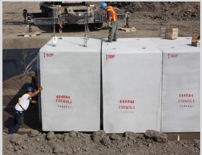
26.16 Erection of PBC unit.
