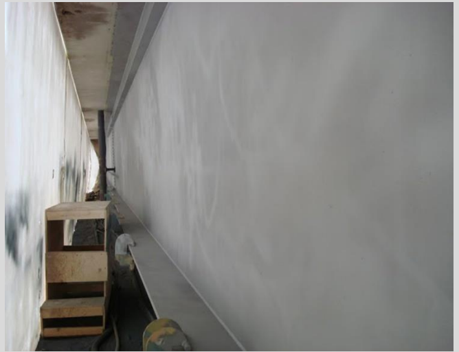
22.6 Girder after sandblasting.
