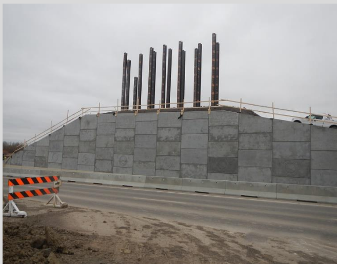
25.16 Completed backfilling and panel installation. Panels require cleaning prior to application of pigmented sealer.
