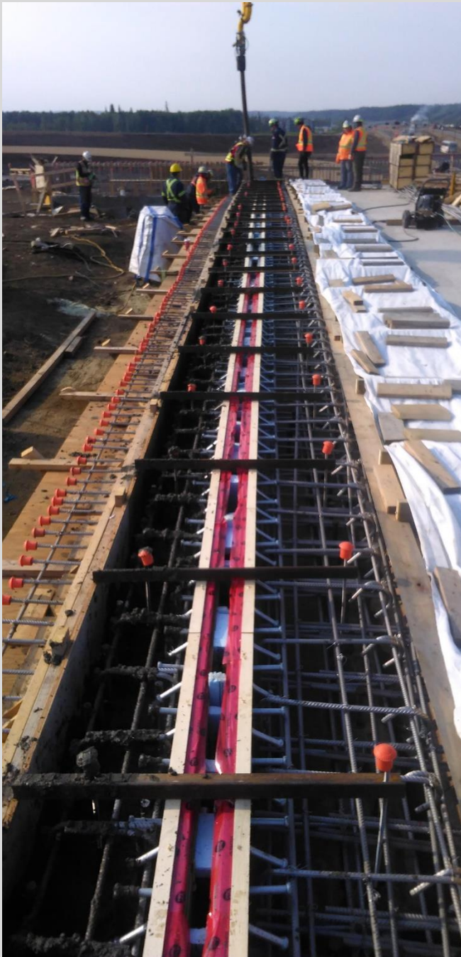
6.18 Casting abutment side of strip seal deck joint.
