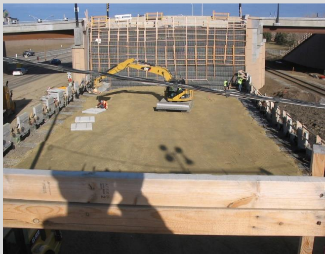
25.13 Two stage wall construction.
