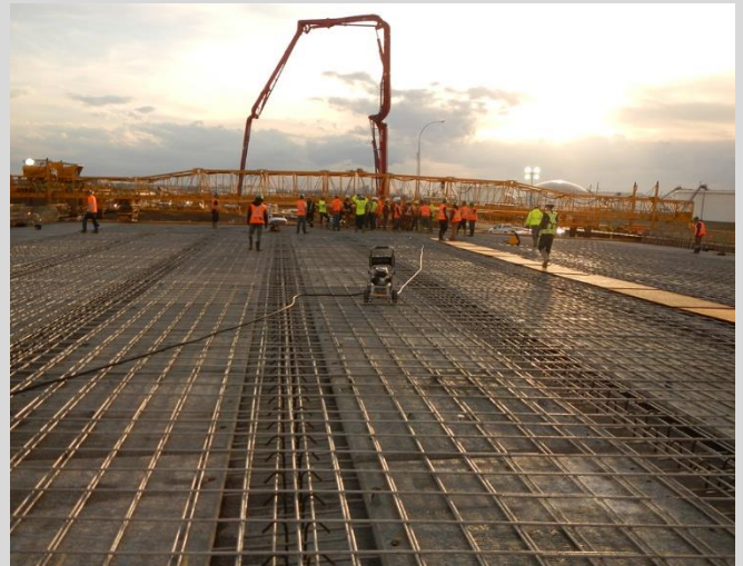
4.54 Start of deck pour. Plywood walkway on deck reinforcing steel for safety and protection of reinforcing steel. Pressure sprayer for cleaning and wetting deck.
