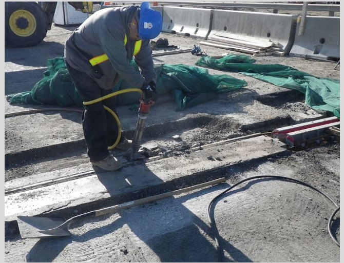
20.14 Existing deck joint removal using pneumatic hammer.
