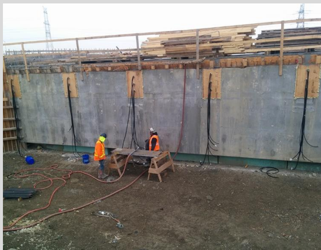
7.32 Workers open and close bleed tubes as instructed by the post-tensioning supervisor.
