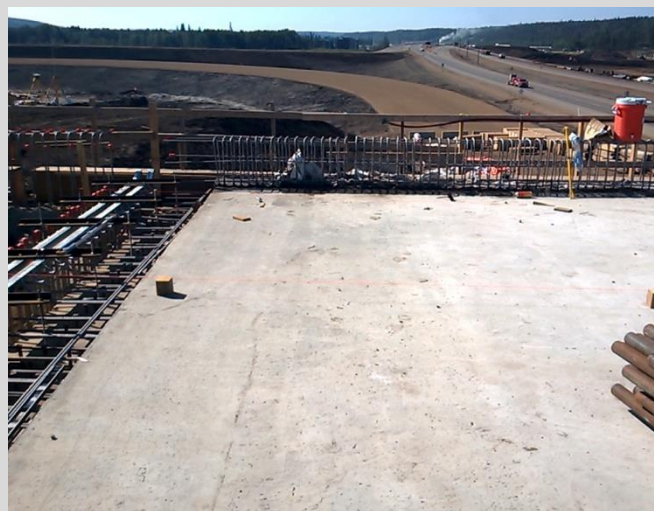
6.16 Strip seal type joint temporarily supported.
