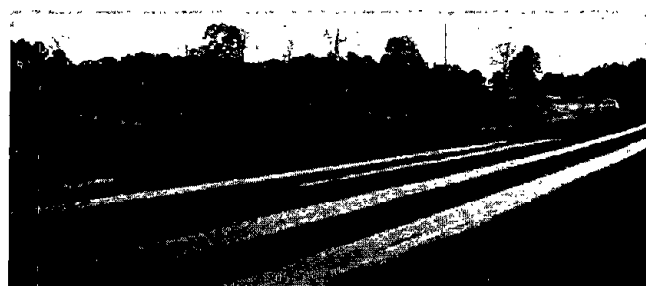
FIGURE 3 Extreme variation in friction (skid number of the advance pavement is 70, and skid number where the wheel paths have flushed is less than 10).
