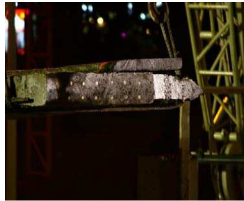
Figure 6.21 Section B-B – Béton sain
