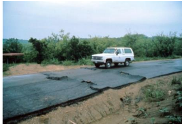
FIGURE 24: PAVEMENT DAMAGE FROM EXPANSIVE
