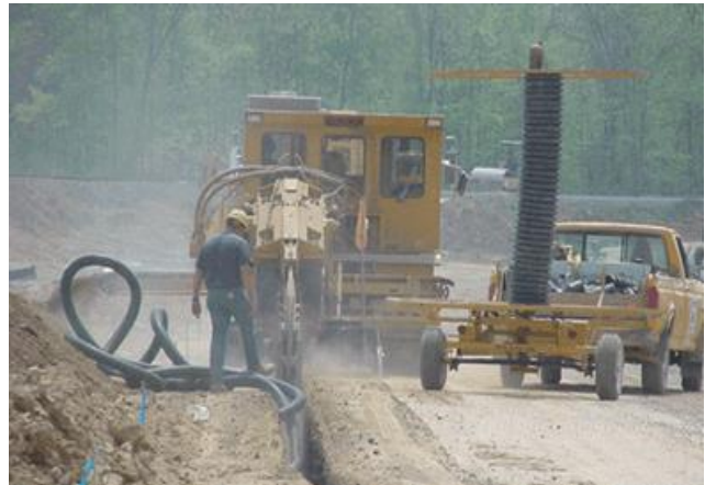
FIGURE 27: UNDERDRAIN INSTALLATION.
