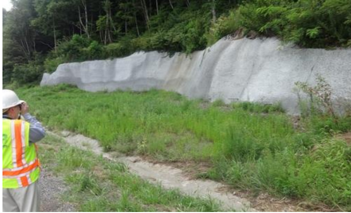
FIGURE 28: COMPLETED TOE WALL AT THE BASE OF THE SLIDING MASS AT I-77, MP 1.8 , VA I-77.
