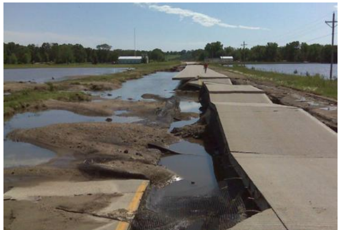
FIGURE 16: IA-1 FLOOD DAMAGE NEAR MOUNT VERNON, IOWA.
