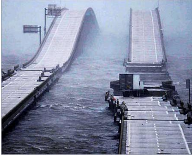
FIGURE 11: SOME OF THE 2004 DAMAGE TO THIS INTERSTATE BRIDGE CAN BE ATTRIBUTED TO THE SEA LEVEL RISE THAT OCCURRED IN THE PREVIOUS DECADES (I-10; PENSACOLA, FLORIDA).
