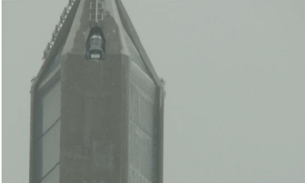
Figure 1.19: Ice accumulation on pylon glazing February 24, 2011
