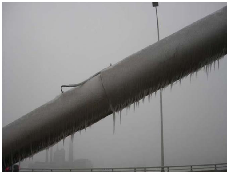
Figure 1.3: Ice Accumulation on the East Side of VGCS (Baker, 2007)
