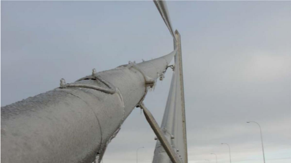
Figure 1.11: Ice Accumulation up east side of stay February 22, 2011
