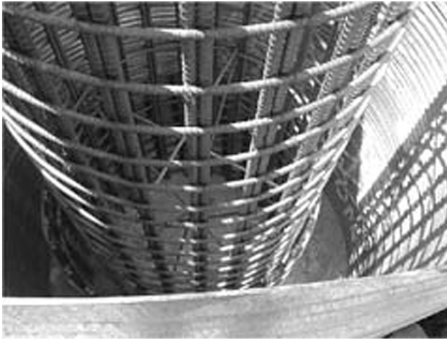
Fig. 2.2.2(c)—Hoop reinforcement in a reinforced concrete column (courtesy of HDR Engineering, Inc.).
