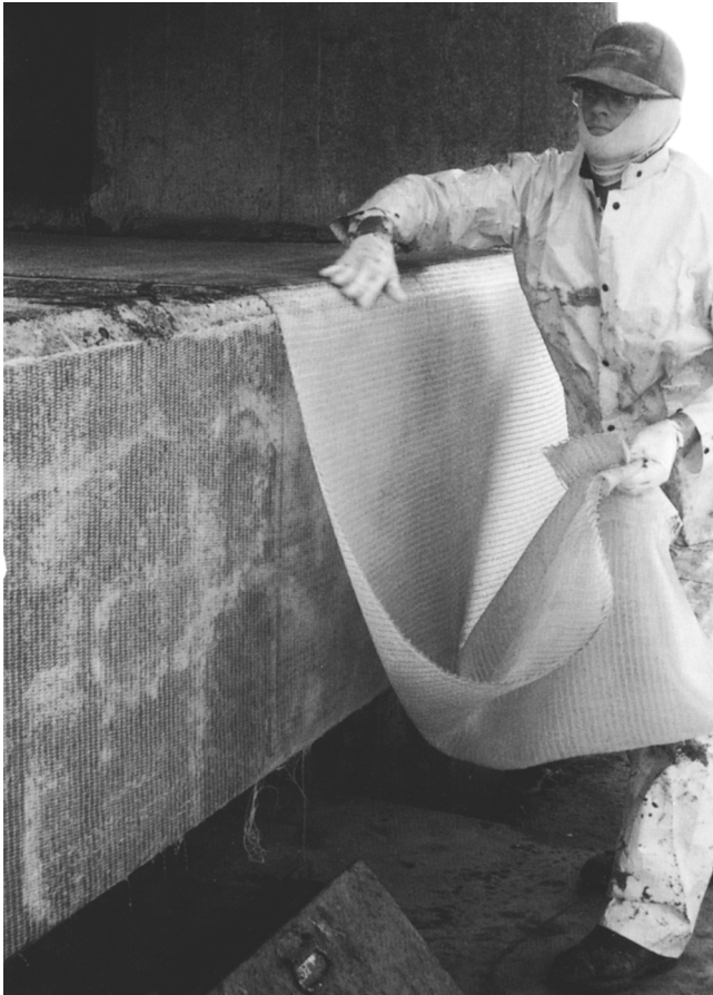
Fig. 3.4.2—Installation of FRP sheets on a reinforced concrete beam (courtesy of Hexcel Fyfe Co.).
