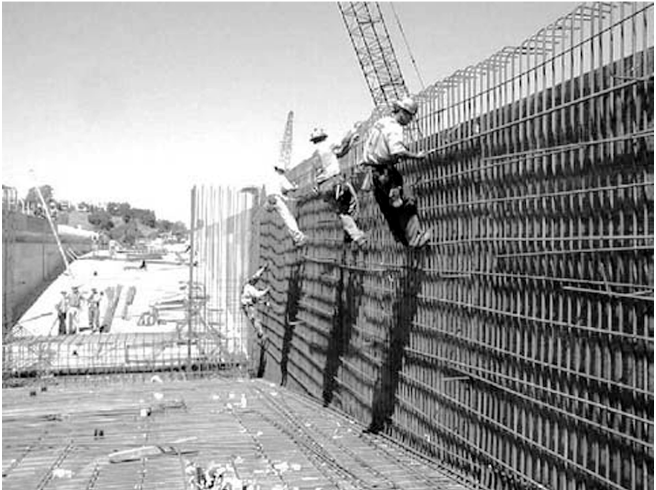
Fig. 2.2.2(b)—Stirrups to resist shear in a concrete box girder bridge (courtesy HDR Engineering, Inc.).
