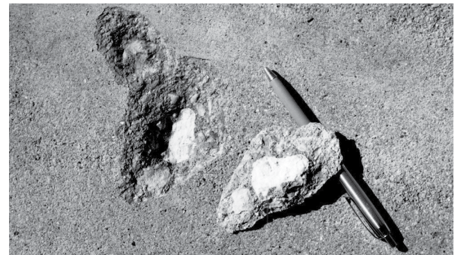
Fig. 3.7.3—Popout due to unsound aggregate particles.
