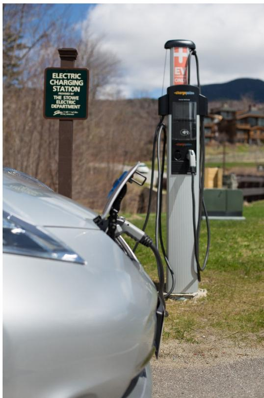
Figure 15. ChargePoint Level 2 EVSE in Stowe.
