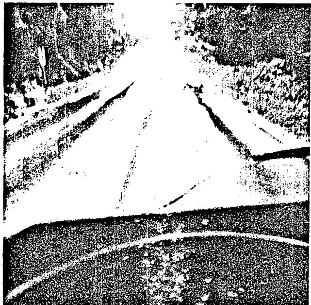
This rutting caused by traffic is the result of a combination of compaction and plastic flow. Such pavement failure could be avoided by using compaction requirements and a bitumen content reflecting a stable equilibrium condition under the design load as determined by the GTM.
