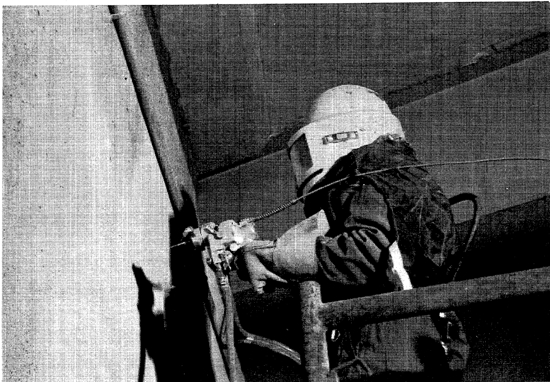
Figure 17/ Application of Flame-Sprayed Zinc Anode
