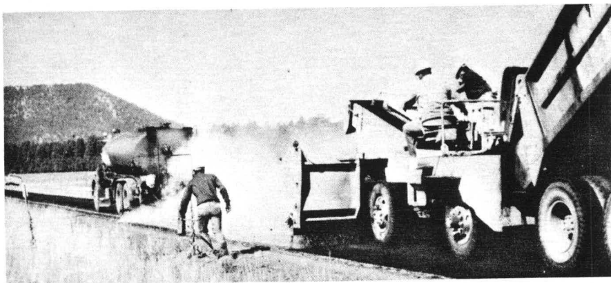
Modified distributor truck lays asphalt-rubber membrane, followed by chip spreader.
