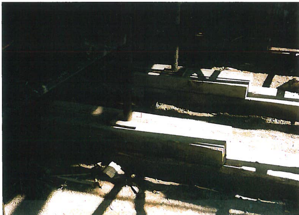
Figure 6.6 Mudsill Splice
