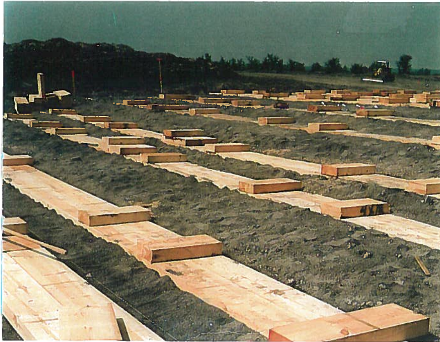
Figure 6.1 Site Preparation and placement of mudsills
