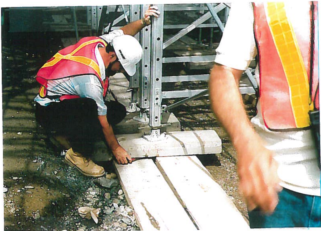
Figure 6.5 Void Under Sill
