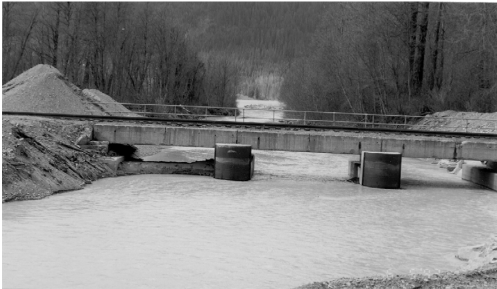
The stream is crossed by a road bridge followed by a railway bridge.
