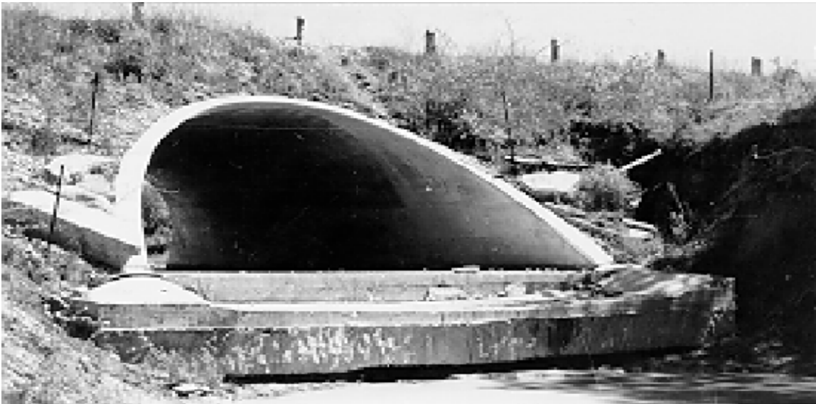
Figure 7.16: Degradation at Recently Added Concrete Floor and Cutoff
