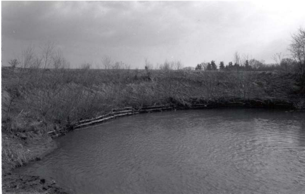
Figure 10.11: Live Cribwall Installations on Small Stream
