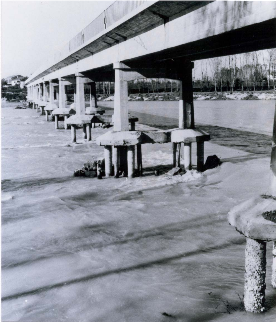
Figure 9.04: Foundation of Bridge Piers Removed by Upstream Progressing Degradation Caused by Gravel Excavation Downstream From the Bridge.
