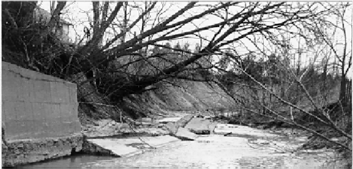
Figure 7.13: Stream Bed Degradation Exposing Retaining Wall Footing
