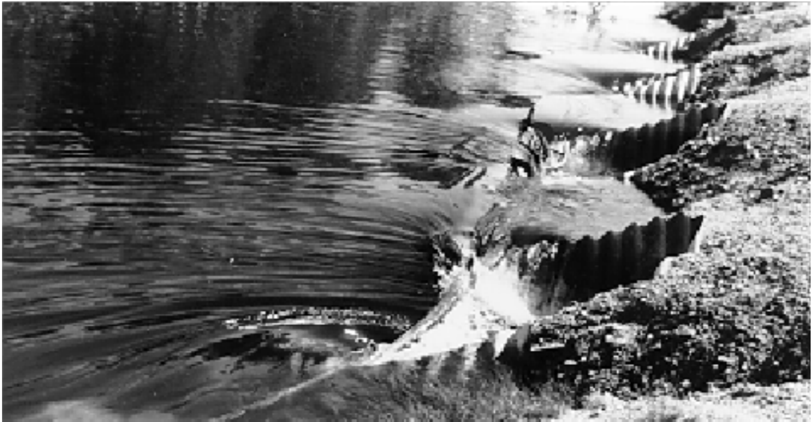
Figure 7.5: Flood Levels at a Culvert Crossing
