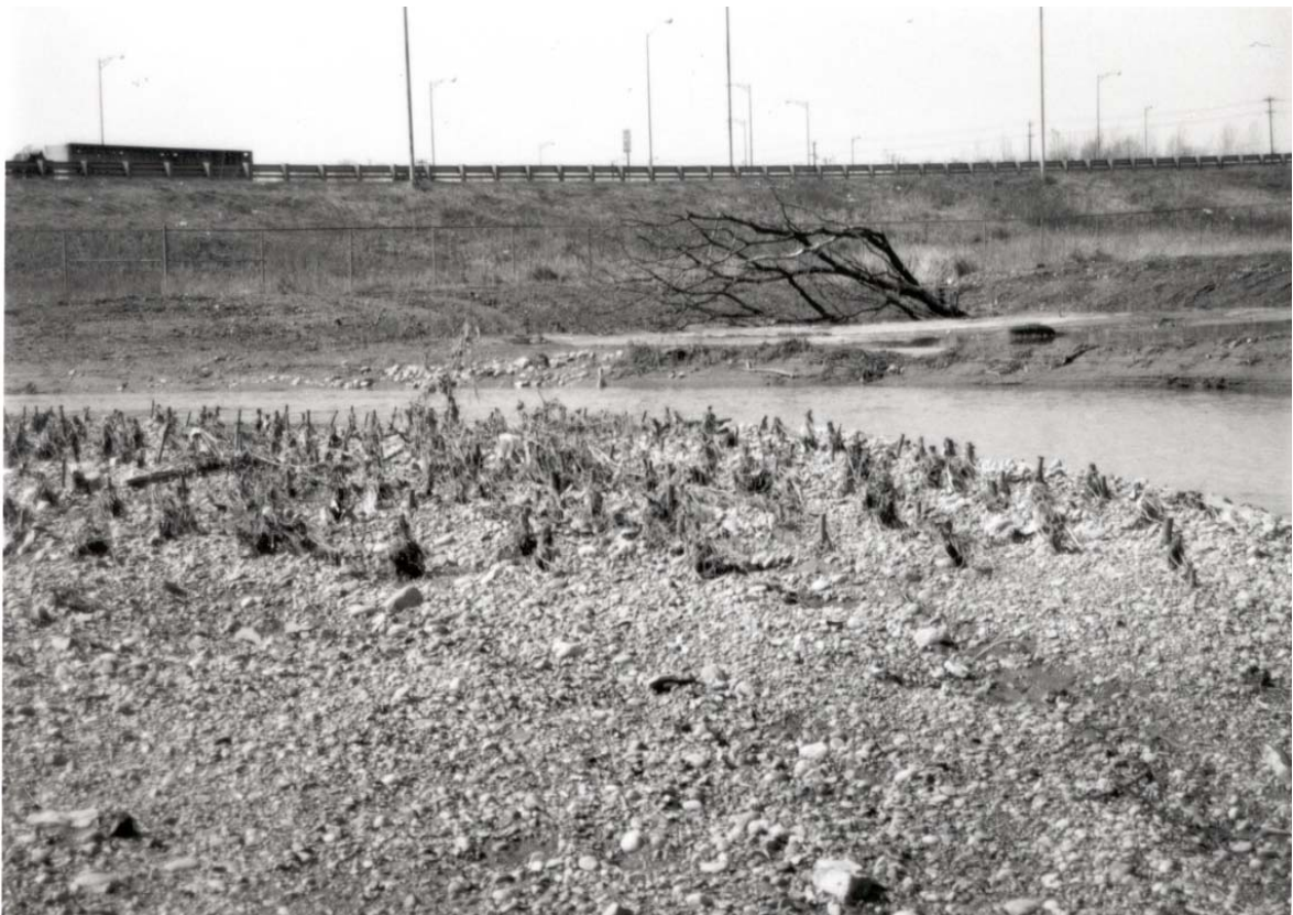
Figure 10.6: Live Stakes Used to Stabilize a Bar on Laurel Creek
