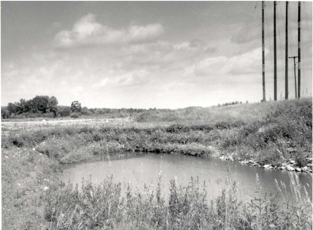
Figure 10.5: Brush Layer Used to Stabilize a Spillover Area
