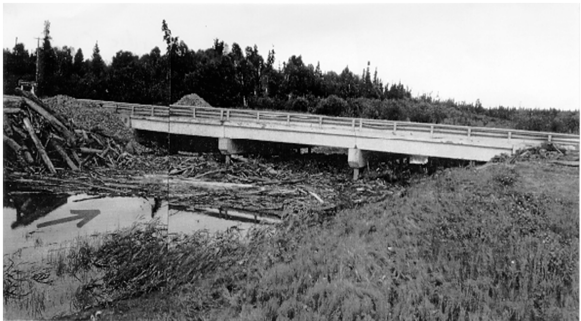
Figure 5.27: Bridge Opening Obstructed by Logs
