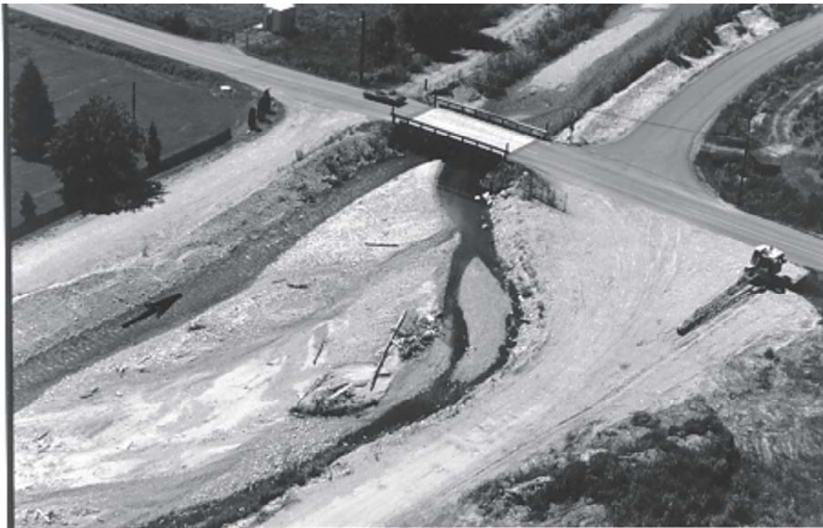
Figure 9.48: Deposition Indicated by Mid-channel Bars Upstream and Downstream from a Bridge.
