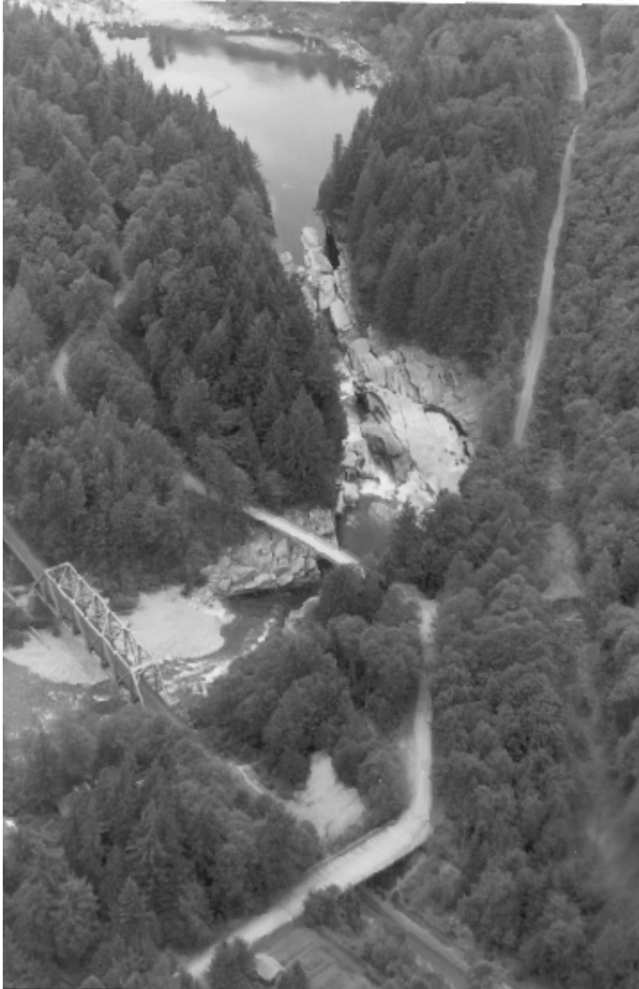
Figure 9.11: Narrow Bedrock Reach with Several Bridge Crossings.
