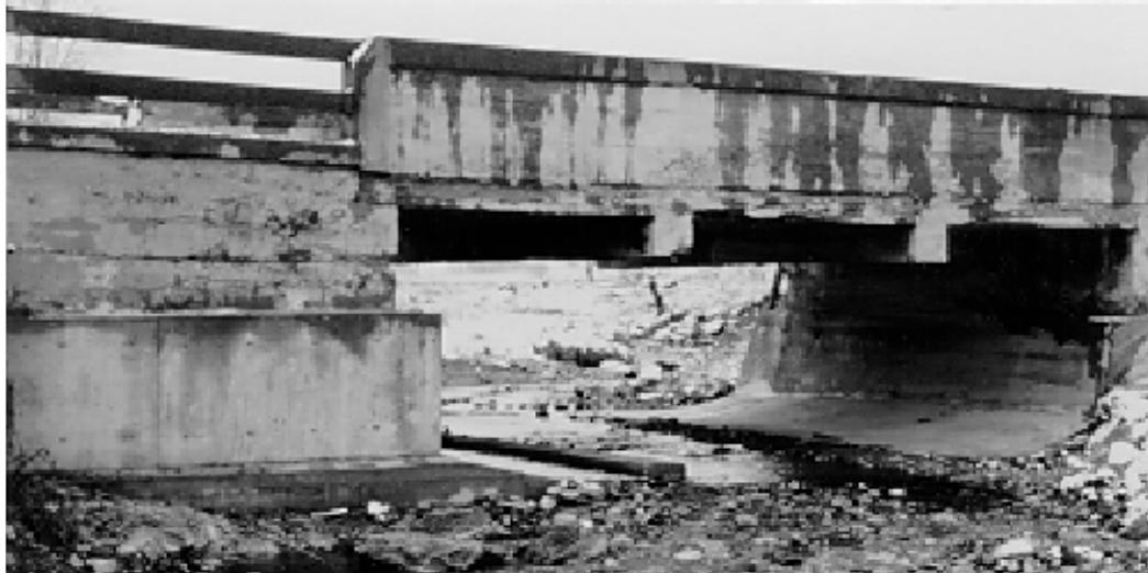
Figure 7.20: Scour Counter-measure Using Concrete Flooring
