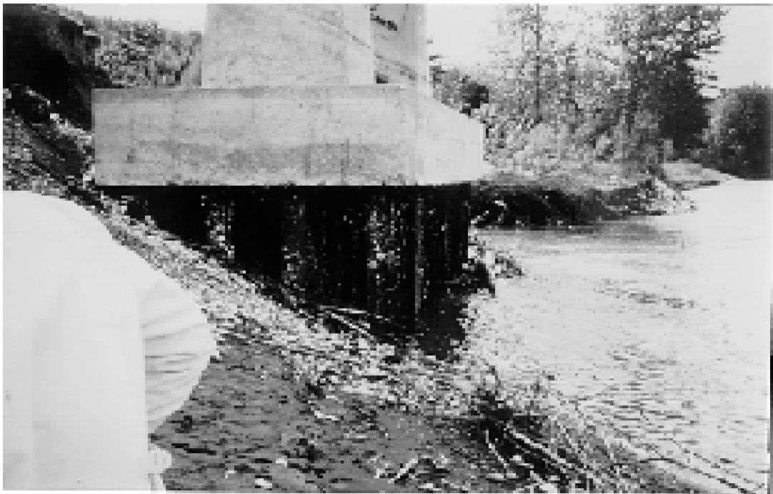
Figure 5.8: Local Scour at a Bridge Pier
