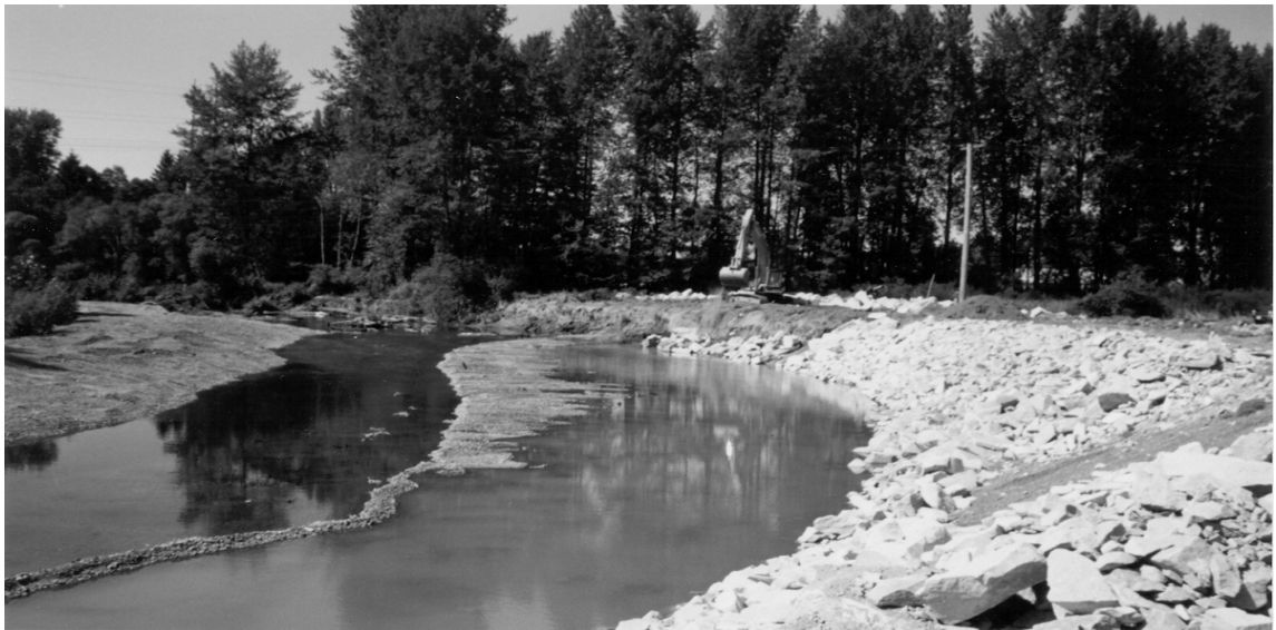
(b) Protected bank with no pools.
