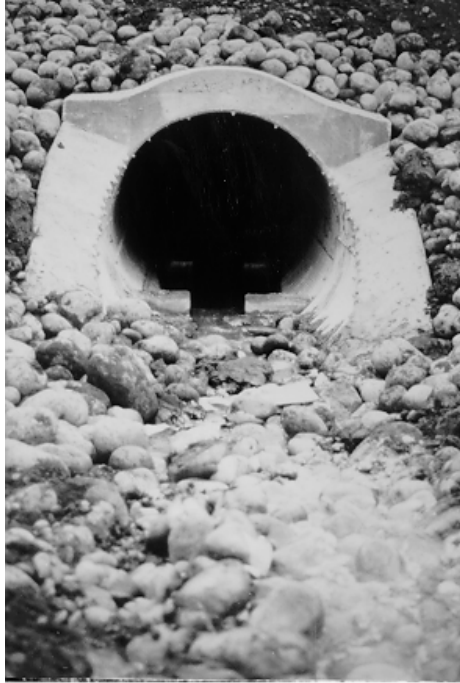
Figure 5.12: Slotted Weir Baffles in a SPCSP Culvert
