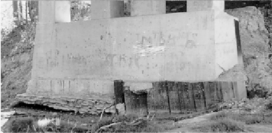
Figure 7.15: Degradation at Bridge Pier Footing
