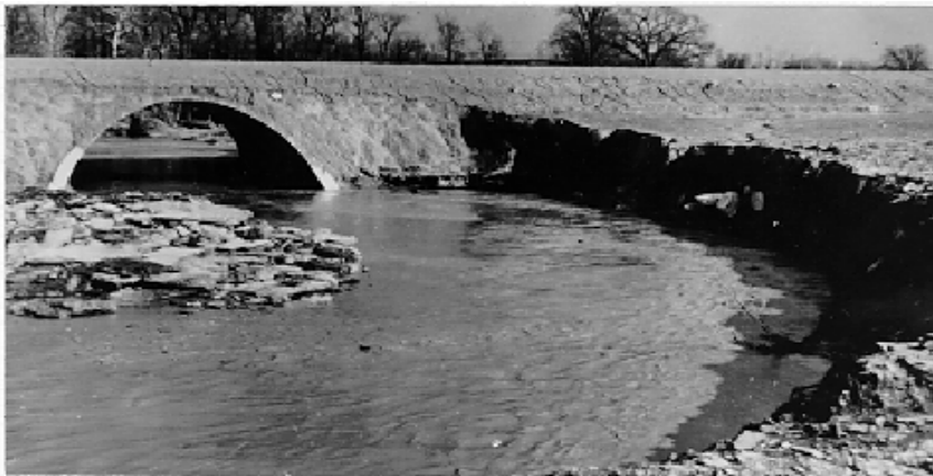
Figure 7.12: Undermined Check Dam Indicating Degradation
