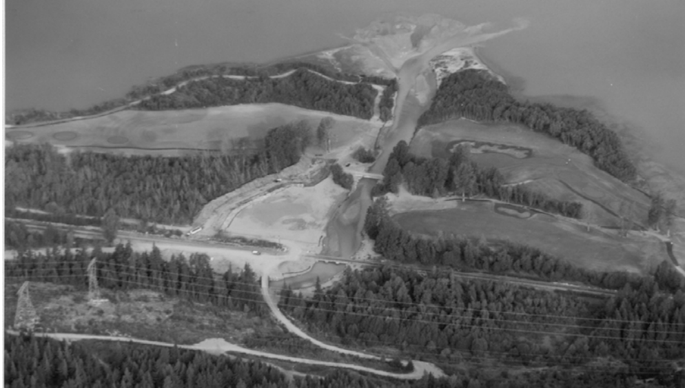
(b) Aggradation at railway crossing. Note the spoil pile on the left bank after excavations of the river bed.
