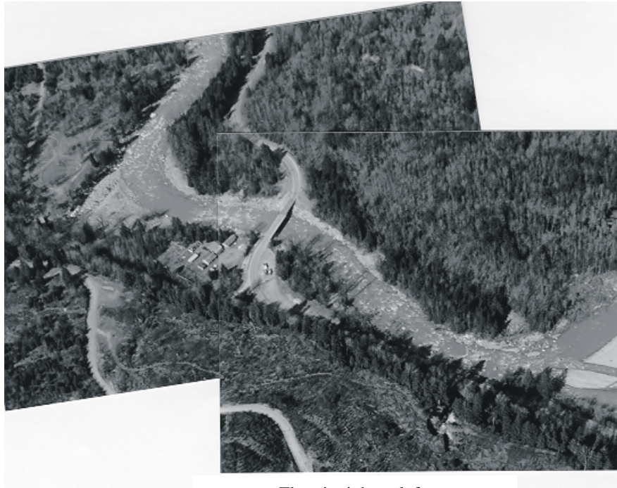
Figure 9.12: Boulder-lined Reach with Riprap Protection at Bridge
