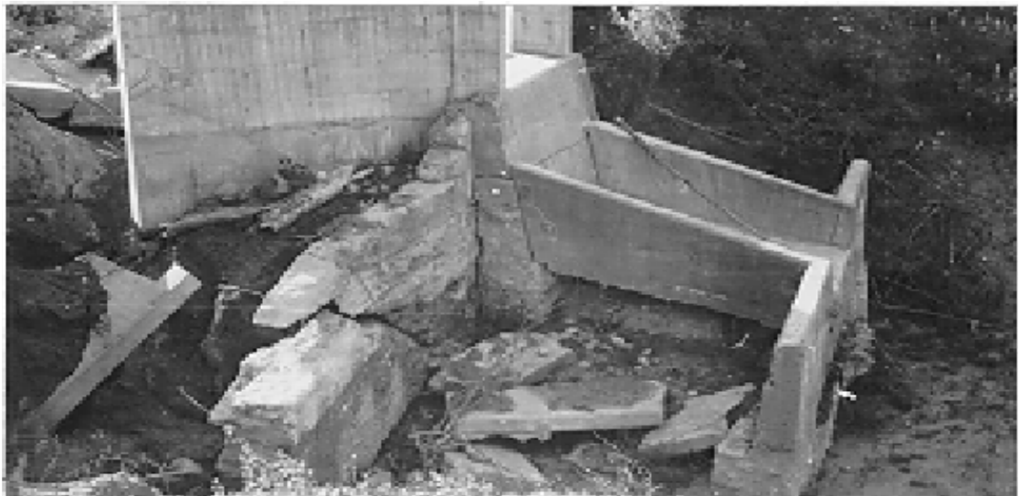
Figure 7.14: Undermined Flume Originally Constructed to Control Degradation at Culvert Upstream
