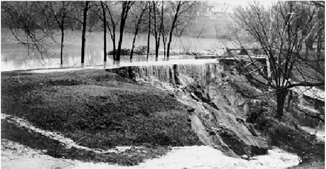
Figure 7.25: Earth Fill Dam Overflowing
