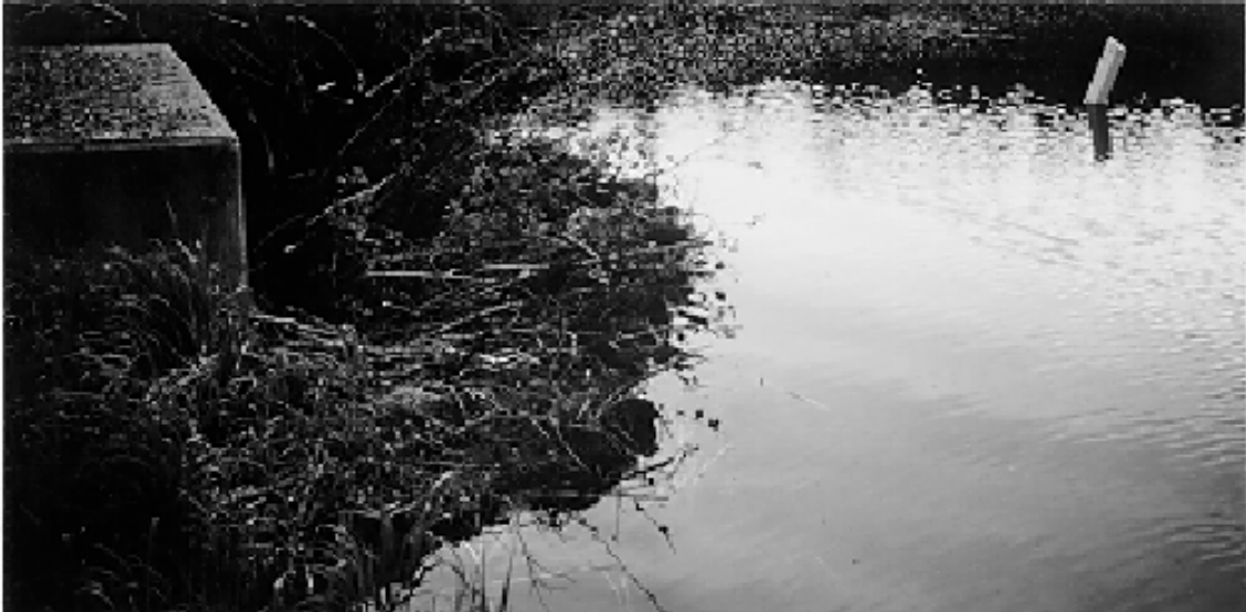
Figure 7.27: Beaver Dam at Inlet of Culvert
