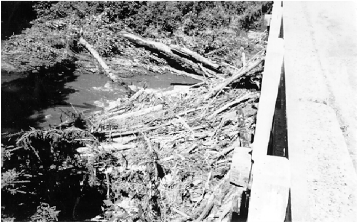
Figure 5.26: Severe Debris Problem at a Bridge Crossing
