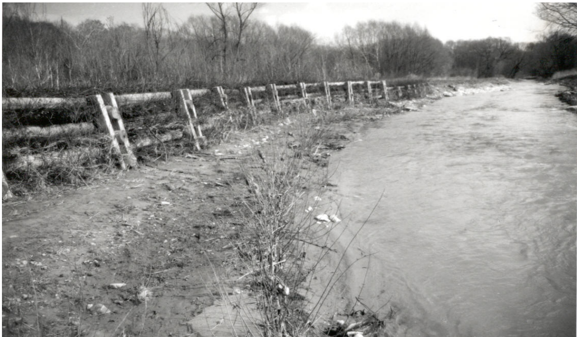
Figure 10.9: Live Cribwall Installation
