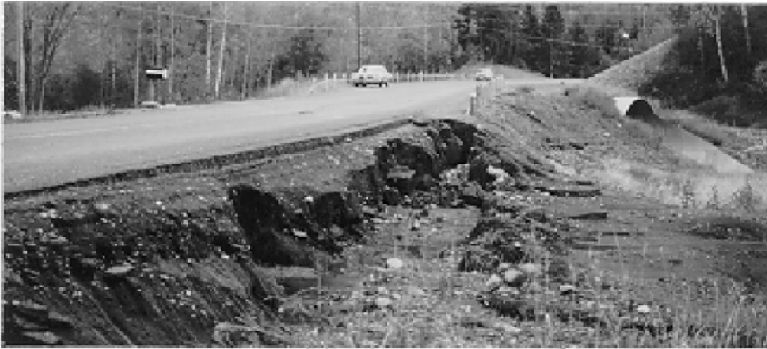
Figure 7.10: Evidence of Relief Flow at a Culvert
