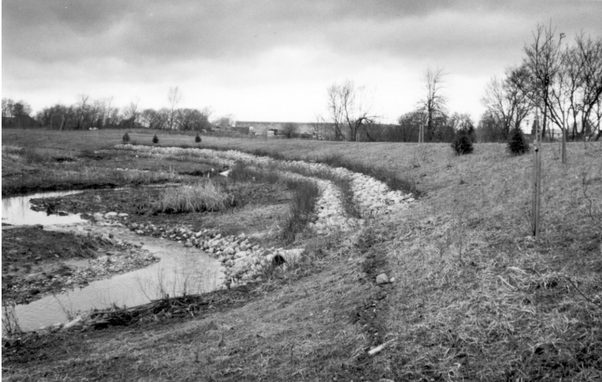
Figure 10.8: Riprap Installation with Brush Layers
