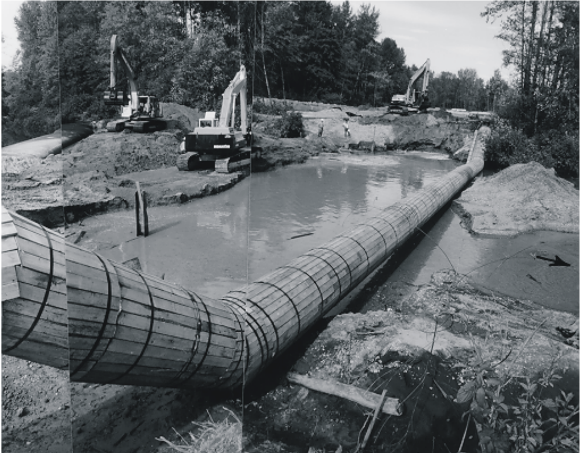
Figure 9.51: Excavation of Trench across a Small Stream for a Sewer Line.
