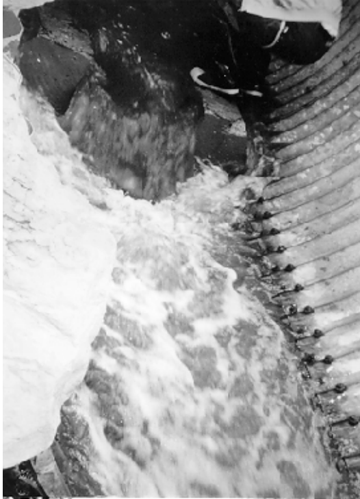
Figure 5.16: Weir Baffles in a Steel Culvert
