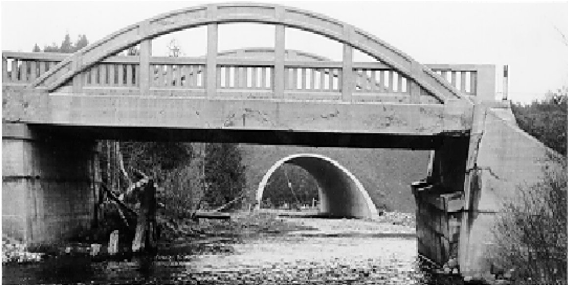
Figure 7.19: Damage in Bridge Abutment due to Scour
