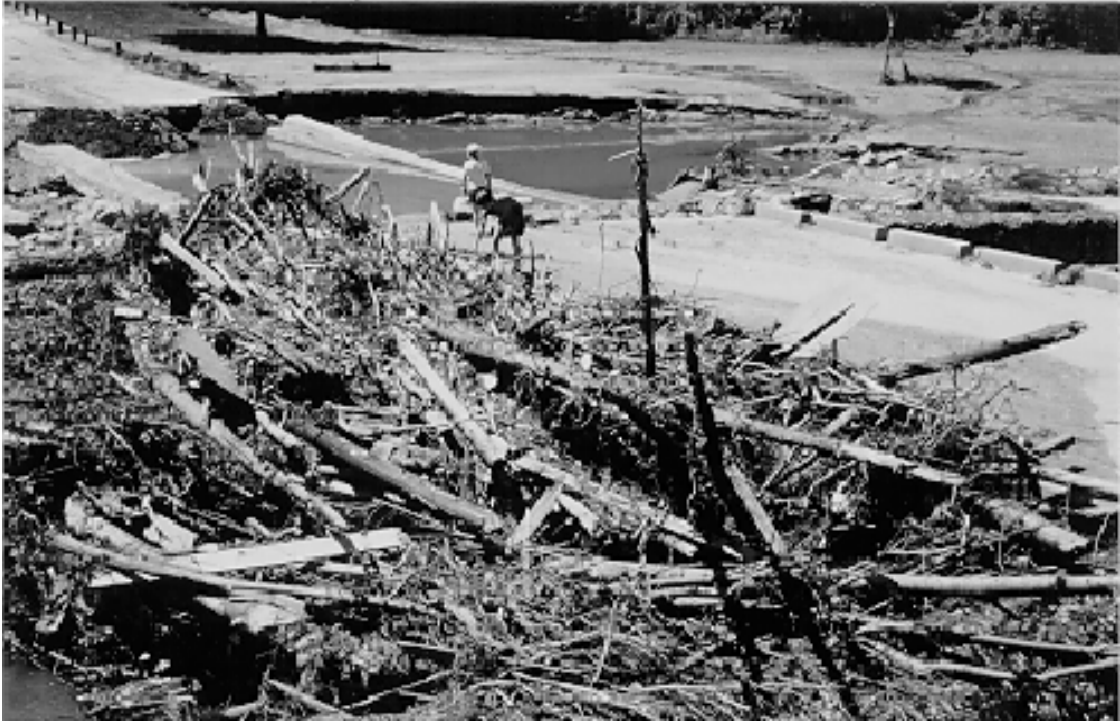
Figure 7.24: Debris Jam at a Multi-span Culvert
