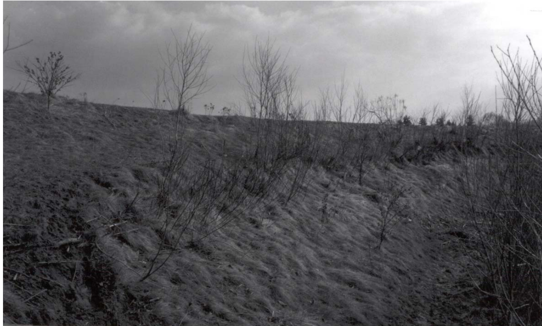
Figure 10.2: Live Fascine on Contour after First Year Growth
