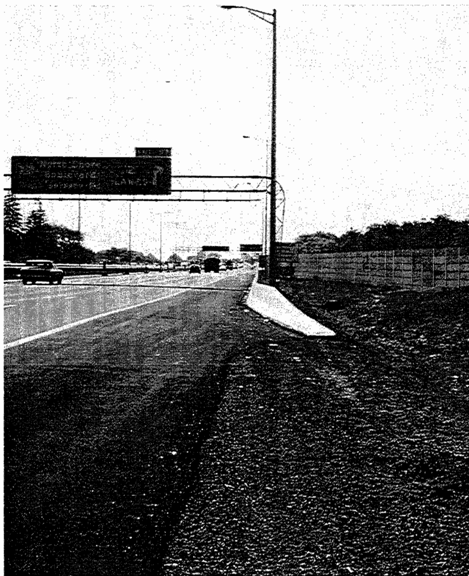
Figure 4.3.12 Tapered End Treatment, Permanent Installation
