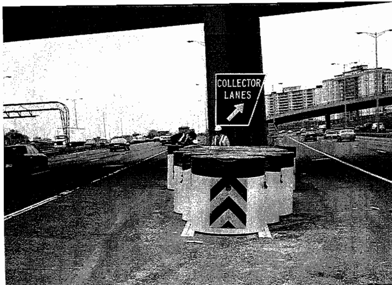
Figure 2.9.2 Gore Area Protected with a CIAS Installation
