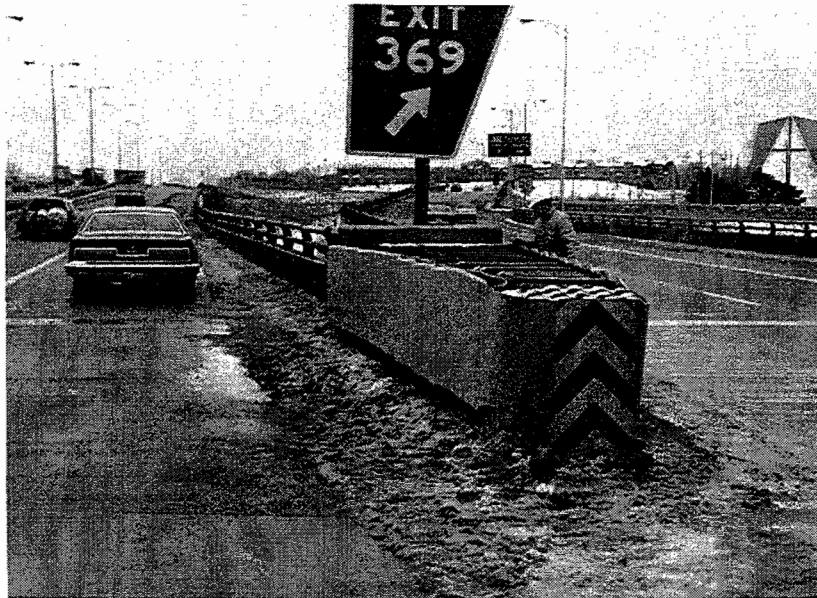
Figure 2.9.1 Gore Area Protected with a HI-DRO System
