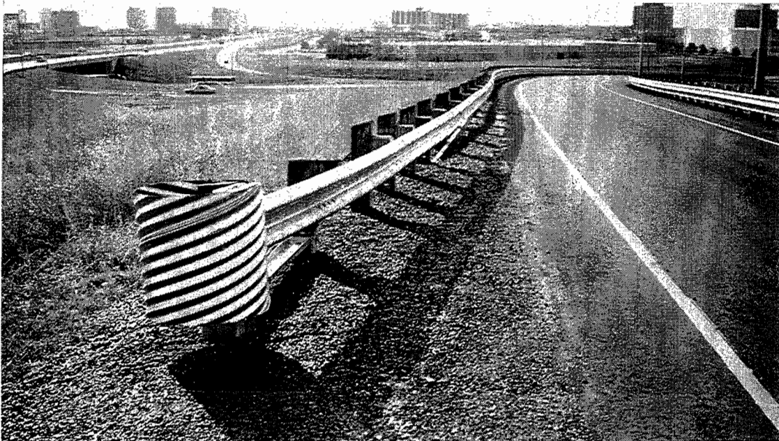
Figure 5.2.8 ECCENTRIC END LOADER Installation
