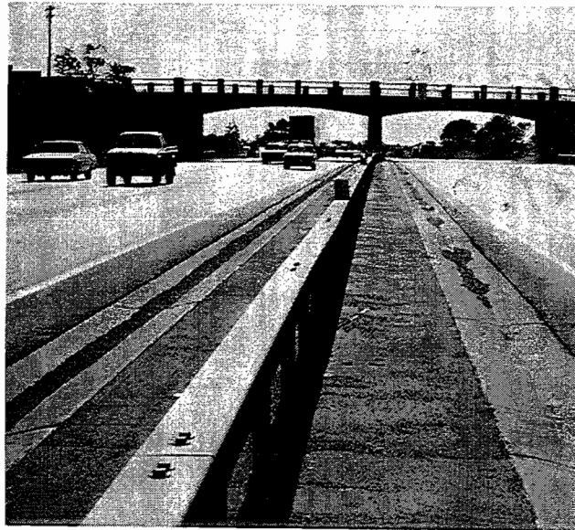
Figure 4.3.4 Box Beam Median Barrier (203.2 x 152.4 mm)
