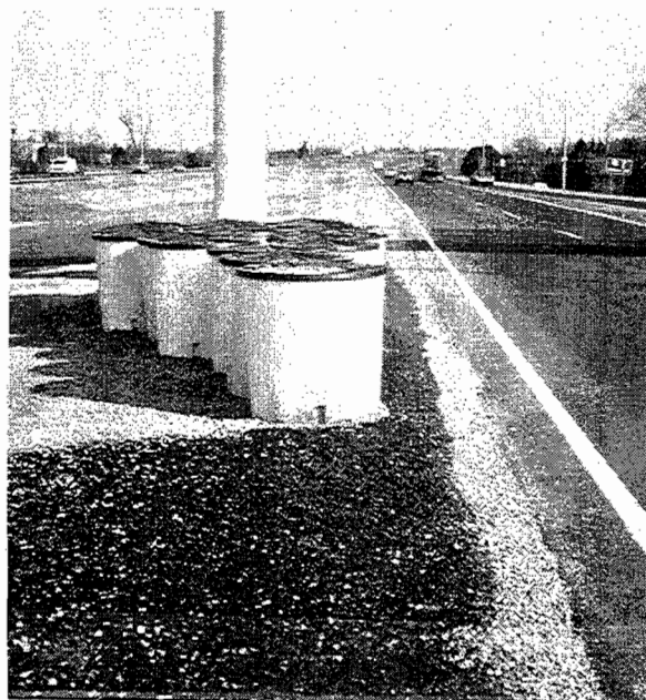
Figure 2.8.8 Pier Protected with Inertial Barrier Modules
