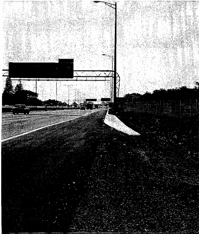
Figure 5.2.4 Concrete Barrier Turned Down and Flared End Treatment
