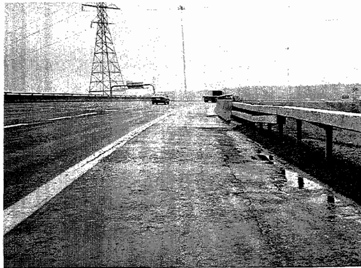
Figure 4.3.5 Double Beam Installation
