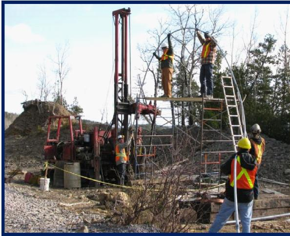
Figure 4. Emplacement of a 52m long vertical string of SAA sensors at site 1 in zone III (note the required curvature radius needed for inserting the string).
