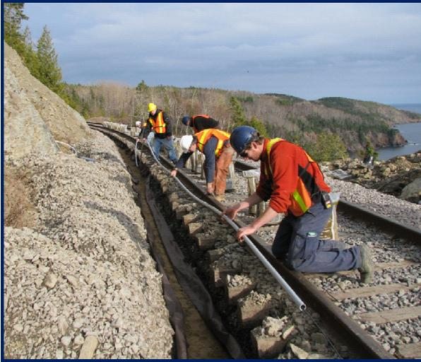
Figure 6. Installation of the 60m horizontal SAA string along the railroad track in zone III.
