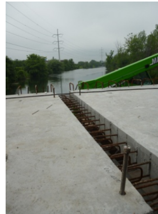
Figure 16. Joint de béton
