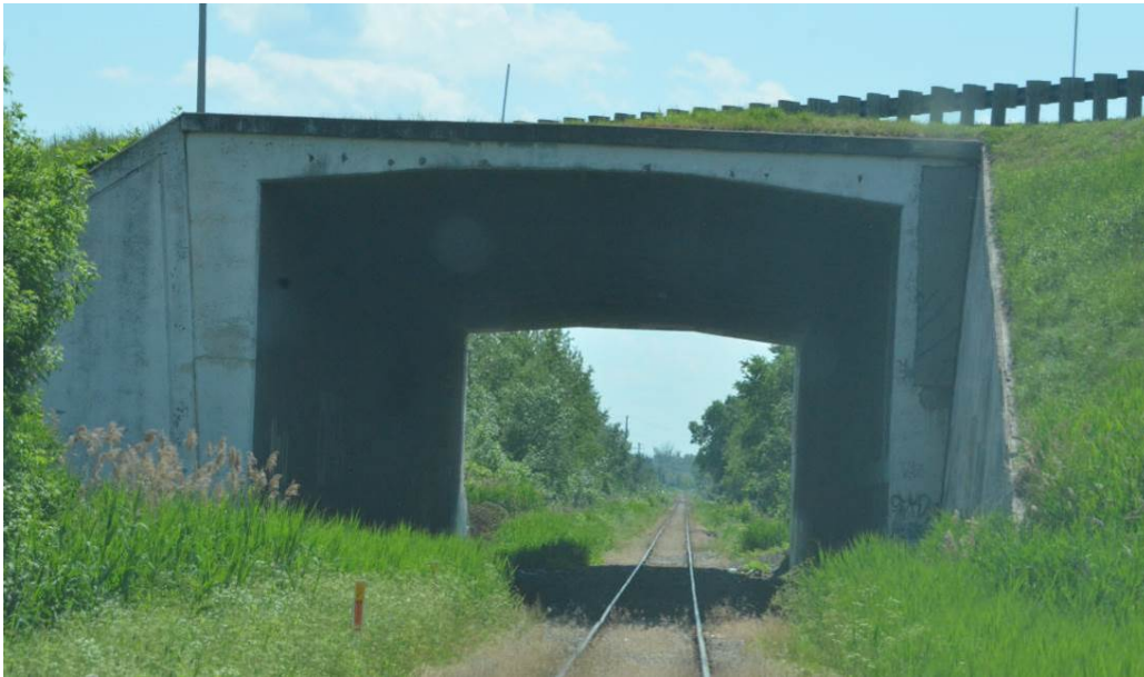
Figure 51 – Pont routier de l'autoroute 15, P.M. 79,40
