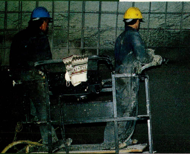
Dry-mix and wet-mix shotcrete is used to repair concrete structures.
