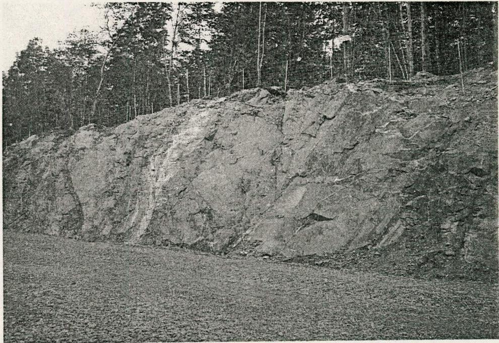
PHOTO 6 INFLUENCE DES CONDITIONS GÉOLOGIQUES: L'ORIENTATION D'UN SYSTÈME DE JOINTS PRATIQUEMENT PARALLÈLE À LA DIRECTION DE LA COUPE A ANNIHILÉ LE PRÉDÉCOUPAGE.
