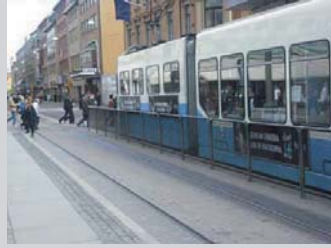
Fencing between the tracks at tram stops
