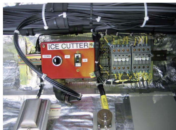
Ice cutter switch (under cove) to avoid operator confusion
