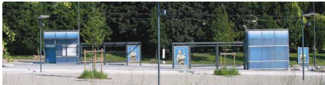
MULHOUSE - STATION DE TRAMWAY ILLBERG
