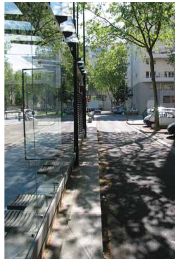
LYON - PROTECTION PARE -VENT DES STATIONS
