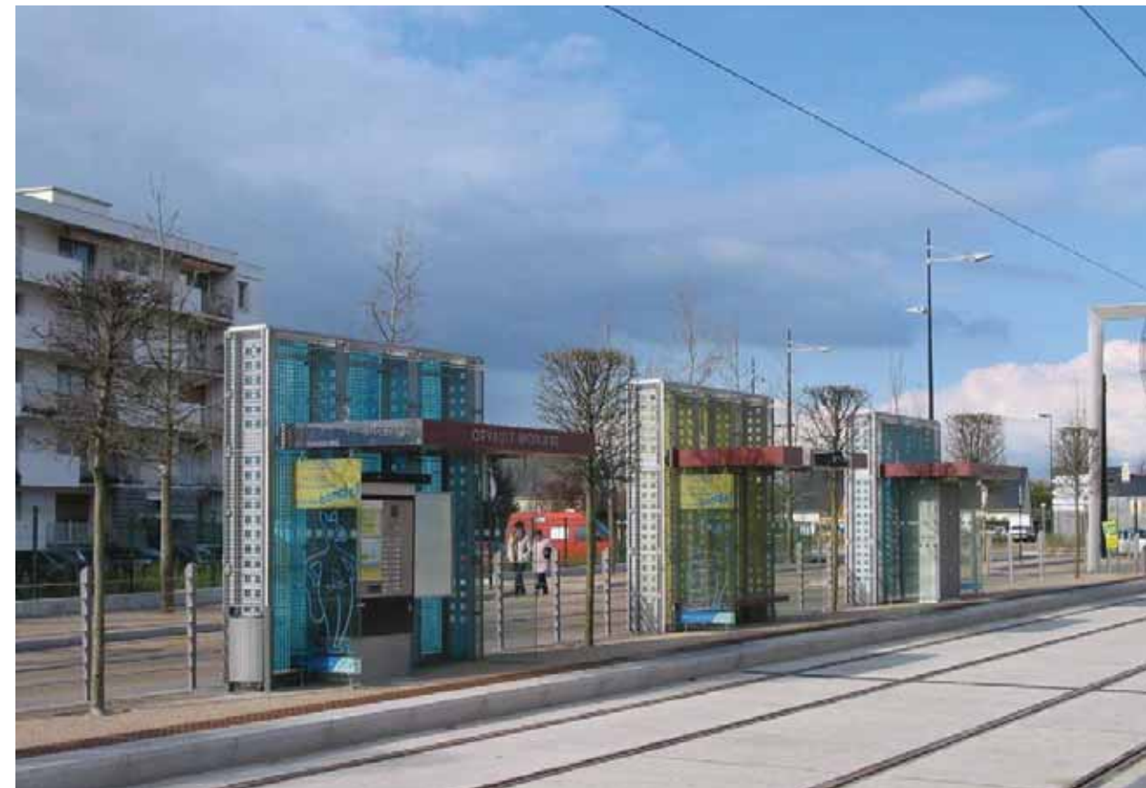
NANTES - STATION ORVAULT - MORLIÈRE
